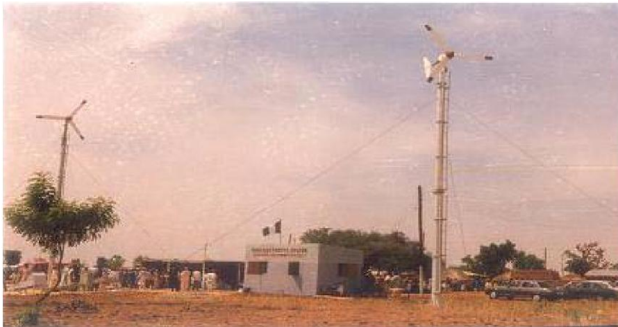
Fig 9. A 5kW aero generator in Sayya Gidan Gada, Sokoto State [39]
