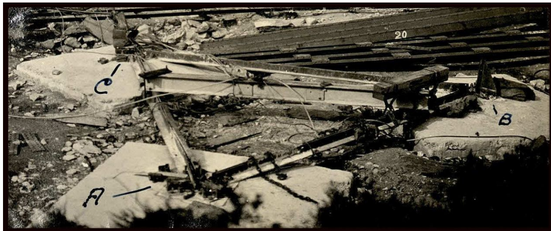
100. Detail of 1923 lattice mast base arrangements from a larger photograph (MS.Photogr.c.243, photo 729/x) following Mast 13's collapse. The hand-drawn labelling is contrary to the foot pad labelling scheme indicated by MS.Photogr.c.243, photo 734/x (see mast identification graphic at p.10, based on information in original caption for 104 ), and is not considered to be the general identification scheme used across the site.
