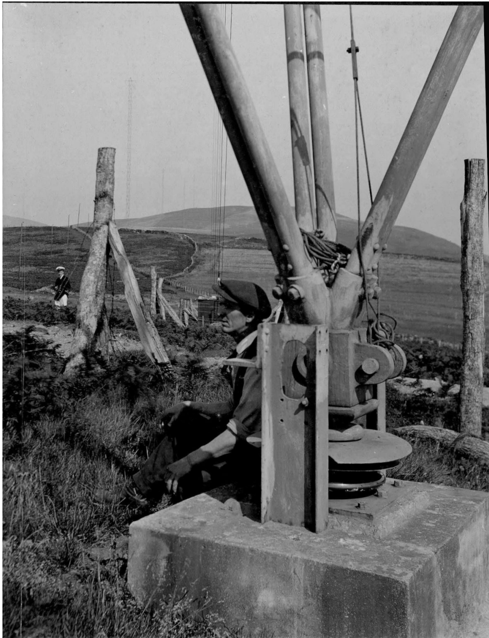
R8. A worker takes a break at the base of a receiving antenna support mast in this contemplative scene. Note the halyard, which is seen to run inside standoff brackets in other images. Four other lattice masts of the original, 'inverted-L' receiving antenna are seen to run up the hill in the distance. The top of the nearest mast seen in its entirety clearly has a horizontal arm. This supported a single wire either side; contemporary accounts describe it as a "two wire" antenna (Bodleian Special Collections, MS.Marconi.198), though electrically, it was one, connected at a common anchor point and then to the receiving sets. A man in naval uniform bearing the sleeve insignia of Lieutenant looks on, centre right, hinting at a WW1-era date. The mast converges on a tilting bearing. The steel uprights, with roughly-cut oval openings either side of the base mount would almost certainly have been a temporary pivot or securing point for erecting the mast at installation. Guy wires kept the mast vertical. The base remains in-situ, but the steelwork is now rapidly dissolving in the salt-laden gales. Bodleian Special Collections, MS.Photogr.c.243, photo P.2097, date unknown, probably ca. 1918. The distinctive curved field boundary, which is unchanged today, permitted the location to be confirmed as 52.581847^{\circ} , -4.066318^{\circ}
