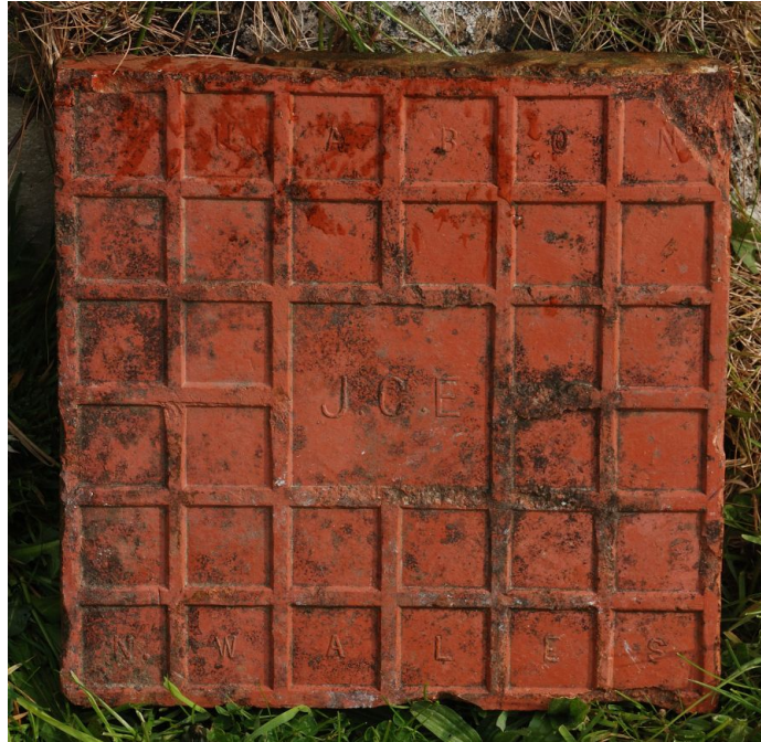
C33. Reverse of transmitter building floor tile, bearing 'Ruabon', 'J.C.E.' and 'N. Wales' impressions, indicating J.C. Edwards (Ruabon) Ltd, active 1903-1956 (Denbighshire Archives, GB 209 DD/DM/27).
