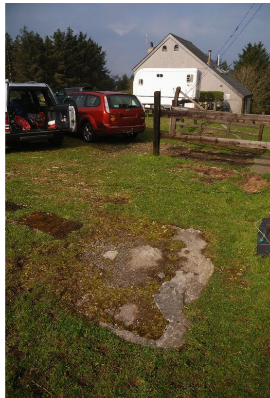
D24, right: concrete base (foreground) with embedded vertical bolts, the base for an earth catenary tubular steel mast support. The power house building, now a domestic dwelling, is seen in the background and, in 2023, was externally clad in timber. Due to such modifications, the power house has failed to meet listing criteria and cannot be protected by law – another tragedy of long-term laxity within the Welsh heritage agencies.
