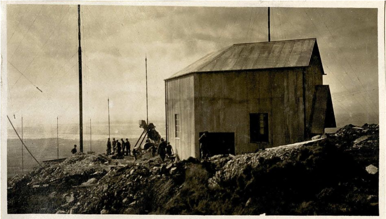
72. A very atmospheric photograph of the double inductor ('ATI') house during construction in early 1923, taken from the east. MS.Photogr.c.243, photo 711/x. The dark line across the building appears to be an old water stain on the image. Note the slack wire running steeply from ground at lower right; this may be evidence the 1921 pylons are still in place. A rod-insulated wire is also seen and may have been for tensioning, acting forwards, but removed from its pole.
