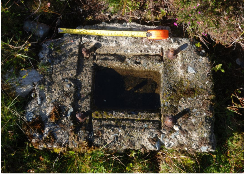
127. Deeply-socketed, small concrete base with four bolts. This lies at the top northern edge of the 1923 extension inclined trackway leading to the lower reaches of the site. It was not deeply-set in the ground and is quite loose now. It may have been a points or other trackway-related feature. Bolts separated by 14" x 9". Socket aperture = 9½" x 6¾" at top, 8½" x 4 ½" at bottom; 3" deep.
