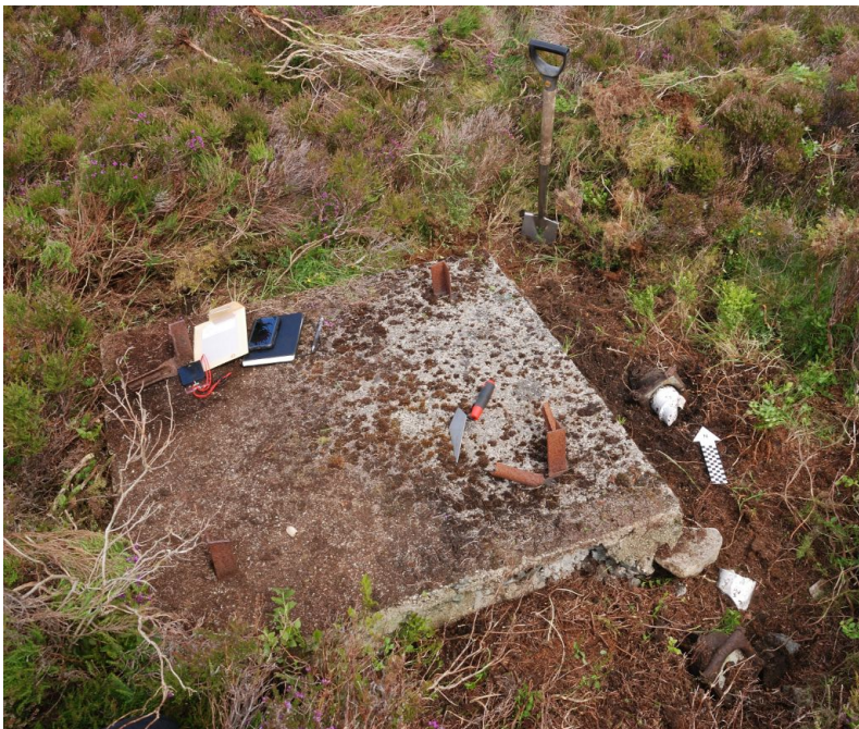
49. A counterpoise base (concrete of 4' x 4') for the 1923 extension/upper array, showing remnant lattice ironwork (32" x 32") and two large tubular insulator fixings, now known from detail visible in MS. Photogr.c.243 image 718 (inset, right) to be used to strain the wires at the tower; a 'jumper' wire interconnected both sides of the counterpoise wire over the tower. Concrete = 4' x 4'. 53.121962°, -4.169796°
