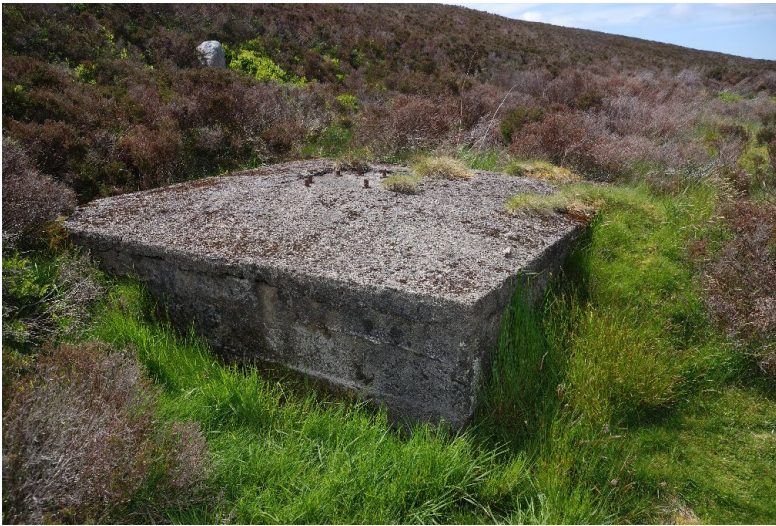
99. Profile of a 1923 lattice mast base block (one of three per 3-sided mast). As is the case for most of the concrete structures, the raised top surface, for drainage away from the metalwork, was evidently laid separately to the main block, and appears to be fairly weak in comparison. The studs, however, ran deep into the main block. Note horizontal shuttering impressions. Mast 14, footpad C, 53.123037°, -4.169589°. Inset, top: 1915 installation of mast plate at Abu Sueir, Egypt, prior to "grouting and plastering", clearly a generic and widely used Marconi site construction method, shown completed at inset, lower (MS.Marconi.219).
