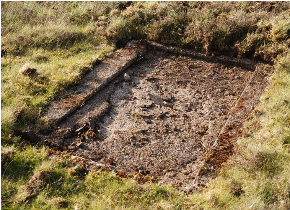
125. Entirely grassed-over when discovered, surface clearing revealed a large concrete base with corner bolts, iron spacers and two trackway rails protruding, leaning slightly towards the south-west. Thought to be a trackway winder base serving a trackway running downhill to the west, to a quarrying area behind the 1914 upper masts. Located immediately to the NE of 1921 extension, northern Pylon A. 53.123001°, -4.171694°.
