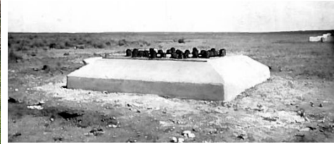
99. Profile of a 1923 lattice mast base block (one of three per 3-sided mast). As is the case for most of the concrete structures, the raised top surface, for drainage away from the metalwork, was evidently laid separately to the main block, and appears to be fairly weak in comparison. The studs, however, ran deep into the main block. Note horizontal shuttering impressions. Mast 14, footpad C, 53.123037°, -4.169589°. Inset, top: 1915 installation of mast plate at Abu Sueir, Egypt, prior to "grouting and plastering", clearly a generic and widely used Marconi site construction method, shown completed at inset, lower (MS.Marconi.219).
