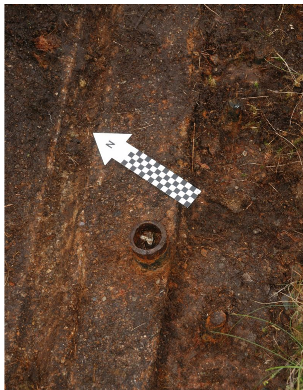
84. After a couple of days' drying, the much brighter concrete (and distortion of the outer edge of the internal drainage channel) clearly confirms the original 1923 double ATI concrete base was cut into (ca. 1925) in order to install a new feedline. Steel tubes, externally threaded, OD = 2¼", lead cable sheath diameter ca. 30mm. An additional wire (lead cable sheath diameter ca. 15mm), possibly the connection to the GLC (lower) earth screen, to the east of the porch, in the MUU (upper)-facing part of the ATI house ( 85 , below), seems to have been in place from 1925. Tube (unthreaded exterior) for this cable is OD of 2½", ¼" wall thickness. The hole for the cable to emerge from the base was found, but no trace of the cable remains.
