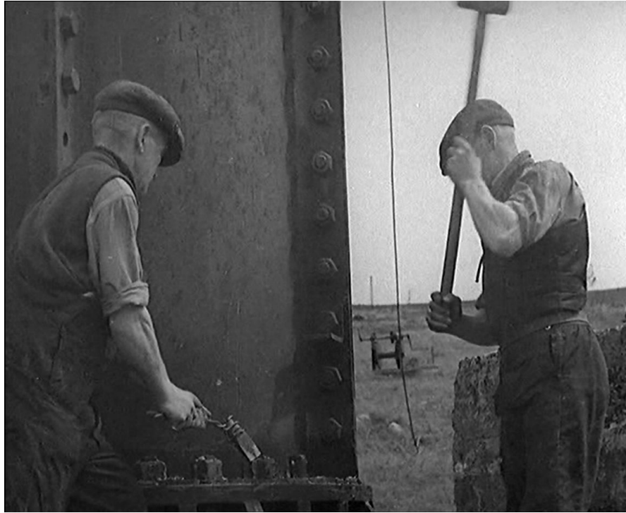
21. Hand-operated, empty, possibly triatic winch uphill of a mast, almost certainly Mast 1, given the concrete anchor to the immediate right of the hammer-wielding gentleman, during demolition in 1939. The scene shows the men splitting mast base flange to tube-securing nuts with a sharp chisel mounted on a thick twisted-wire handle to eliminate impact shock to the user's hand. This usefully explains the numerous split nuts still to be found across the site. Source: © Reuters via British Pathé, Film ID: 1013.05, issue date: 1/06/1939, under licence.
