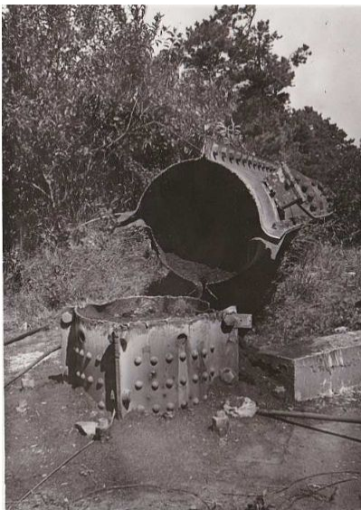
129. Felled four-section mast, usefully showing the fairly thin steel used for such supports, at Chatham, MA, USA. 1954. © Chatham Marconi Maritime Center, via Ed Moxon.
