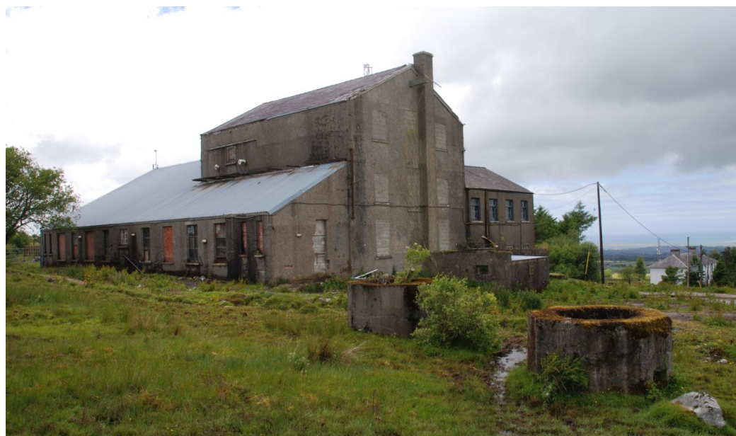
114. Octagonal inductor bases to the north of the transmitter house (on domestic land, access by kind consent of the occupiers). The nearest base, far right, is seen in a poor photo to support an inductor (see 116), and thus predates the 1925, GLJ 'third' antenna.
