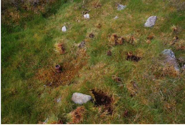
107. Ca.1921 extension pylon 'A', footpad 'C'. 53.122060°, -4.174204°
