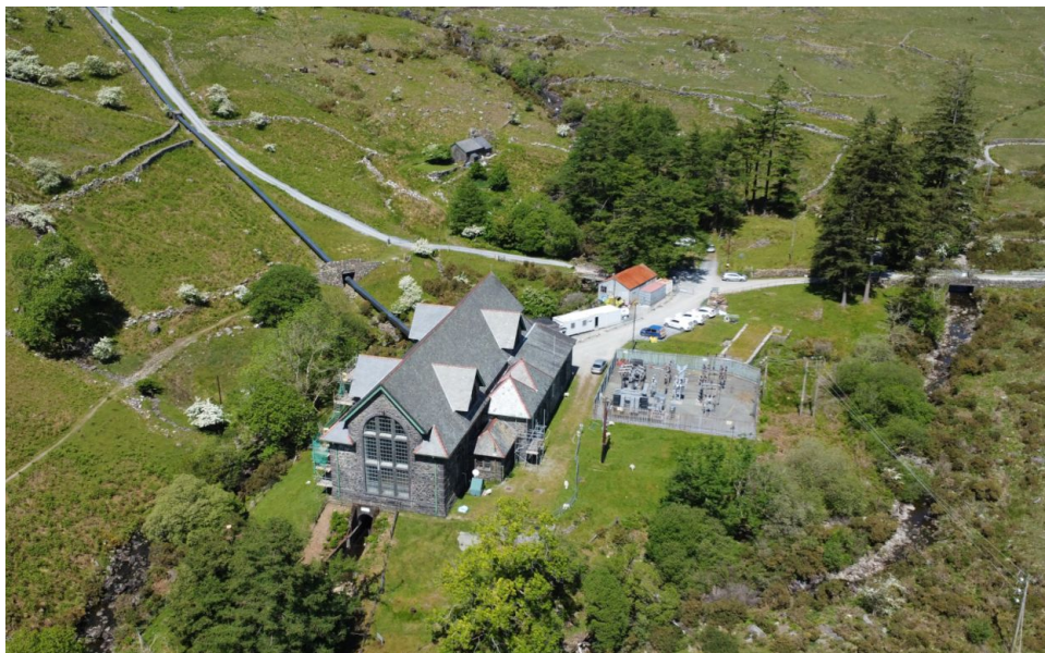
T15. Cwm Dyli hydro plant, built 1906. Image of summer 2023.
