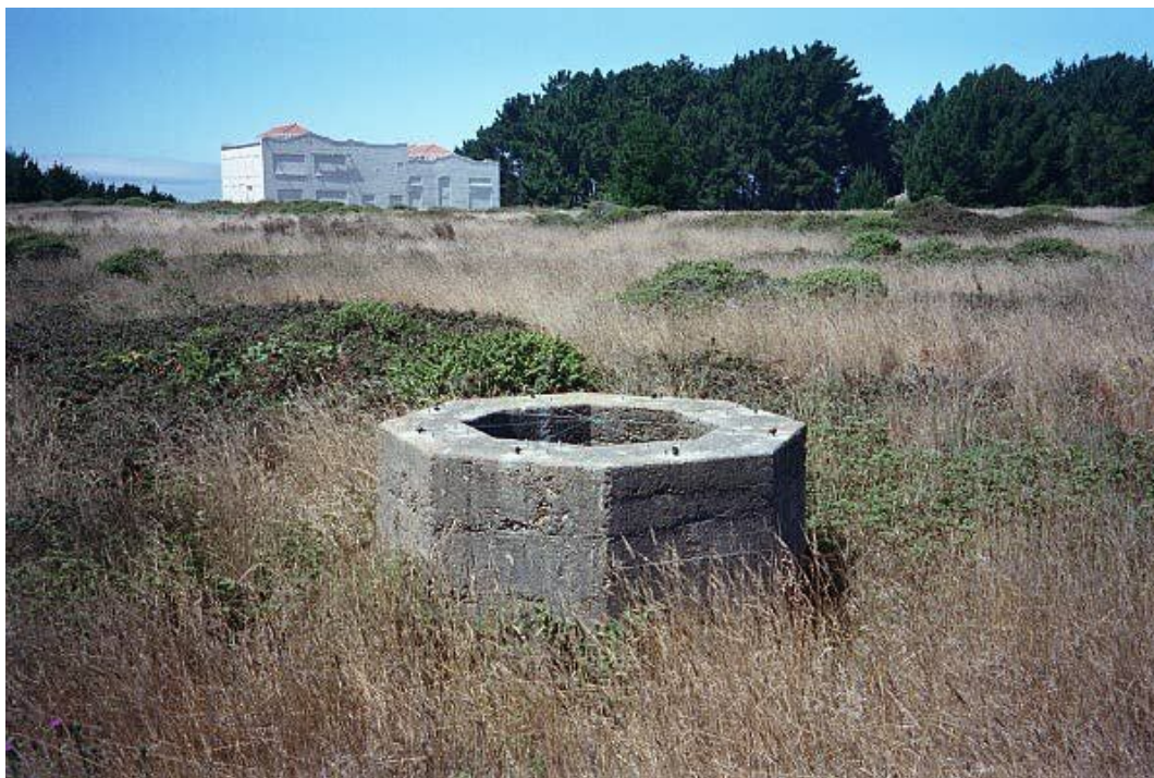
113. Octagonal inductor base with no side openings at Bolinas, CA, USA. Image courtesy California Historical Radio Society.
