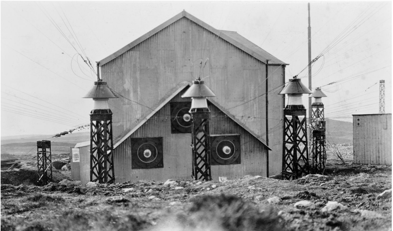
73. Double ATI from the north-east (MS. Photogr. c.24, 745/x). The three lattice supports in the foreground were set on concrete bases on an elevated, rocky platform between the foreground and end of the building. The central base was sought and confirmed during fieldwork (see 75). Bodleian Special Collections.
