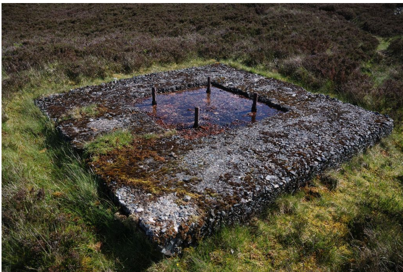
106. One of four ~8 ½' concrete base feet for one of two ca.1921 extension pylons (53.120347°, -4.175167°), each pylon centre separated by 600'. Each of the four footplates of each pylon was separated by 60'. At the lower (southerly) mast, the NE corner base had to be installed on what was apparently boggy or otherwise difficult ground, with bolts emerging from a concrete base in a deep excavation to reach firmer ground – see 107.
