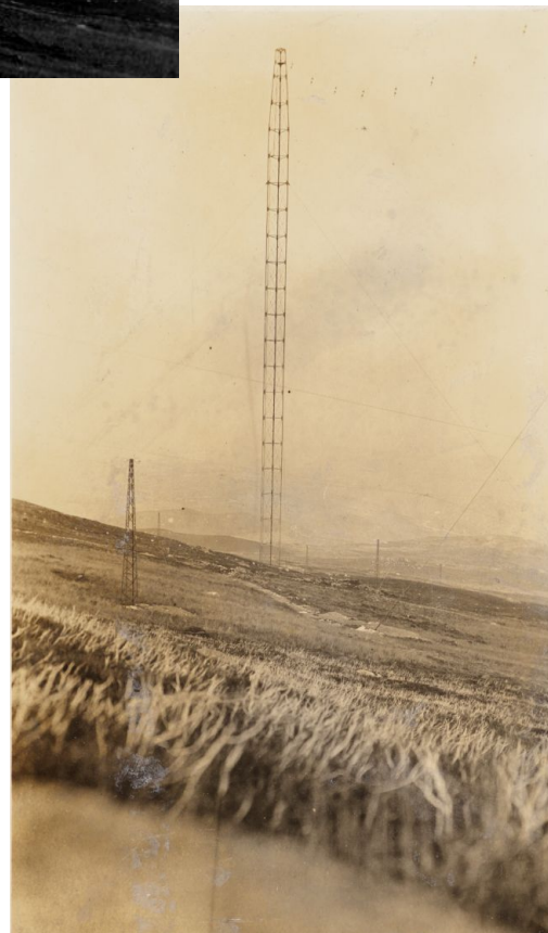
70a (above) Photographed shortly after completion in 1924, the extension array radiating wires, hung from a triatic seen running between Mast 15 and the out-of-shot Mast 16, can be confidently traced out by careful contrast enhancement. Some of the elevated counterpoise wires (dotted green lines) are also evident, as are what may be tensioning wires (solid green) running from lower centre to lower right. The steeply-sloping wires to the rear, Llanberis end of the array, which terminated at the lower ATI house, are clearly revealed. The original image, MS.photogr.c.243, photo 718/x, is seen at 70b , right. 70c , radiating wire suspension schematic, at upper left.
