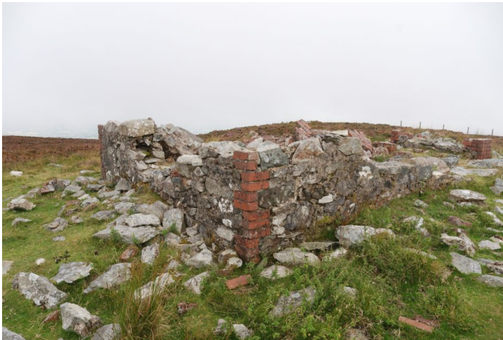
Left: blockhouse 6, eastern elevation to left, northern to right.
