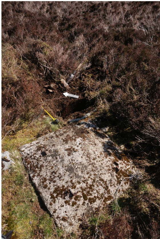
D12 , left: 1923 support mast concrete base, with location of copper wire attached to surrounding galvanized steel plate, below scale arrow. The mast was offset from the pattern of counterpoise supports, and there are two other known examples. Their purpose is not yet known.
