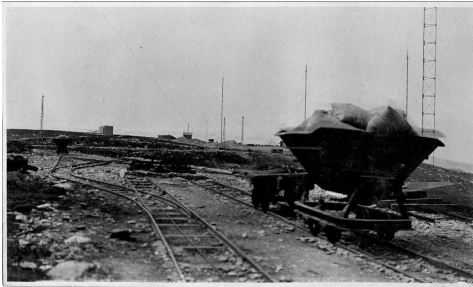
General view at top of Incline showing level run to main dumps arrangement of brake pulleys and cross over.
