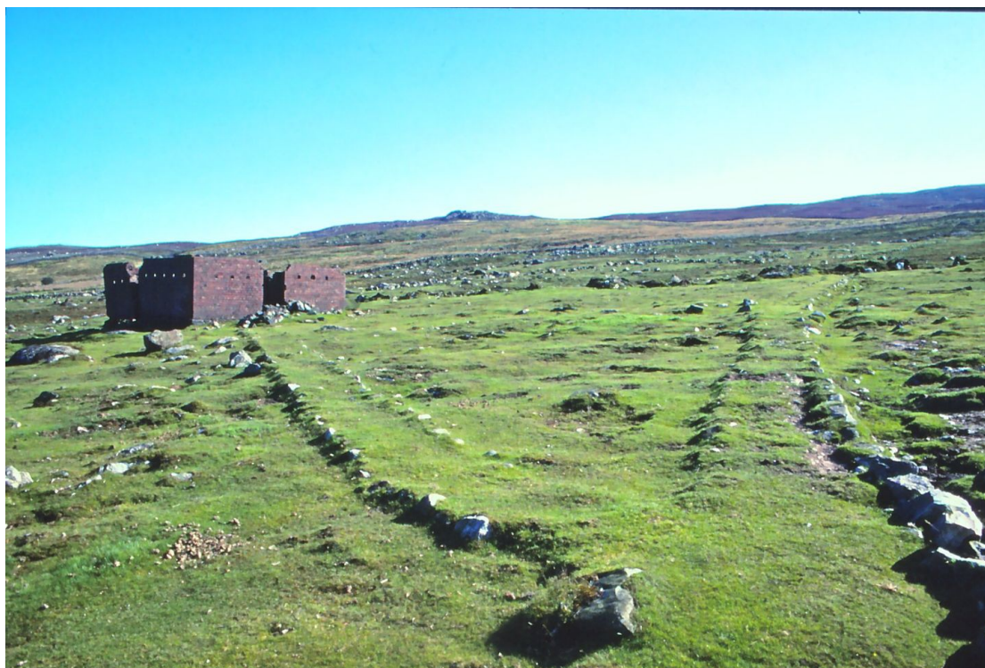
143. Blockhouse 2, photographed in 1988, when the raised stonework trackbeds built to transport materials were clear of plant growth. The track going uphill to the right continues to blockhouses 3, 4, 5 and 6. By 2022, undergrowth has rendered invisible that which was, 34 years earlier, very clear. Image: Plate 6 in Gwynedd Archaeological Trust's Report 1302, March 2016, p.88. By kind permission of and © GAT.
