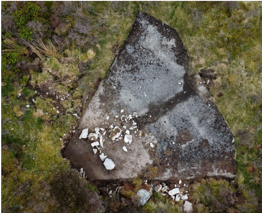
D18 , left: aerial view of upper double anchor base for mast 11C (to upper left), 12B (to lower centre right). Dimensions as given in D14.
