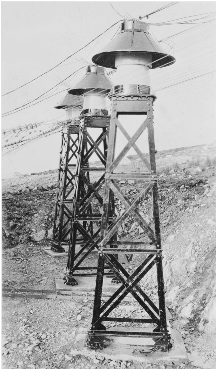
76. Straining towers of the upper (double) ATI, serving the 1923 extension. Bodleian Special Collections, MS. Photogr. c.243, photo 748/x. Lattice base measurements (nearest facing length in photo of 1156mm or 3'9 1/2") permitted scaling and a determination of an exact, 12' height for the steel lattice. Wires to the hat are the antenna feed, the catenary of wires below being the counterpoise connections. The towers are seen to be grounded via copper straps at their furthest left-hand corner in each case. The mounted insulator and rain hat added about 3'6" to the height. The ceramic fragments at C40 are consistent with the insulators mounted on the frame. Dated January 1924.
