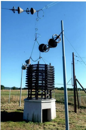
108a , left. Octagonal inductor at VLF station, SAQ, Sweden, serving to match the antenna radiator wires seen leading down from the support towers at centre right. Image courtesy Eric P. Dollard. Also see rear cover for an image of one of Carnarvon's inductors.
