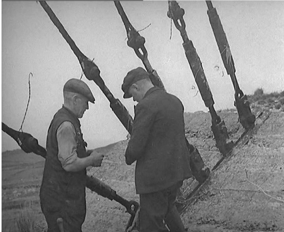
6. Preparations for stay cutting with explosives (method confirmed in Aberdeen Evening Express , 24 th May, 1939, p.5 and Liverpool Daily Post of the same date, p.13), during May 1939. Five stay attachments are seen. Other photographs show seven stay wires. This is explained by two wires being attached, via a trapezoid plate, to each of the lower two anchor attachment rings (plate just visible lower centre). In this image, and in another of the tower immediately before felling, some of the lower stays have already been detached. The projecting thin wires appear to be copper grounding wires (cut) between stays. Image © Reuters via British Pathé, still N°. 7, Film ID: 1013.05, issue date: 1/06/1939, under licence.
