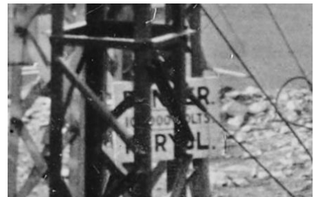
73a. Detail from 73 of hatted strainer mast at right rear, showing a bilingual 'Danger' and (Welsh) 'Perygl' warning of what appears to be 10,000 volts (MS. Marconi 790, item 5, details valve tests, almost all with the anodes ('plates') at 10,000 V, in April 1926).
