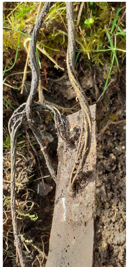
Excavated grounding strap (right) for the stay cable of Mast 13/17 at anchor block 13/17A, with two bonded, 7-strand copper wires running into the earth. The wires and band were covered with ballast-type stone. Scale squares = 1cm ( not arranged to show north).
