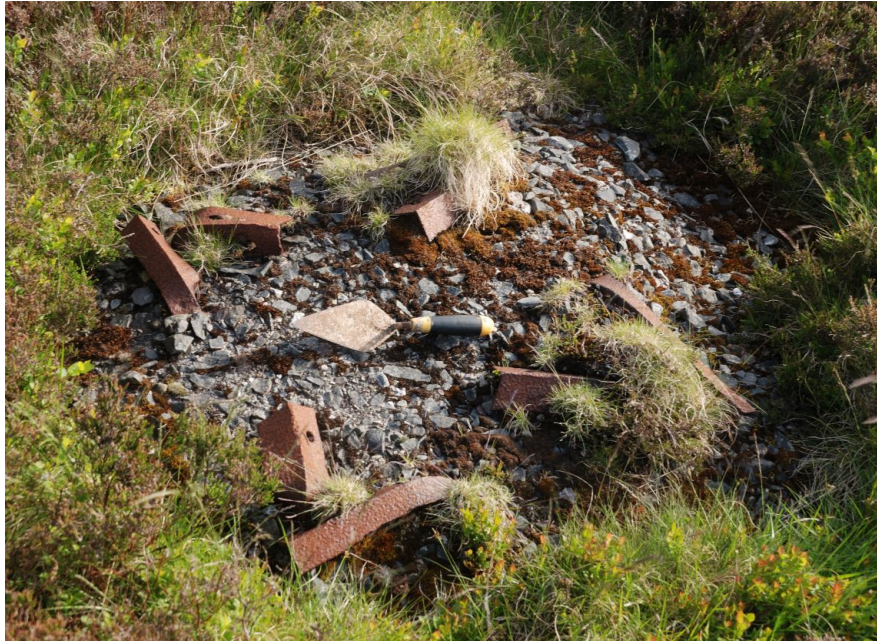
48. A typical concrete base for an elevated counterpoise lattice mast of the lower, N°1 antenna array after ca. 1921, with remains of the mast legs (1¾" x 1¾" L-section steel). Many of the bases can only now be found when the pattern of installation is worked out from those few that are more readily found, and the pattern of shallow trenches for ground wires that are still seen to run between them. The bases in many parts of the lower end of the lower antenna are now fully buried by deep bog growth, whilst the bases for the 1923 extension are typically overgrown by dense, tall heather and, at the lower end, by bog growth. Trowel blade = 6"/15cm, bases typically 35" x 35", lattice sides 20½" x 20½".
