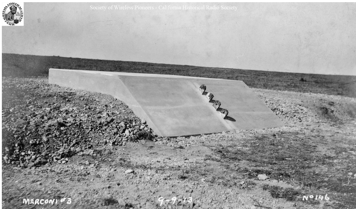
11. The global span of Marconi's wireless system becomes clear as we find an anchor block of the same form in Bolinas (initially callsigned 'KET'), California, USA, at 5,168 miles from Carnarvon. All US Marconi stations were soon taken over by RCA due to government concerns over control of communications. Date as per photo annotation. Image courtesy California Historical Radio Society, which, in 2017, revived the later callsign 'KPH' as a WSPR beacon receiving station on the amateur radio HF bands.
