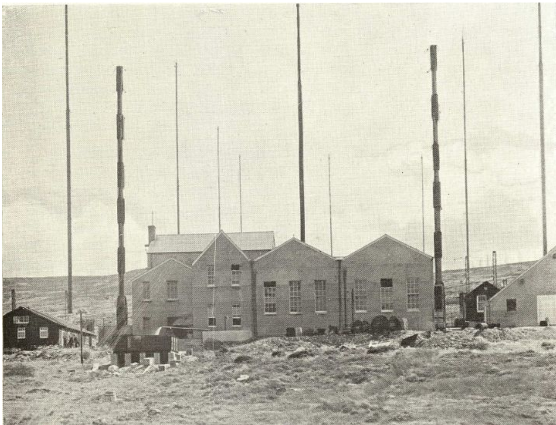
56. Looking uphill (east). The elevated ground screen is in place, as are the two shorter steel towers, which an account written for Engineering journal (Bodleian Special Collections, MS.Marconi.198) indicates is the forward radiator wire straining system that was a later addition and not part of the original, 1914 antenna. The wires are recounted as meeting at a common anchor, still present, to the west of the buildings – seen here converging towards the ground, at far lower left foreground. The ~500' extension masts to the rear are not seen. Date unstated. From the content of the pamphlet in relation to “recent removal” of timed spark transmitters (October 1921), the existence of Alexanderson alternators (from early 1921) and valves (1921), the absence of rear pylons (ca. 1921, uncertain) or the 1923 extension masts, the date of the photo is likely to be around mid-1921, the pamphlet itself somewhat later, perhaps very late 1921 or early 1922. The rear extension of ~500' must therefore have happened around mid-late 1921, as they were already removed by early-mid 1923.
