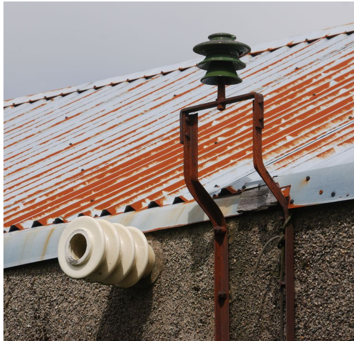
C38. At the southern end of the transmitter buildings, a large through-wall white insulator, of the same kind still seen at the eastern, antenna-facing elevation and at both, now demolished ATI buildings, remains in perfect condition. It may have been the connection to a later common earth point to the rear of the building. Alongside, a multi-part green 'pin' insulator, of currently uncertain purpose. A brown multi-part insulator also remains in perfect condition, mounted slightly to the east on the same wall (C39, below).
