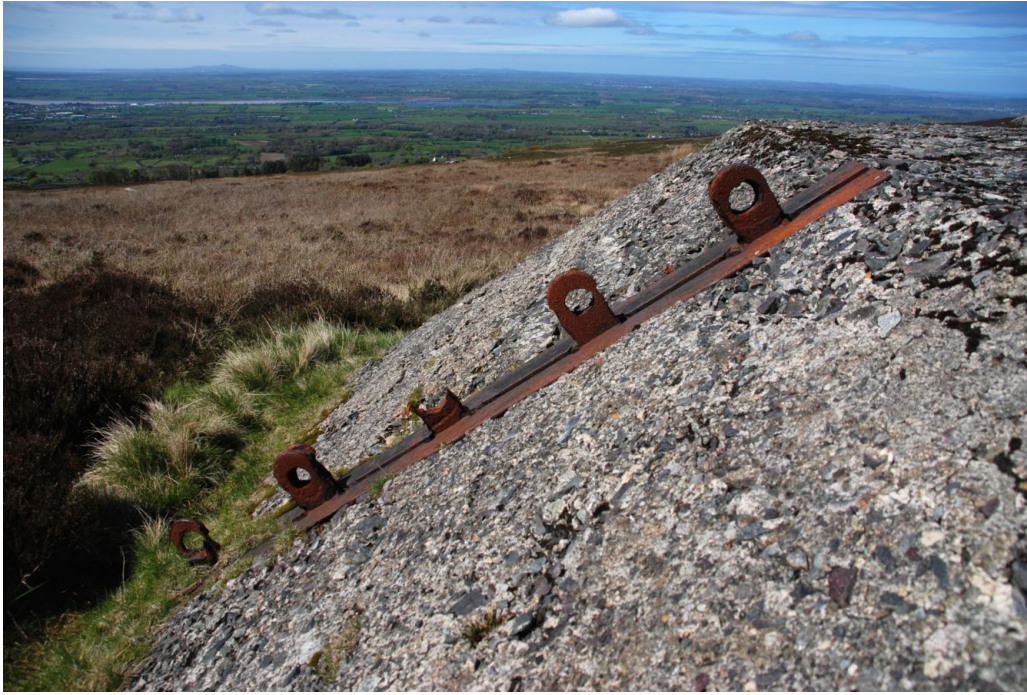
8. Anchor block (6C) and stay turnbuckle attachment points, April 2017.
