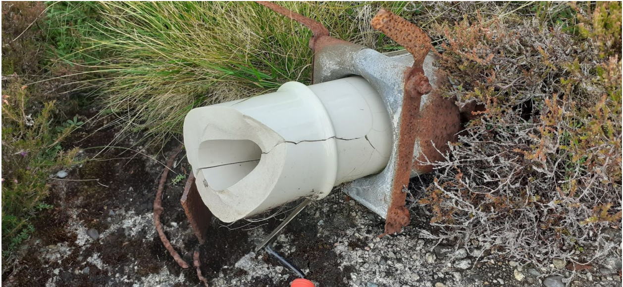
50. Detail of a 1923 counterpoise system insulator fixing (galvanised iron and ceramic). 53.122355°, -4.171794°
