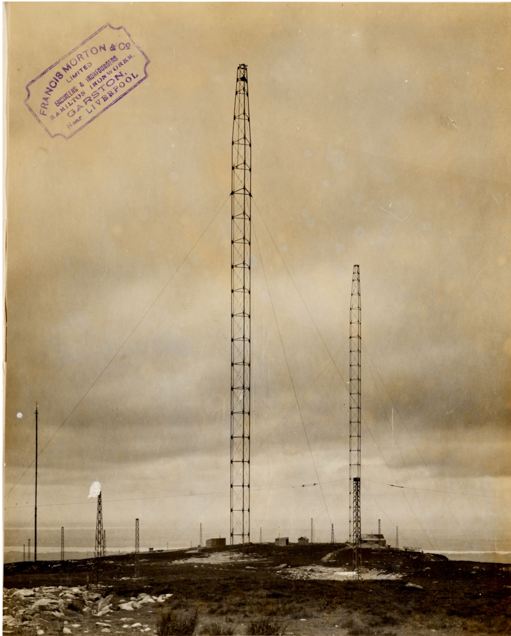
65. An extremely informative, chance-find photograph of Carnarvon's extension to the NE from June 1923 (MS. Photogr. c. 244, a file dealing with Ongar and Brentwood stations, Essex), which appears to be correct dating and labelled photo 737/x. Mast 11 lies, without triatic and antenna wire as yet, in the background, behind blockhouse 5 which has a mixed stone/brick extension to the original, entirely-brick building, for use during the antenna extension's construction (see Appendix IV); blockhouse 6, out of shot to the rear of this photograph, is seen in photo 705/x of the same folder to already be missing its roof and semi-derelict by 1923, only 9 years after the armistice. Mast 12 lies at centre. Various small lattices, mostly or all for elevated counterpoise ('earth screen') support feature prominently, as does the upper, northernmost tube mast of the 1914 antenna, lower far left. What may be wire strainer poles are just visible above the horizon of the summit, lower left, though they were redundant by this time. The ca. 1921 extension, northern Pylon A, would dominate the view between the 1914 mast and Mast 12, but has clearly been removed by this point; one of its concrete base feet is visible when the image is viewed at original scale.
