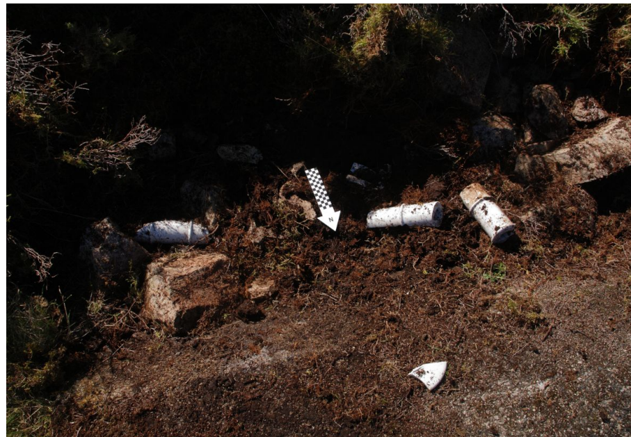
D16, right: tubular insulators once making the link between anchor block and guy wire via metal retaining fixings – see 50. Located at base of southern, mast 12 -facing, sloping edge of 1923 upper double guy anchor.
