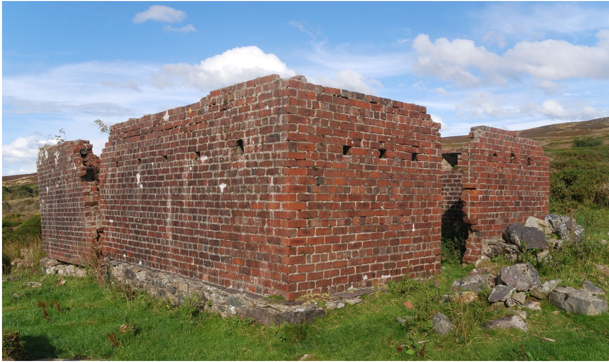
H7. Blockhouse 2, showing stone base as for all site blockhouses, and that all firing holes remain open and were never blocked. It seems not to have had any use after the end of WW1, adding to the evidence that blockhouse 5's firing holes were blocked simply because of repurposing for the 1923 antenna extension. Most or all of the blockhouses had an open porch in front of the doorway.
