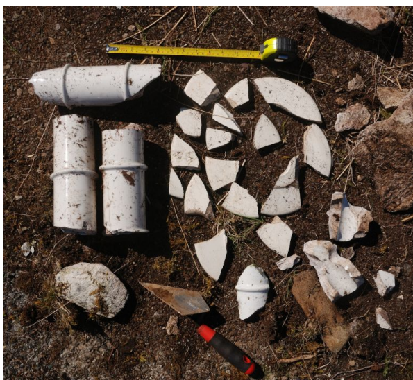
D17, left: tubular anchor wire insulators and disc 'reel' insulator remains. None bear a maker's mark. Tape open to 1ft, trowel blade = 6". 1923 upper double guy anchor.
