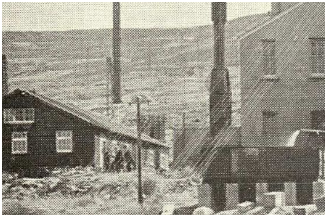
116. Detail from a larger, poor quality image that nevertheless distinctly shows (centre, just behind and to right of the telegraph-type pole), one of seemingly two earth system tuning inductors per side of the transmitter hall at the position of the octagonal base in foreground in 114 . Bodleian Special Collections MS.Marconi.198. See also rear cover image, discovered in 2024, for much better detail of the opposite side inductor.
