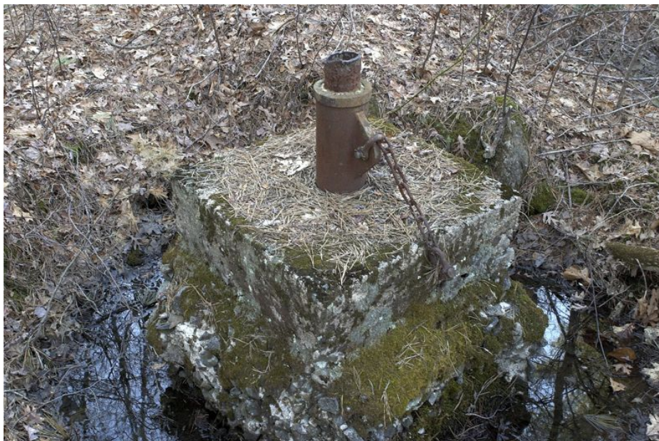
33. Wire strainer base at Marion, MA. Image by kind permission and © of Marian Howell via Sippican Lands Trust.
