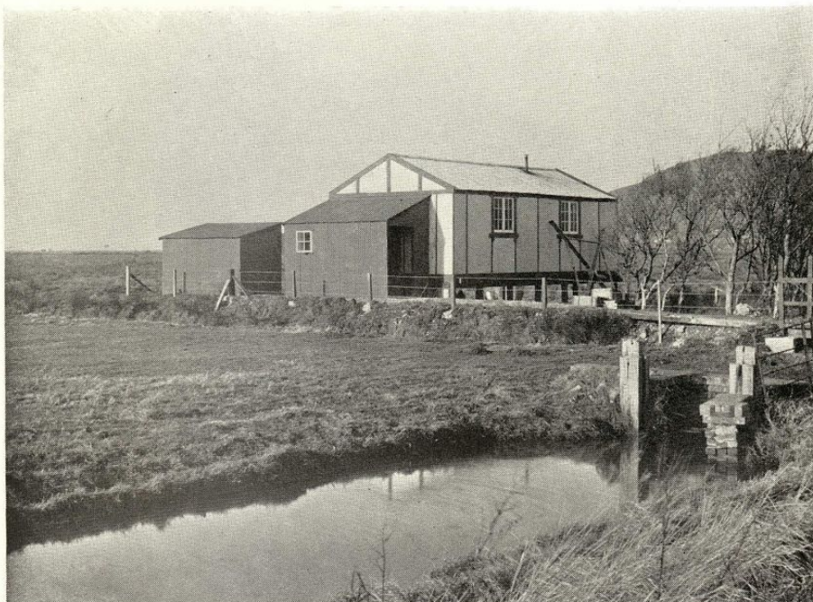
R3. Auxiliary station, centrally housing various control circuits for the later antennas. Ca. 1922 Marconi C°. pamphlet about Towyn, in MS. Marconi 198. Note the channel and high water level on ground only ~2m above OD sea level. A nearby embankment broke, flooding the Marconi station to a depth of three feet, causing “wireless men on boats” on 23/9/1922 – see
