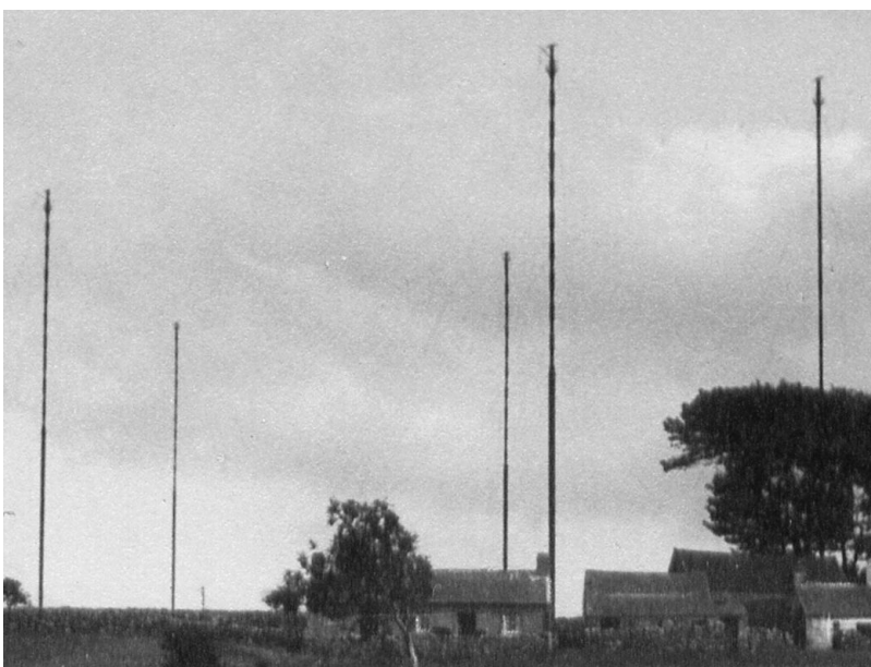
90 a. Circa 1925 image from the Hayward collection, showing masts 1 and 4 (two leftmost, northern) with arms extending to the north. These do not appear in earlier images of this array and it may be the arms were standoffs for hanging the GLJ antenna, which is known from Woodward's drawings to have been located to the north and for which no evidence of mast bases can be found. Original taken by R.N. Barrington, then Engineer-in-Chief at Carnarvon.
