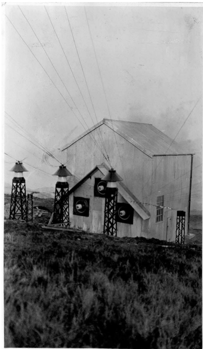
79. The lower, single ATI house for the 1923 antenna array, seen from the south. Internal dimensions 22' x 22', externally measuring, at corrugated sheets, 23½' x 23 ½'. Bodleian Special Archives MS. Photogr.c.243, photo 744/x. As for the double ATI, the feed to the radiating elements are from the three 'hatted' towers, the counterpoise wires from a single catenary strung between the two towers to the sides of the inductor house.
