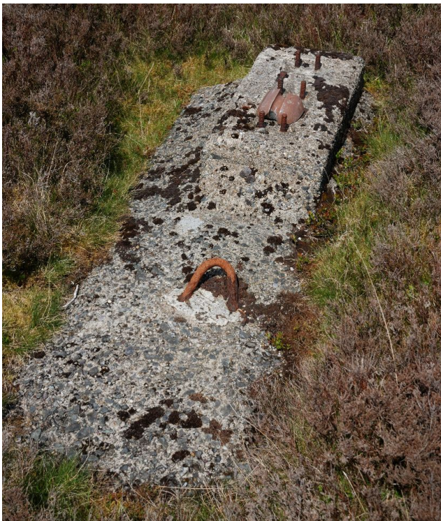
22. Winch base and wire-guiding loop (erosion of the underside of the loop apex is evident by touch). The lighter fine concrete at the base of the loop, evident at all winder sites, suggests it was added at a later point to the base. Protruding block 25½" x 7½" (with variations); bolt centres 10" and 11"; bolts ¾" dia, protruding 2½". Lower base typically 85¼" x 37". Lower and upper base apparently cast as one unit. A broken brown stay insulator rests to the rear.
