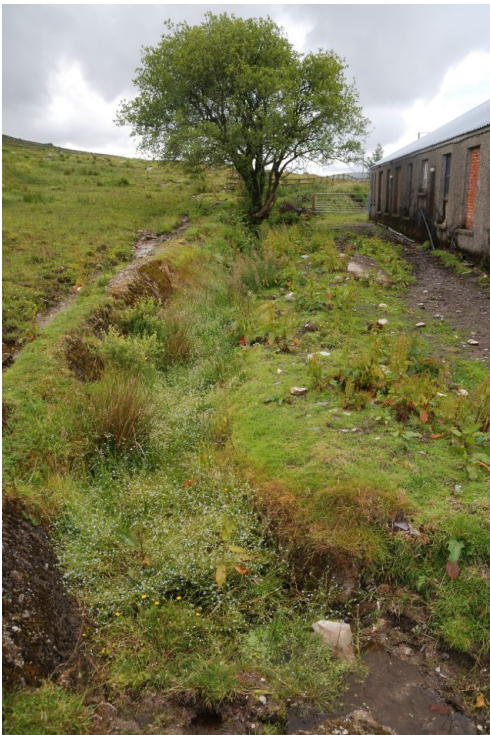
40. A low but substantial concrete retaining wall/dam (centre left) and deep drainage ditch (centre) in front of the station transmitter buildings. The site is extremely boggy and wet in all seasons, and is susceptible to soil movement. The boggy layer impedes the penetration of VLF waves into the acid igneous bedrock below, but the overall characteristics of the ground would nevertheless remain quite poor; the ITU global ground conductivity atlas maps (Recommendation ITU-R P.832-2, 1999, p.10) gives a low-resolution assessment of Wales’ ground conductivity ( 40a ) as a poor, 1 mS/m; seasonal changes at VLF are insignificant (ibid. 3.1, p.2).
