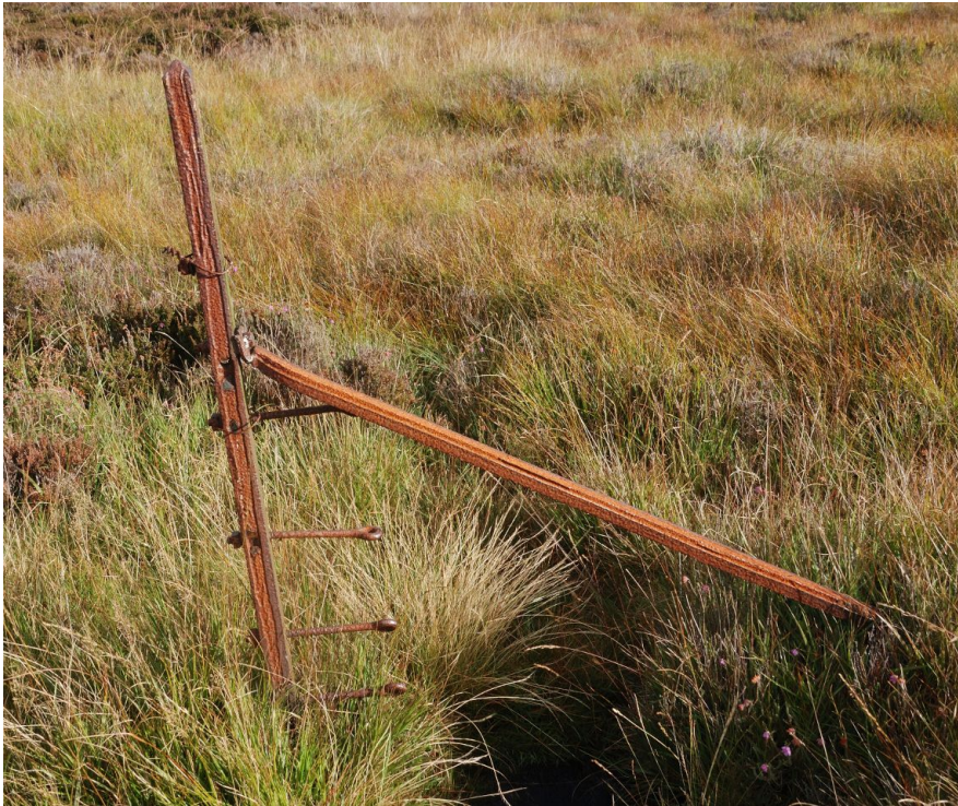
132. One of several remaining 1914 boundary fence posts and strainers, this at the upper northern end of the 1914 site. Upright post 4' above ground level, post 42mm x 42mm, stay 35 x 35mm; 7 x strainers, separated by 8".
