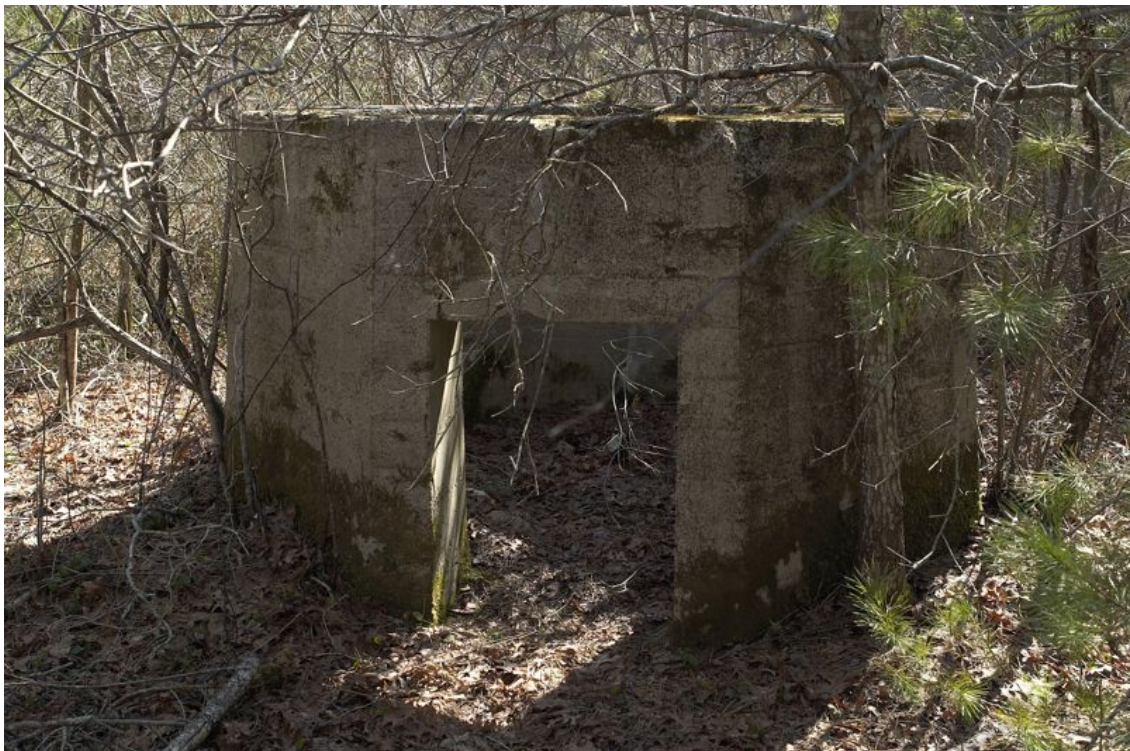
112. Other than the use of horizontal shuttering to construct it, an apparently identical octagonal inductor base at the Marconi station of Marion, MA, USA. Courtesy and © 2008, M. Howells via Sippican Lands Trust.
