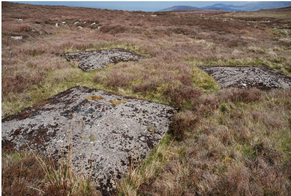
96. The six, 1923 extension masts, running from the top of Cefn Du downhill towards Llanberis, were of very different construction to the 1914 antenna, each being a three-cornered lattice, 400' high. Each of the three concrete bases is ~98" (~8') on a side, of raised tops with a 26"x24" concrete depression made by a mast foot plate in the centre, where eight bolts of \frac{3}{4} " diameter protrude 2" above the concrete. Each base has centres separated by 14'8". 53.121808°, -4.173193°.
