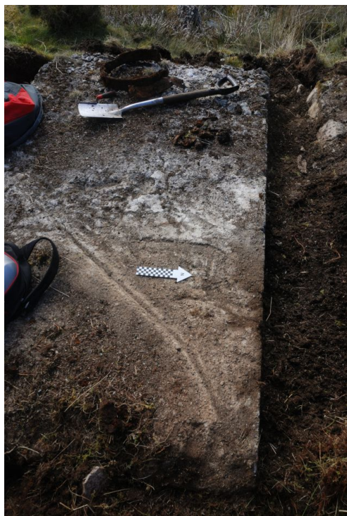
D32 , left: Main platform base after brush cleaning, showing narrow channel, draining to the rear and light impressions in the concrete surface, potentially those of double-bend pipework. The lime-rich concrete surface appears to be somewhat heat-modified at this point. Orientation as per arrow, 1ft gap between bases at far right, incline direction is to top centre (W-NW). D33 , below: aerial view of winder site.
