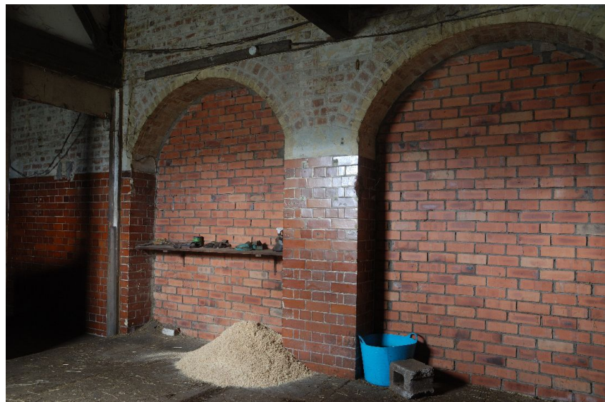
D21 , right: the same arches as in D18, but taken from near the windows at the eastern elevation of the transmitter hall.
