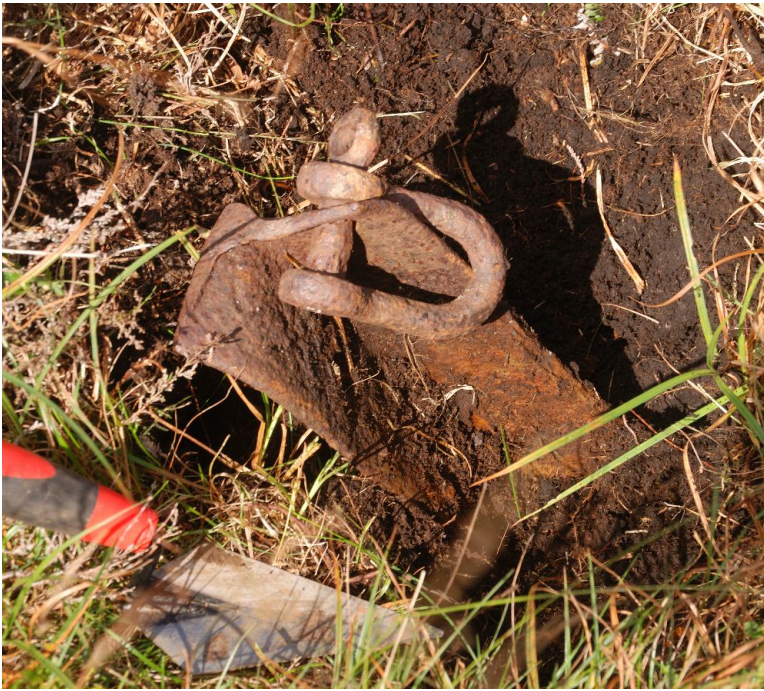
130. 'L'-section steel hammered into the ground, with shackle attached. There are a couple of these around the site, their exact purpose unknown. This example lies adjacent to anchor 6A for the 1914 antenna.
