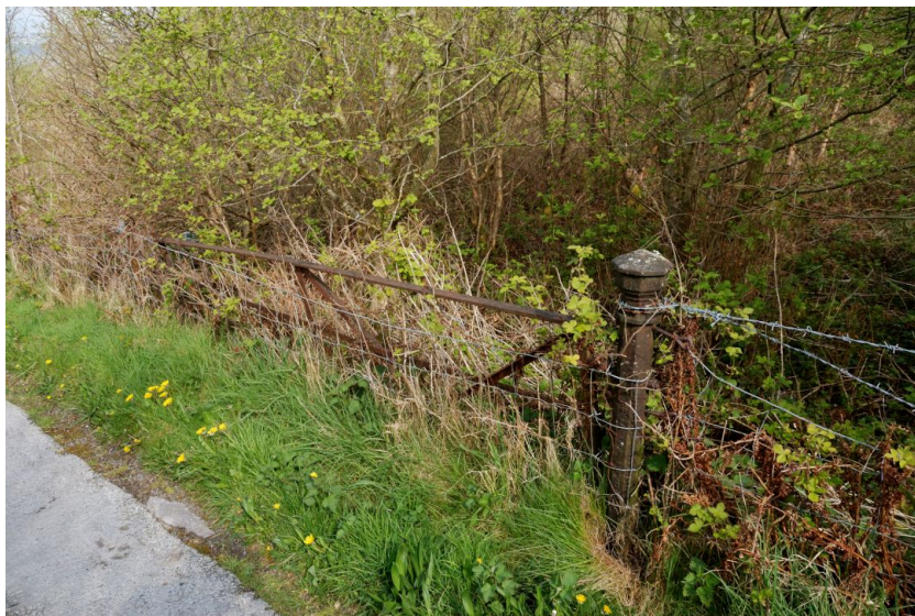
D25 , left: accessway gate, one of two that seemingly overlapped, and ornate iron gatepost by Peerless Wire Fence C o .
