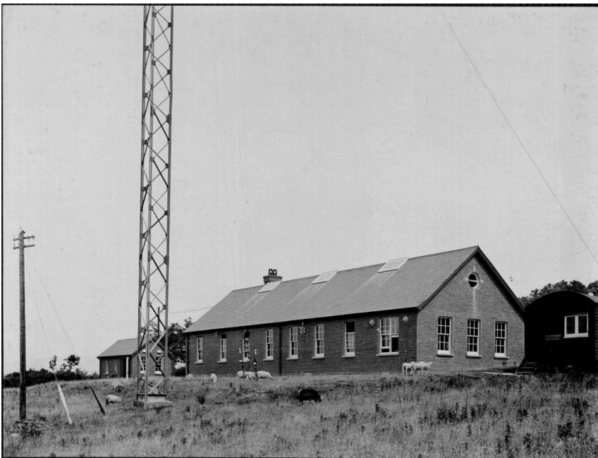
R1. The main Towyn station building. The lattice mast might have been part of an initially single directional Bellini-Tosi frame antenna, but the details are unclear. Later accounts tell of two Bellini-Tosi directional loops, separated by \frac{1}{4} wave (i.e. two mast structures separated by that distance, supporting two loop wires each).
