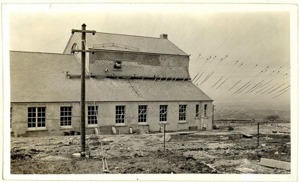
26. Carnarvon transmitter house, antenna and ground feedlines, date unknown, but from the debris and ground disturbance, early-on and certainly not later than 1917, as the same image appears in Bucher ( op.cit. p.294). The 'telegraph' pole at left feed the two of several fence posts in the right foreground, which have multiple wires, the start of the buried earth screen, running into the ground (cf.45). The sloping radiators are fixed, via rod insulators, to a steel beam fixed on or just behind the retaining dam/wall (see 40).
