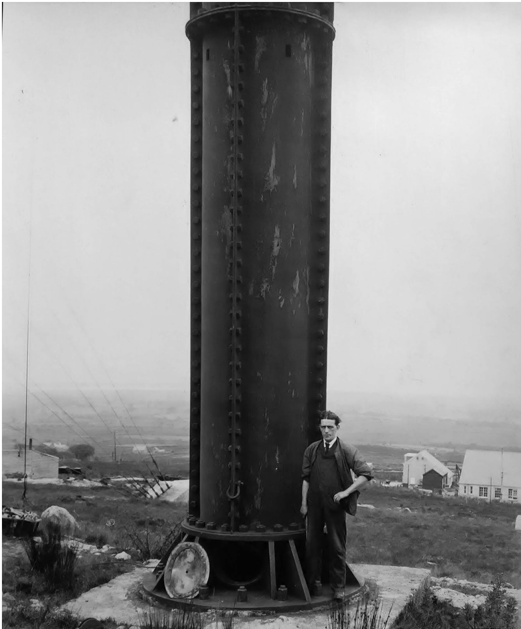
12. Central mast (Mast 2) of the first three masts at the transmitter (western) end of the antenna. A hatch is laid open, giving access to the ladder running to the top gallery, within (The Wireless World, July 1914, p.218). The baseplate at the concrete (6' diameter stud outer to stud outer) is of 16 threaded studs of 2" OD, with two nuts of 2½" OD securing each. The ¼ section mast elements, each 15 feet long, are of fairly thin steel (see 129 ), perhaps ¼" or less thick, with 29 bolts joining each vertically and 20 radially. Rectangular holes, of unknown purpose but potentially related to the raising mast platform used during erection, are seen in the upper centre of each section – also seen in images of Marion (USA) and Ullandhaug (Norway) masts. The lower part of the mast was 3'6" in diameter (presumably internal, but not known – both referenced accounts fail to indicate), the upper part 2'6" (The Wireless World, July 1914, p.217 and Marconi station pamphlet in MS.Marconi.198). Note the 7-stay anchor at rear left of mast and what is probably a triatic halyard, at far left. The item on the floor at left is difficult to identify. The lanyard is behind, rather than connected to it. There are no smaller steel masts either side of the transmitter house at this time. Bodleian Special Collections MS. Photogr. c.243, document P.2092. Date unknown, but pre-elevated counterpoise, and therefore pre-1921, probably around 1918.
