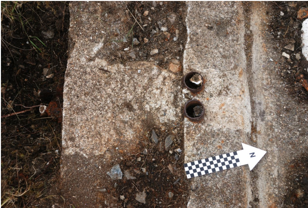
84. After a couple of days' drying, the much brighter concrete (and distortion of the outer edge of the internal drainage channel) clearly confirms the original 1923 double ATI concrete base was cut into (ca. 1925) in order to install a new feedline. Steel tubes, externally threaded, OD = 2¼", lead cable sheath diameter ca. 30mm. An additional wire (lead cable sheath diameter ca. 15mm), possibly the connection to the GLC (lower) earth screen, to the east of the porch, in the MUU (upper)-facing part of the ATI house ( 85 , below), seems to have been in place from 1925. Tube (unthreaded exterior) for this cable is OD of 2½", ¼" wall thickness. The hole for the cable to emerge from the base was found, but no trace of the cable remains.
