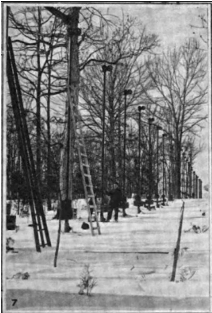
30. A poor copy image from The Wireless World , May 1914 (p.95, image 7 of a montage of 8), showing a row of wire tensioners at the Marconi, New Brunswick station, USA. Note pulleys at top, facing the antenna (off scene, to right), and coaxial weights near their bases. Height of the bases, taking the man to be an approximate guide, is about 22 feet. Chains attached to the bottom of the poles (just visible to the left of the ladder base, and still to be found at Marion and one base at Carnarvon) are of unknown function at the time of writing, but possibly for limiting the upwards extent of the weights' movement. See also 31-34.
