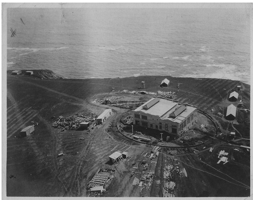
46. Whilst mobile, boggy ground has obliterated the fine detail of the lower reaches of the Carnarvon antenna site, a photograph of the earth screen – on very dry ground – at Bolinas, CA, shortly after installation shows how an earthing ring (which was irrigated by a 3/4" water pipe at the station) of 100 foot radius surrounded the transmitter building, with linear, buried wires leading away in all directions revealed by ground scars. The screen was led towards and over the cliff, and a connection, via a rectangular, 980 square foot plate, to the sea was made (Bill Ruck to Rowlands at Bolinas, pers comm 11/01/2023, with contemporary schematics examined but not released for publication). Image courtesy California Historical Radio Society.
