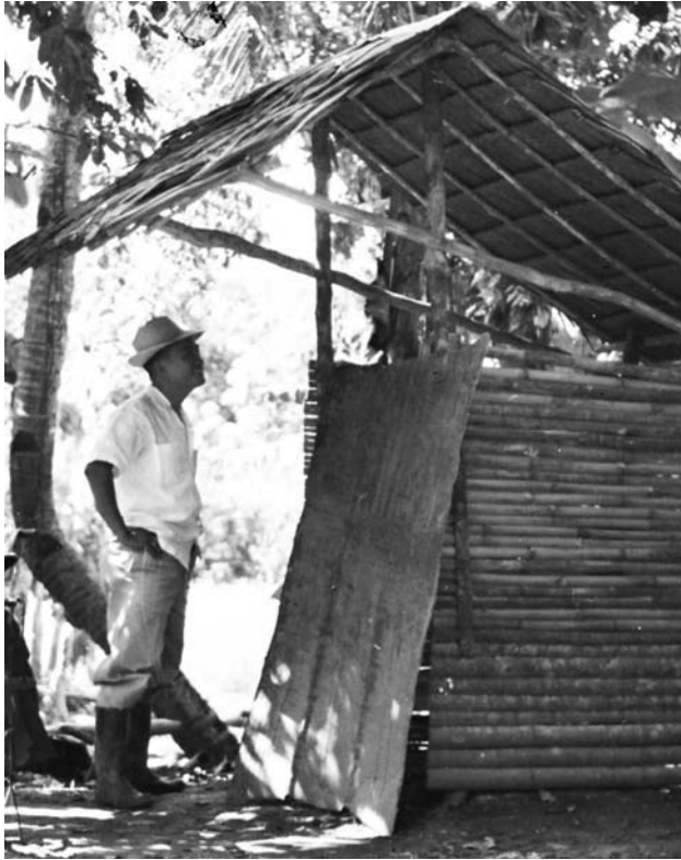
Figure 16.12 Government-encouraged pit latrines in the Philippines serve as a means to prevent schistosomiasis.
