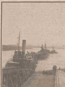
The Caisson Bridge, Grangemouth, being towed to dry dock for overhaul.
