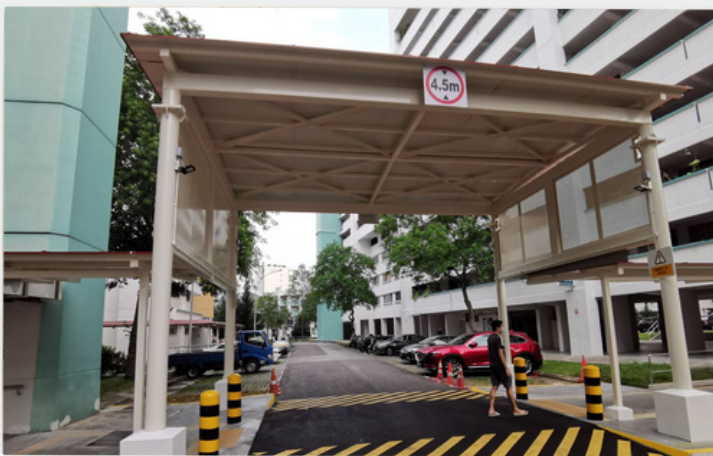
New High Covered Linkway Between Block 131 to 119 Bukit Batok West Avenue 6
