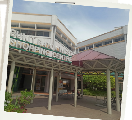
NEW ROOF PANELS
