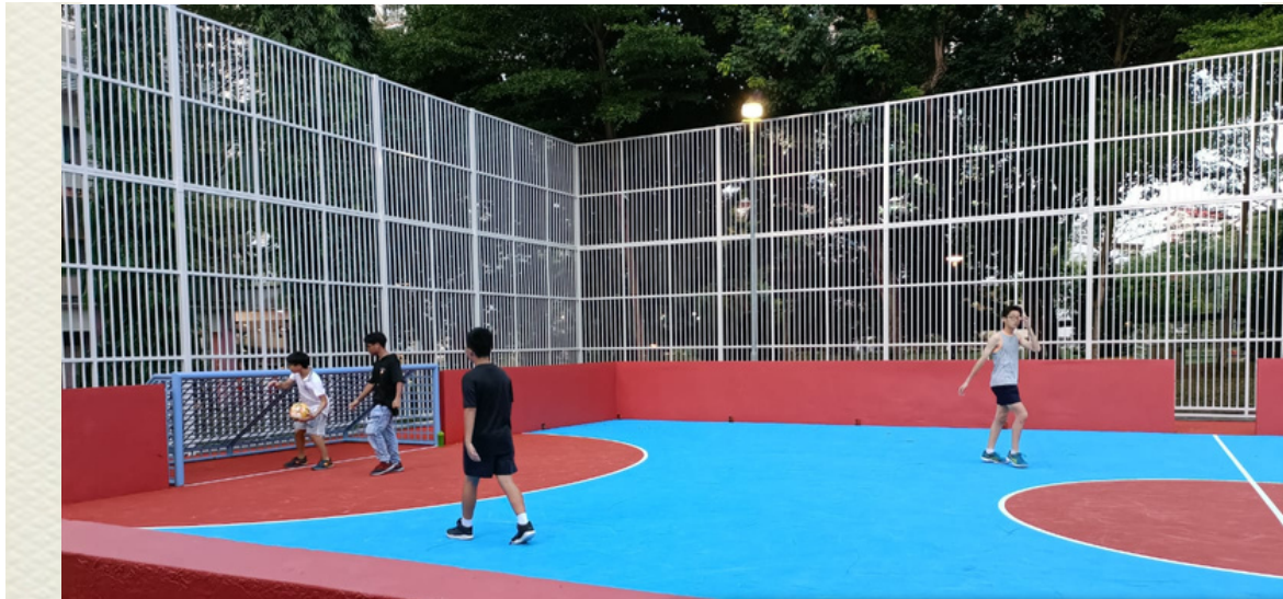
Refurbished Street Soccer Court & Fencing Block 226 Bukit Batok Central
