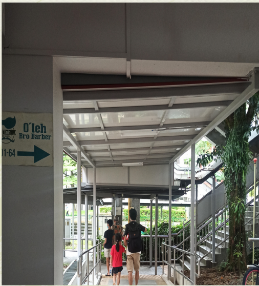
New Low Covered Linkway From Block 642 Bukit Batok Central to Pedestrian Overhead Bridge
