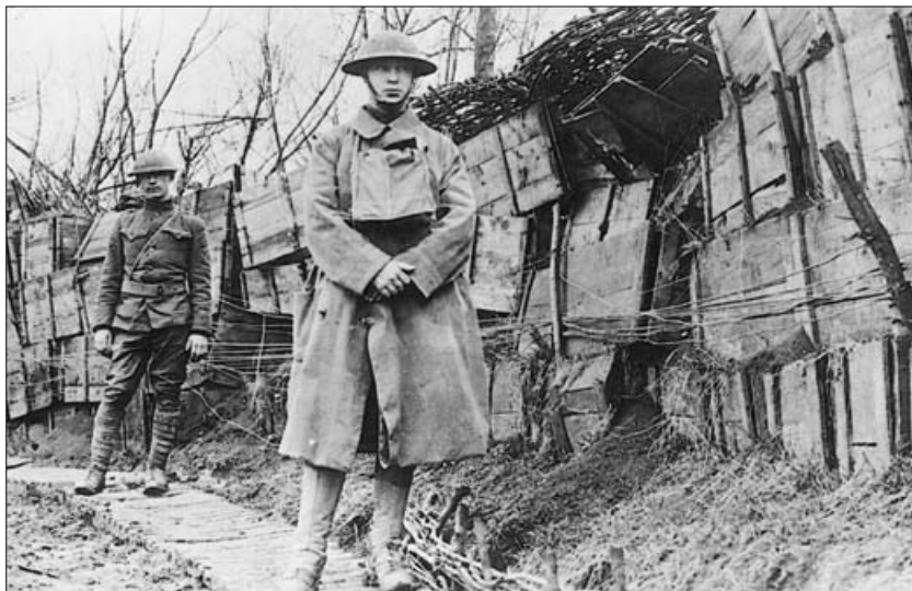
When the lines ran through particularly difficult terrain, such as swamps, instead of digging trenches the soldiers would construct barricades. This is an example of one of those barriers.
