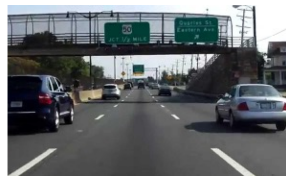
Pictured: Pedestrian bridge on DC 295 in NE Washington before the collapse.
