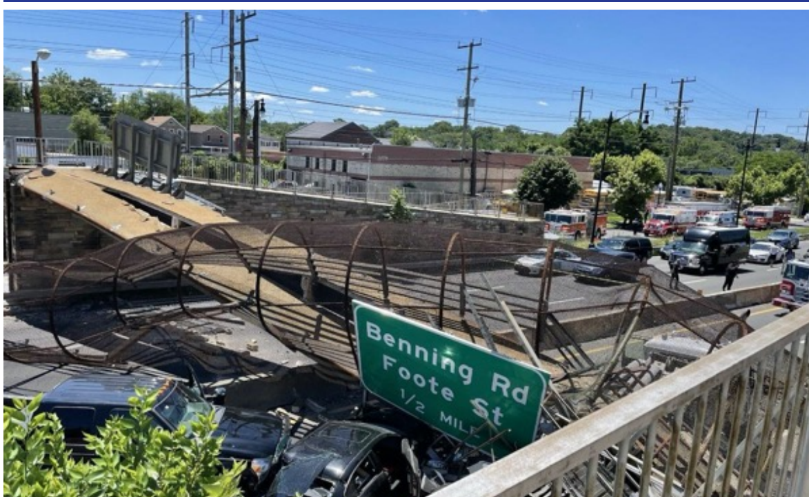
Pictured: Pedestrian bridge collapse on DC 295 in NE Washington DC
