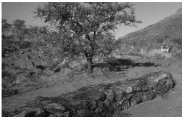
Check dam, Eastern Cape, South Africa
