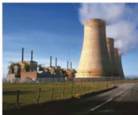
FIGURE 15.1.1 Chapelcross Nuclear Power Station, Annan, Dumfries, Scotland.
