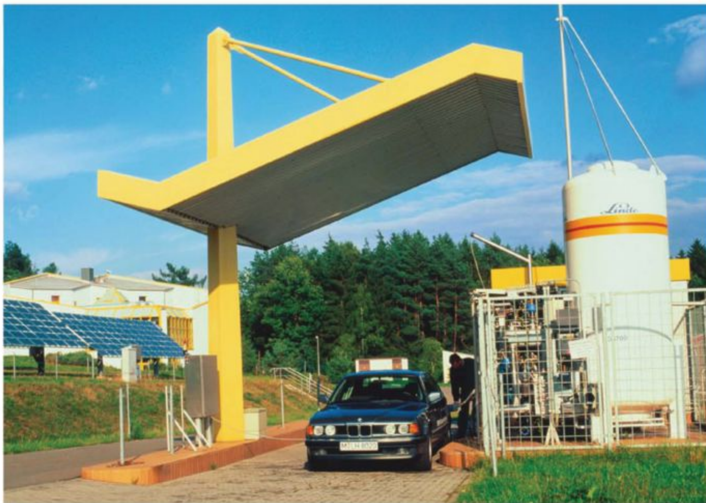
FIGURE 2.4.11 A liquid-hydrogen filling station in Germany. The test car is being filled with liquid hydrogen fuel (from the large white tank on the right) at a hydrogen filling station. The converted car can run for 300 km on a full tank of liquid hydrogen.
