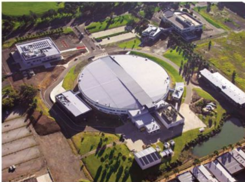
FIGURE 7.3.1 The Australian Synchrotron is about the size of a football ground. This size is necessary to contain the electrons which are travelling at almost the speed of light as they zoom around the storage ring.
