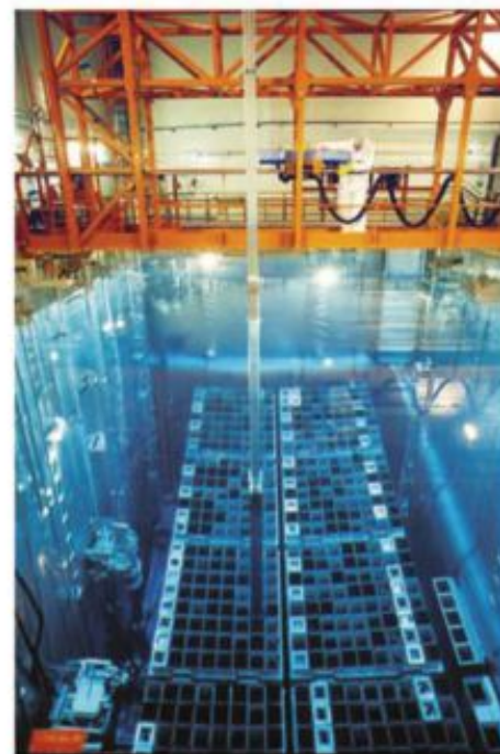
FIGURE 15.2.9 Forty per cent of the world's spent fuel rods are permanently stored in cooling ponds.
