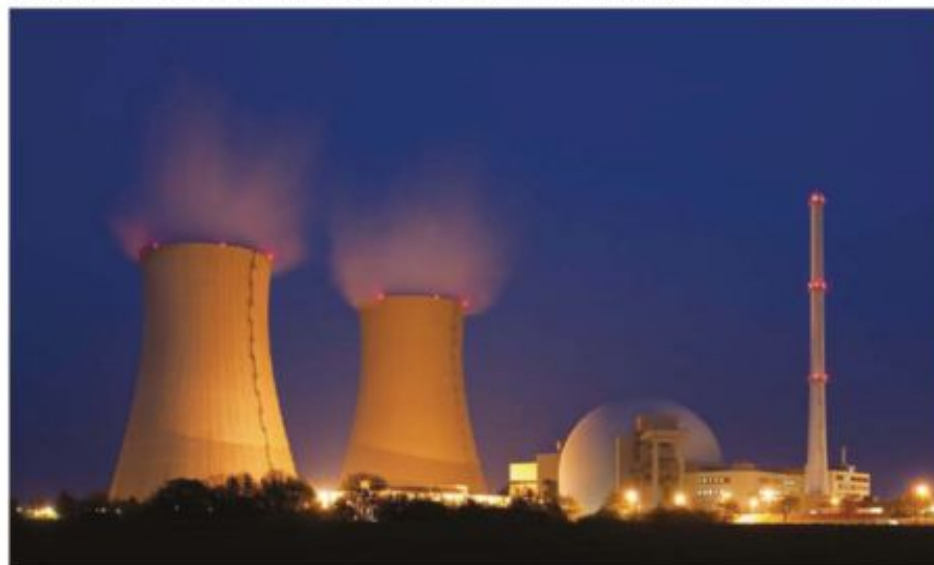
FIGURE 15.2.2 Nuclear power plant at night in Grohnde, Germany. On the left are the cooling towers with water vapour; on the right is the reactor.
