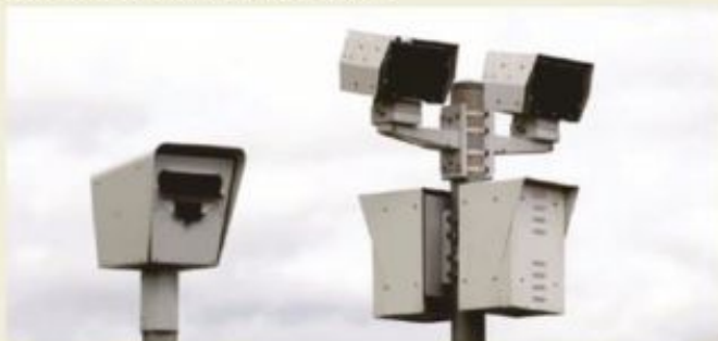
FIGURE 9.1.7 Speed cameras on poles.
