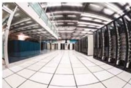
FIGURE 17.3.1 CERN Computer Centre. This computing centre extends over two floors and has 17 000 processors with 85 000 computing cores, as well as computer tape and disk storage capacity for over 200 petabytes of data.
