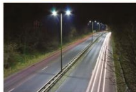
FIGURE 7.4.1 Sodium vapour lamps have been used for street lighting for many years. The characteristic orange colour is the result of sodium's emission spectrum. These are being replaced by LEDs which produce white light and are much more energy efficient. In both types, light is produced by electron transitions between energy levels.
