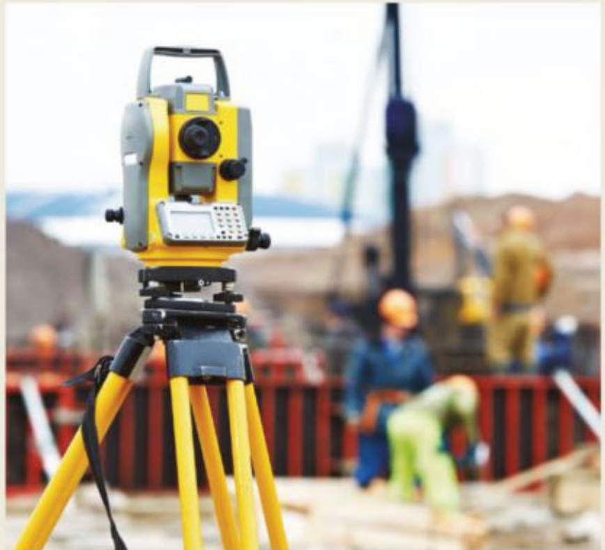
FIGURE 8.2.9 Surveying equipment being used on a building site.
