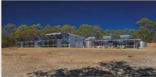
FIGURE 2.4.4 The Sustainability Learning Centre in Hobart has been designed using the principles of passive solar design and has a low carbon footprint.
