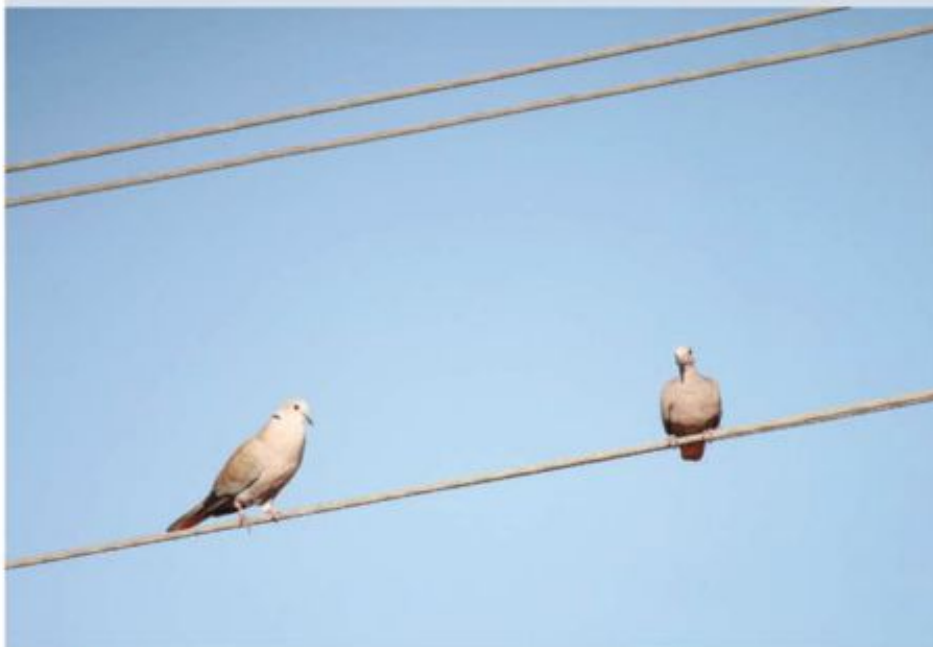
FIGURE 3.3.7 There is no potential difference between each bird's feet.
