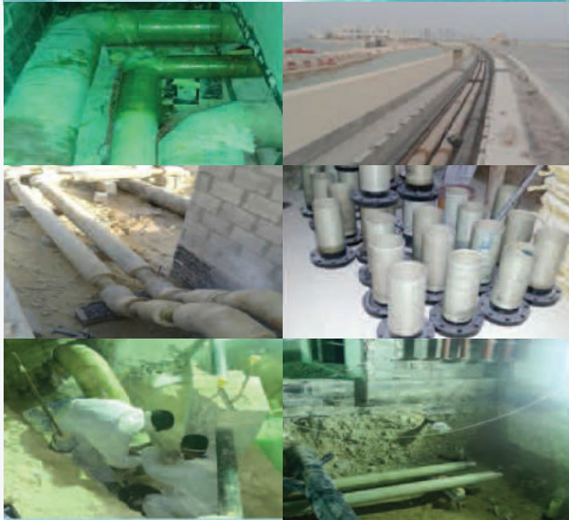
Island Project Villa and Service Compound
