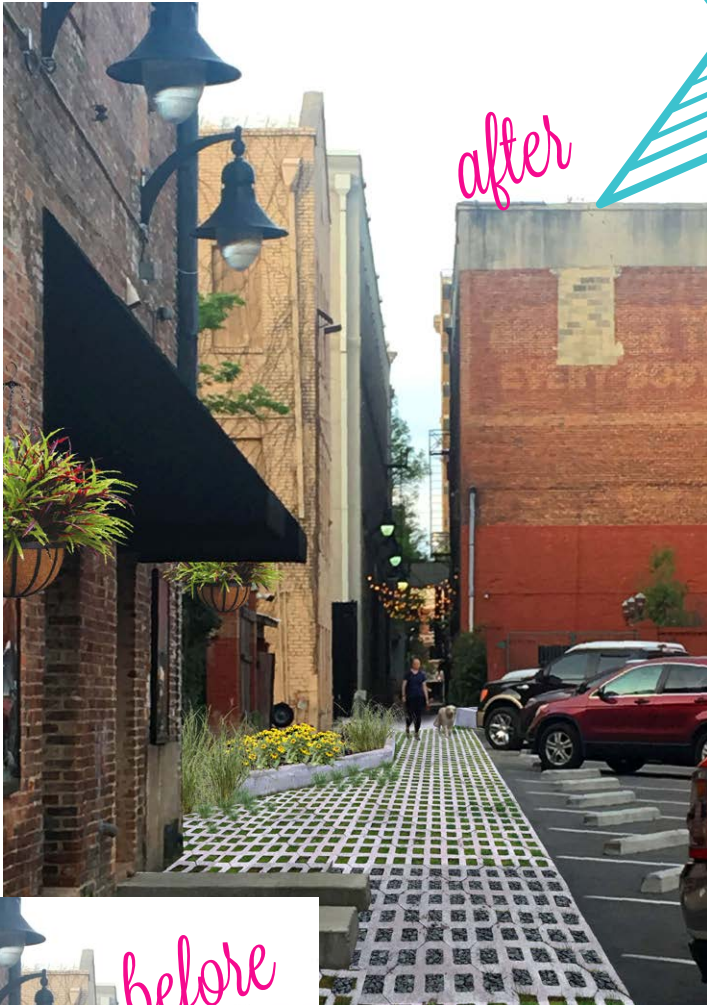
Alley makeover implementing green stormwater infrastructure techniques.
