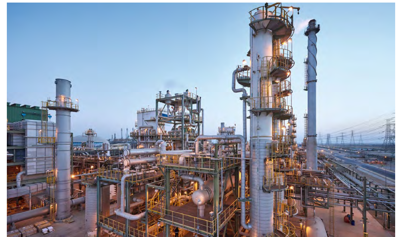
Figure 3: Amine wash-based CO 2 capture process from syngas
