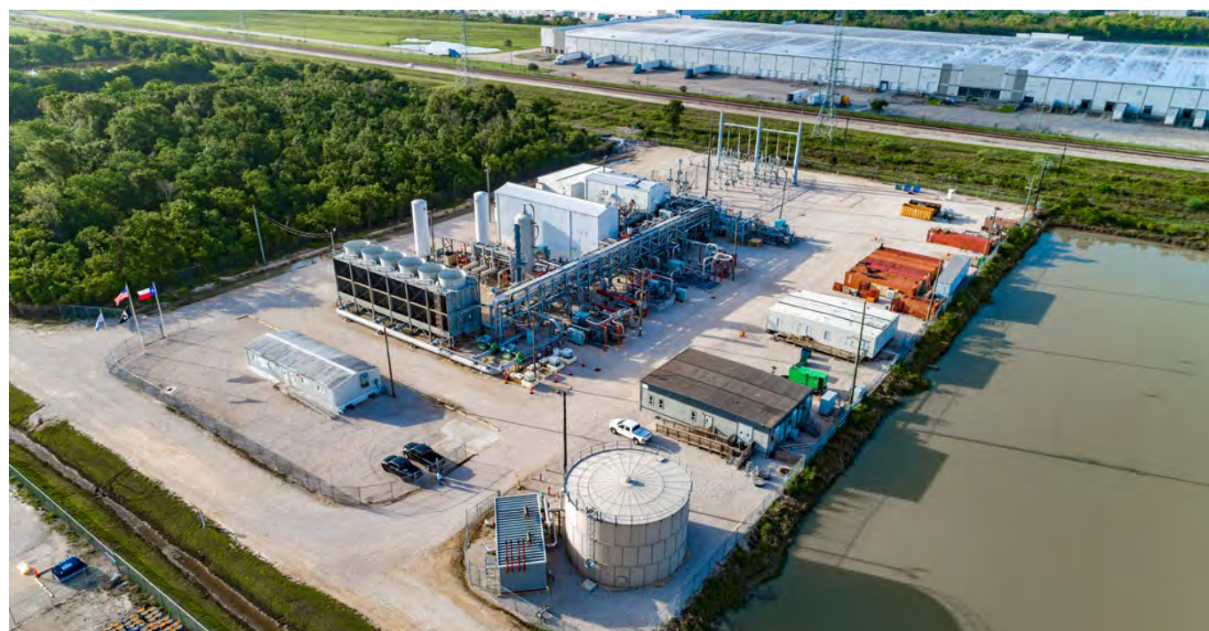
Figure 2: NET Power's La Porte Demonstration Facility
