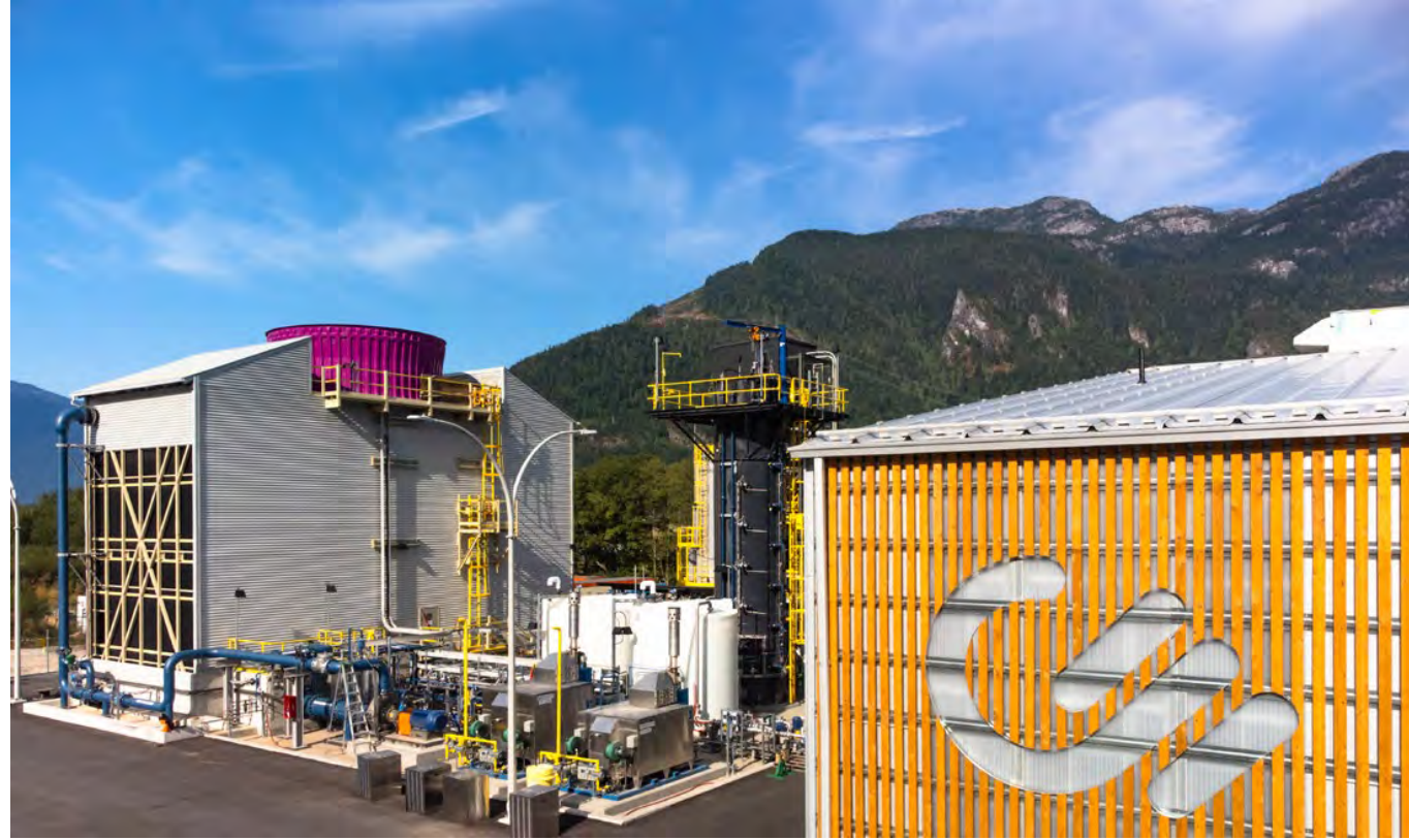
Carbon Engineering's Innovation Centre and Research & Development Headquarters located in Squamish, Canada.
