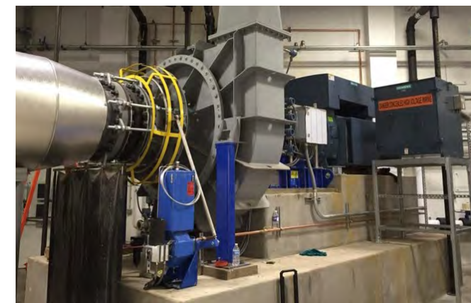
Howden Turbo fans to produce bioethanol from CO 2 at Arcelor Mittal
