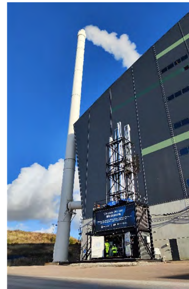
CapsolGo® unit 1 at Filbörnaverket, Helsingborg, Sweden.
