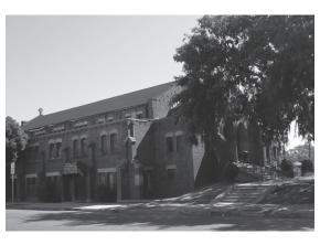
office, and fellowship wing, for a cost of \$75,000. You can see on the side where the old portion was removed (two bays back) and the new section added. Pre-cast cement elements were used (arches around doors, tops of buttresses).
