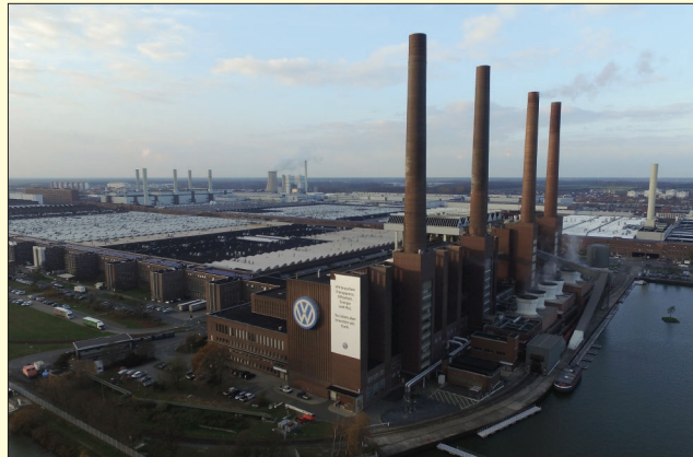
A Volkswagen factory, including its heating plant with four chimneys, in Wolfsburg, Germany.
