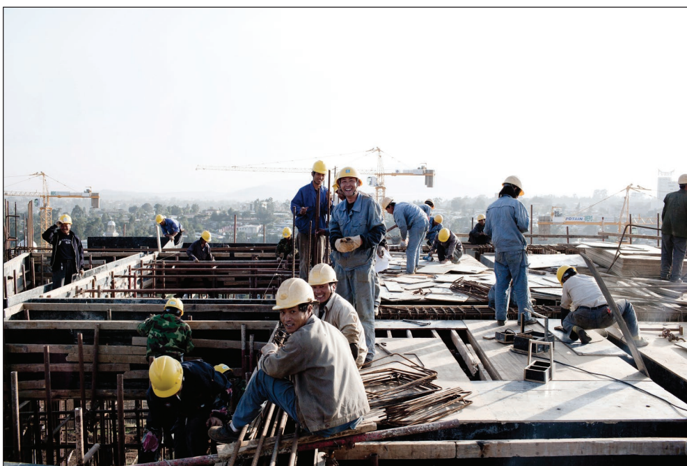
Chinese construction workers build the new African Union Buildings in Addis Ababa, Ethiopia.
