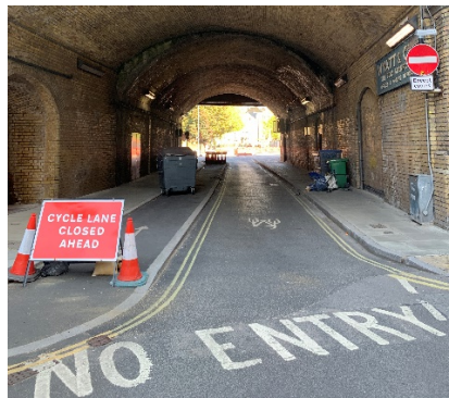
Impeded access to delivery side entrance
