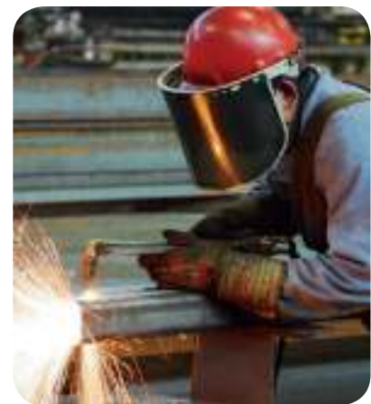
Cutting with an oxy-acetylene torch requires a permit to work
