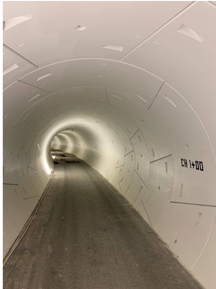
Figure 25 – Sample Incremental Tunnel Marker
