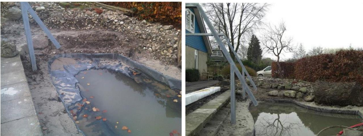
Filling the pond liner with water to settle.
