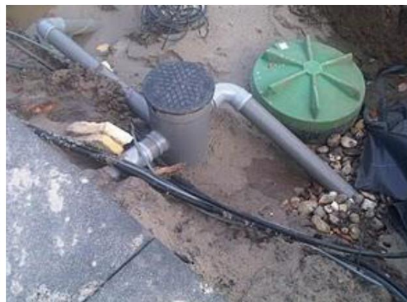
The filter being installed. In the right picture, the bottom pipe is the inflow, the left hand pipe leads to the cistern and the right hand pipe is the overflow into the gravel pit.
