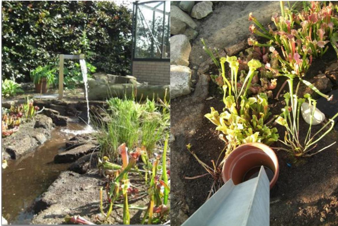
Left: Water feature pumping rainwater from the cistern. Right: The H-profile gutters drain into dug-in terracotta pots (2011)
