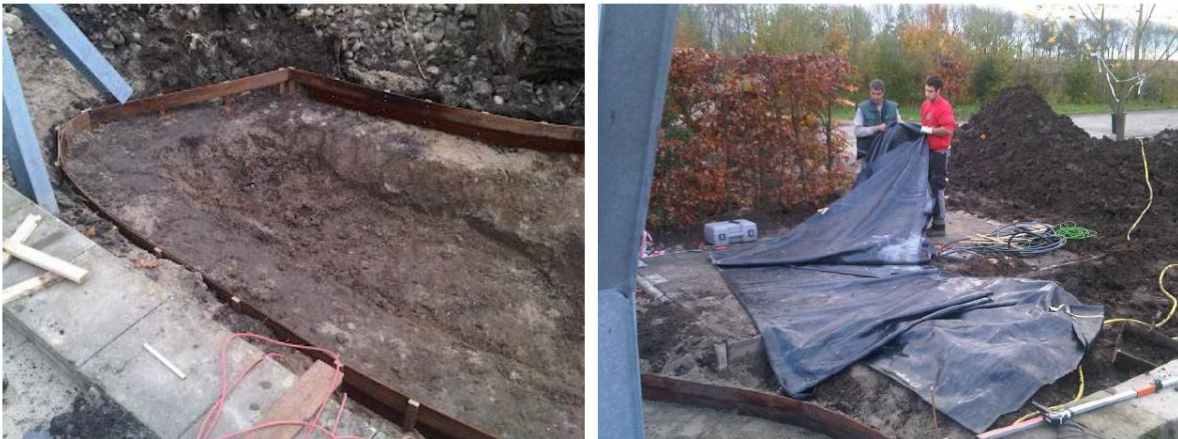
The hardwood edge around the pond and unfolding the pond liner.
