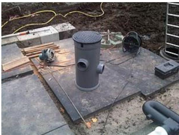
The filter being installed. In the right picture, the bottom pipe is the inflow, the left hand pipe leads to the cistern and the right hand pipe is the overflow into the gravel pit.
