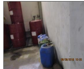
Photo of non-conformity No Secondary Containment provided for chemical.JPG
