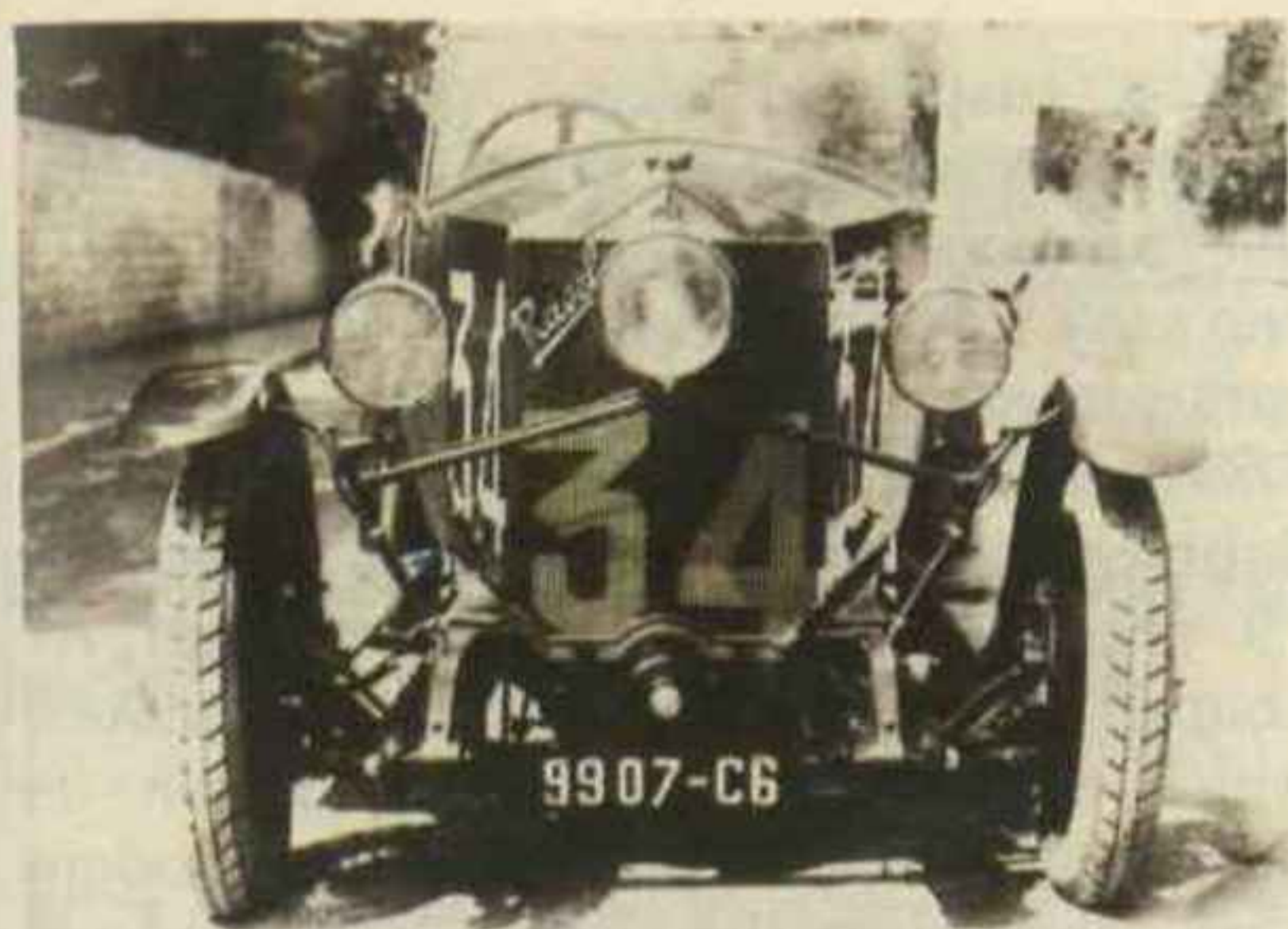
Far left; the 2½-litre Ravel which, driven by Van den Bossche-Smeets, ran the distance but outside the time limit, in the 1925 Le Mans 24 Hours. Its headlamps were arranged to swivel with its front wheels. Below left; a Ravel on a typical French highway of its period. Left; the 1926 Le Mans car. Note triple headlamps. All photos from the Douezy and Dornier Collections
