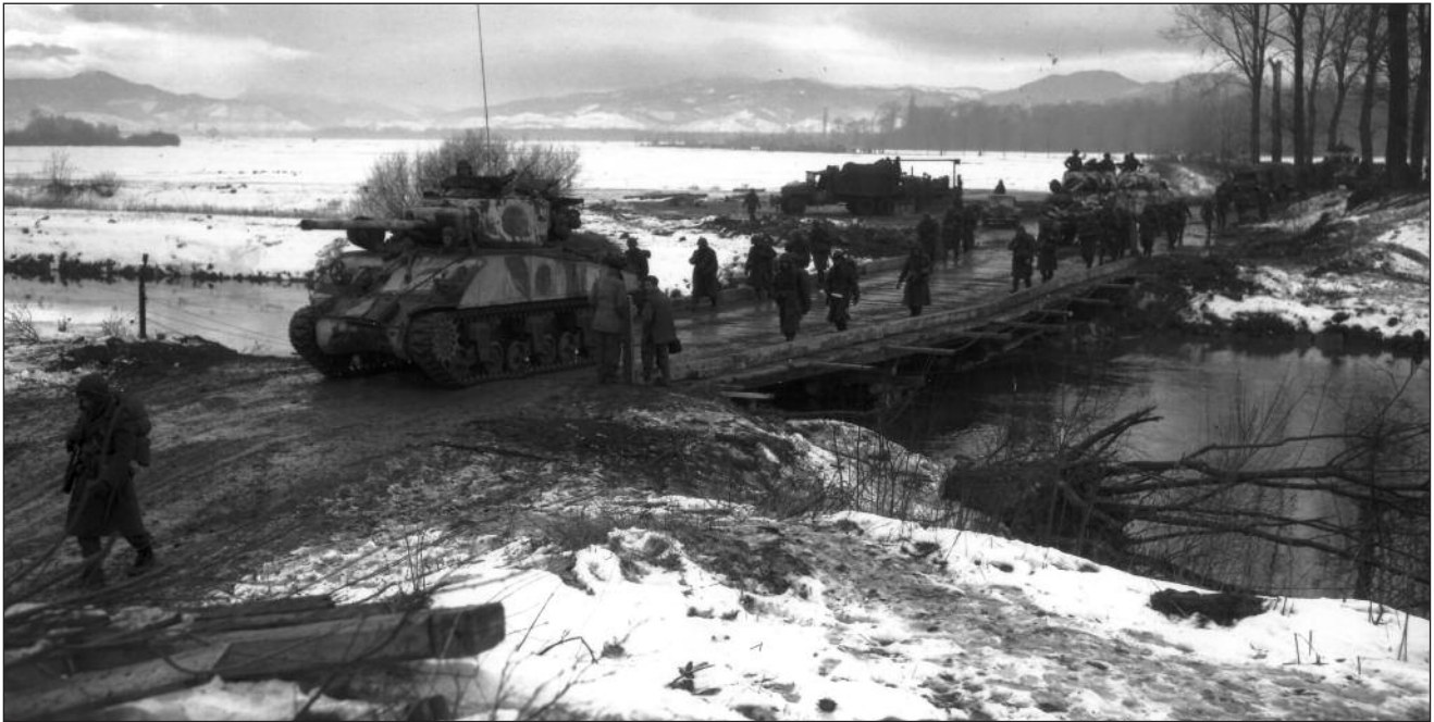
This picture captioned 'in the Riedwihr area' slots perfectly into our story at this point because it shows one of the treadway bridges established over the Ill river although it does not say
