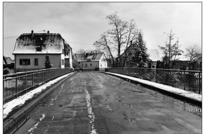
Here engineers complete the construction of a pontoon bridge across the Ill at Kogenheim, probably on the 26th. (ECPAD) Right: A lucky fall of snow enabled Jean Paul to take a 'seasonal' comparison.
