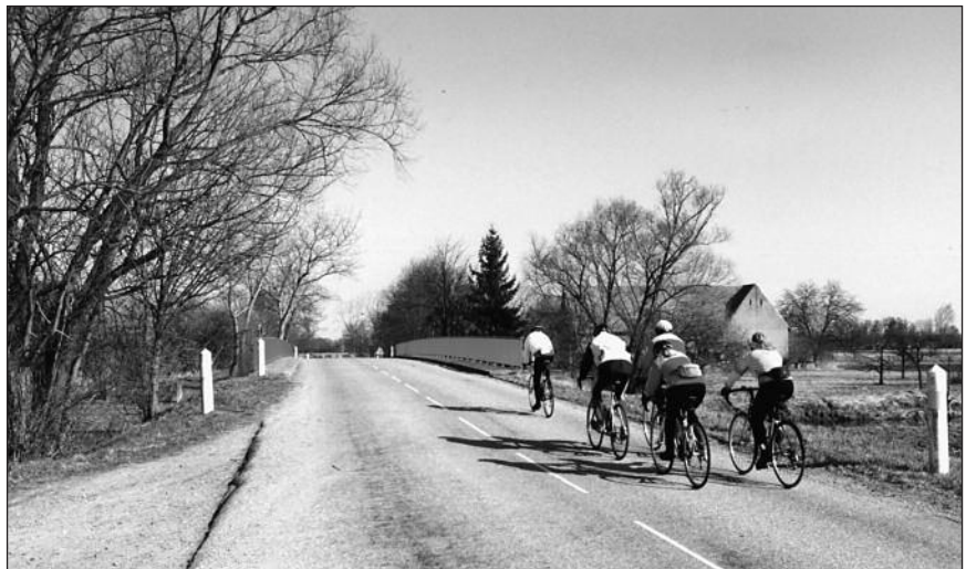
This is the bridge at Maison Rouge as it appears today, looking eastwards. Lieutenant John F. Harmon drove his Sherman up the western ramp — just as these cyclists are doing — but when the tank reached the centre span, the bridge collapsed and the tank fell into the river.
