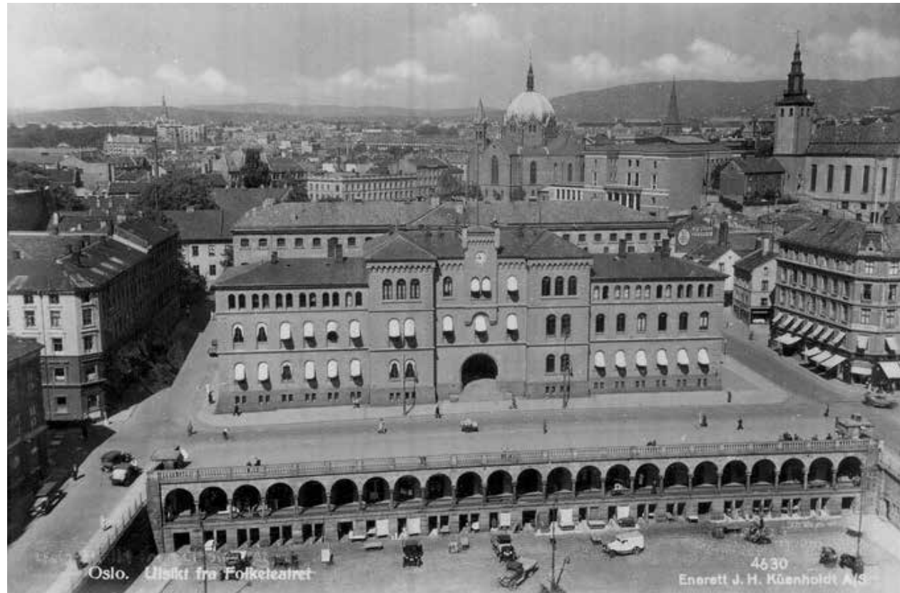
M llergata 19 in Oslo, seen from Folketeaterbygningen in the 1930s. Behind the police station one can discern the prison buildings at Grubbegata.
