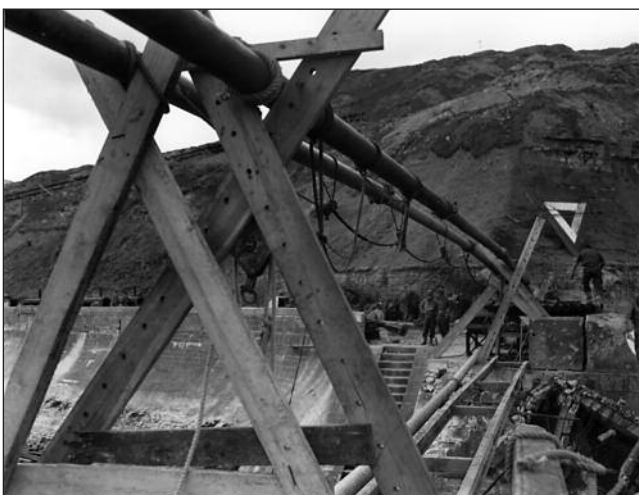
Where the Western Mole (the Quay Letournier) had been damaged by landing craft during the great storm which hit the beaches on June 19, engineers improvised a suspension support to take the lines over the breach. (USNA)
