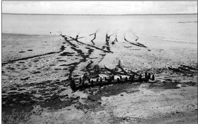
The pipelines to Cherbourg (code-named 'Bambi') had to draw their fuel via the Isle of Wight. Left: Adrian Searle pictured the remains of the 12 lines coming ashore in Thorness Bay from
