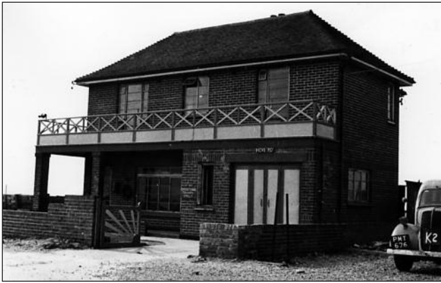
Left: The main pumping control for the British end of 'Dumbo' — the code-name for the Dungeness operation — was located in
