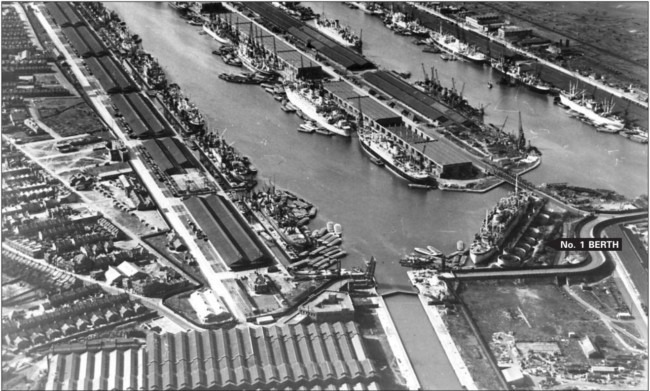
In this early post-war shot of the King George V dock, the storage chambers on No. 1 Berth, just to the right of the lock, still appear to contain unused cable. On the left one can see the bomb sites of Silvertown hit on Black Saturday (September 7)
