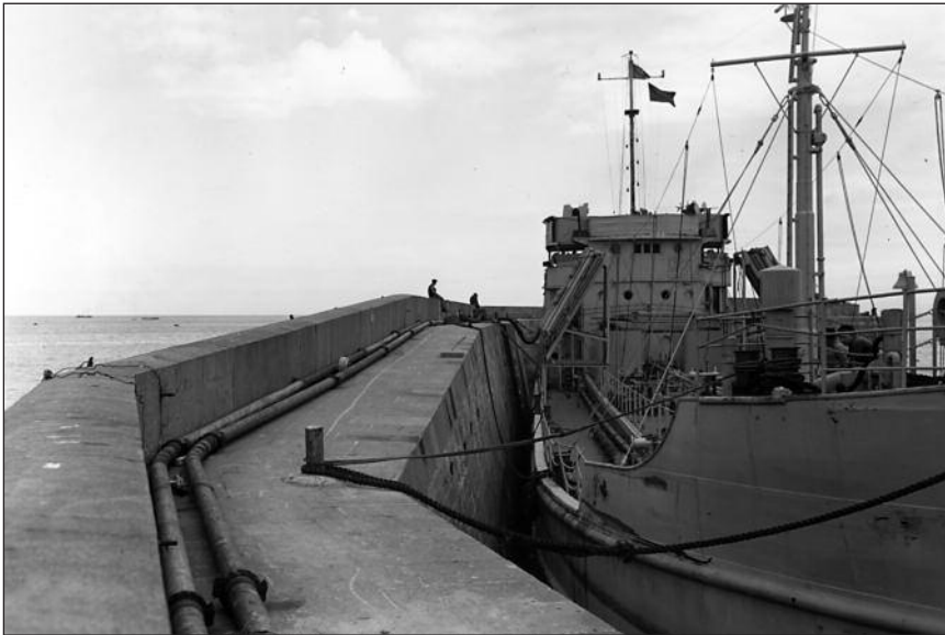
At the joint US-British harbour at Port-en-Bessin, which lay on the boundary between the two forces, two 'Tombola' discharge points were provided. As shown in this picture, the first pipeline was for smaller tankers which could dock against the mole while the other was buoyed 1,000 yards out to sea to permit the transfer of petroleum from larger vessels. (USNA)
