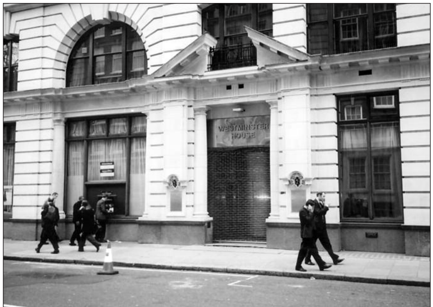
The headquarters of the Petroleum Warfare Department, under whose auspices Pluto was produced, were located in Westminster House in Dean Stanley Street, Millbank. The building is now used in part by Lloyds TSB bank.
