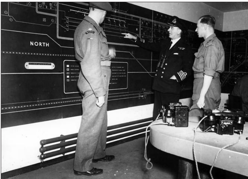
Captain J. F. Hutchings — the commander in charge of the naval side of Pluto — inspects the control board which indicated the flow rate of fuel in each pipeline to France. With him are Major Dagger and Captain Gordon. (IWM)
