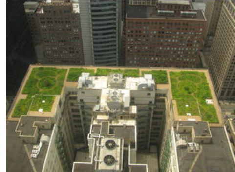
Figure 5 - Example of a green roof on Chicago City Hall (Razavi,2010,9)
