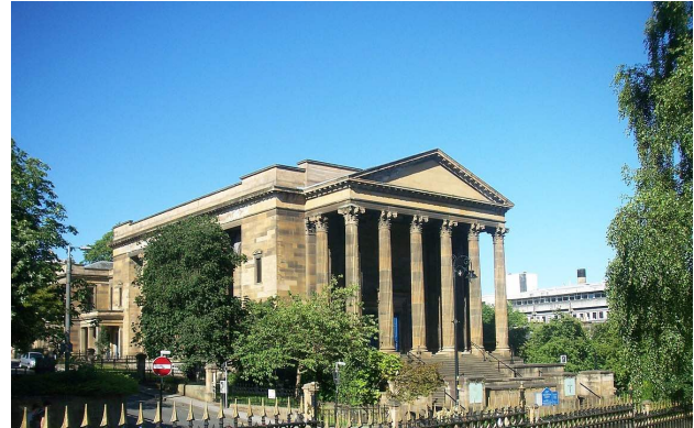
Figure: Wellington Church, University Avenue ( https://en.wikipedia.org/wiki/Wellington_Church ).
