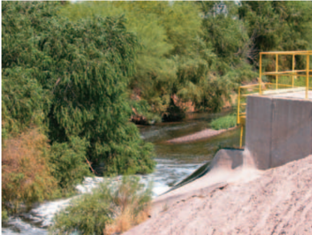
Figure 26.21 Effluent outfall of the Roger Road Wastewater Treatment Plant in Tucson, Arizona. Here, extensive growth of vegetation due to the effluent produces a riparian habitat. Photo courtesy K. L. Josephson.
