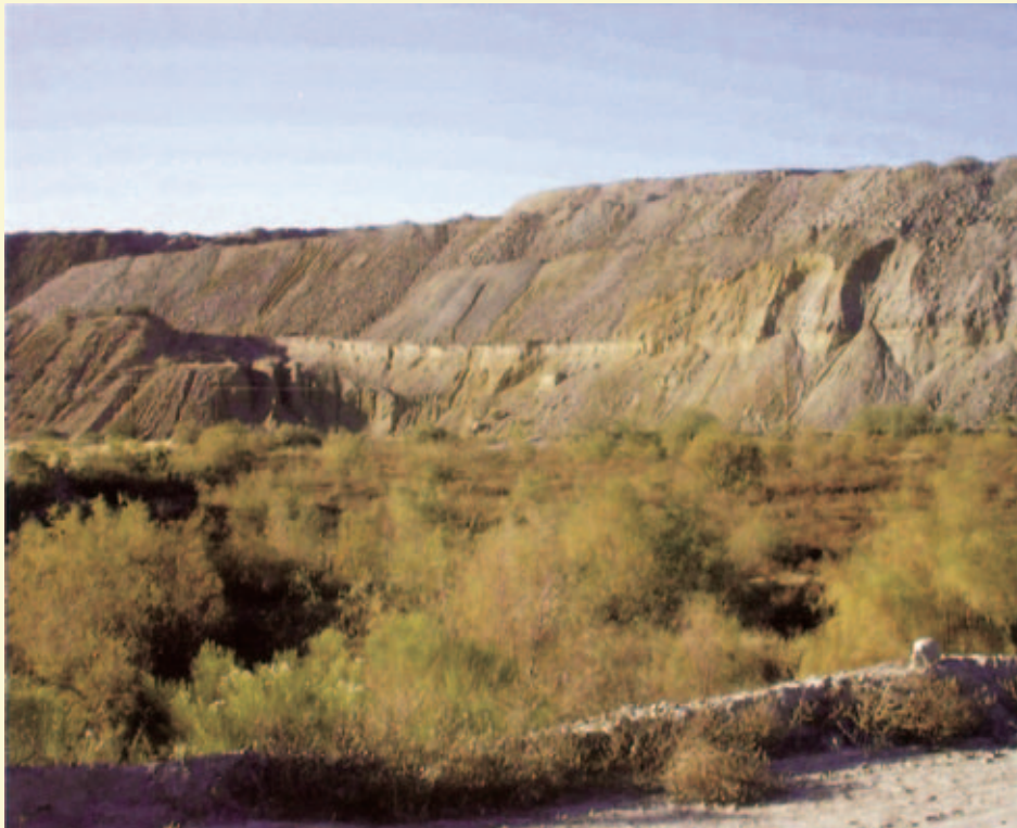
Figure 20.4 Mine tailings three years after biosolid application. From Environmental Monitoring and Characterization © 2004, Elsevier Academic Press, San Diego, CA.
