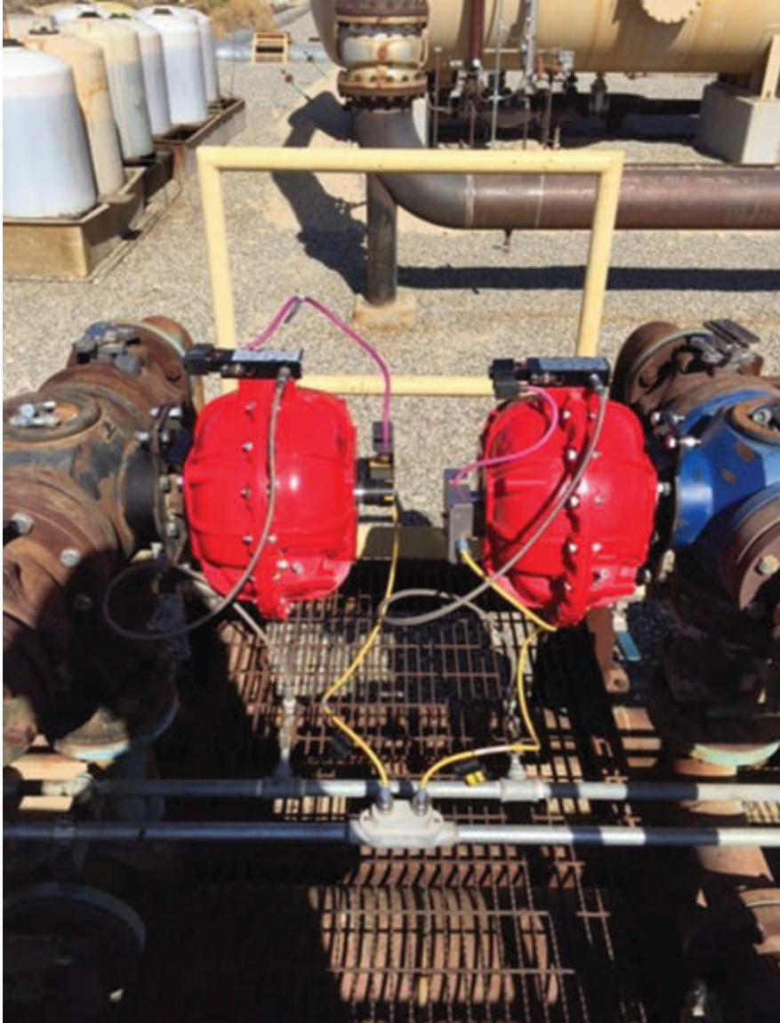
New generation fail-safe actuator without the use of springs for better durability, safety, efficiency and cost. New generation actuators fit where rack and pinions can't.
