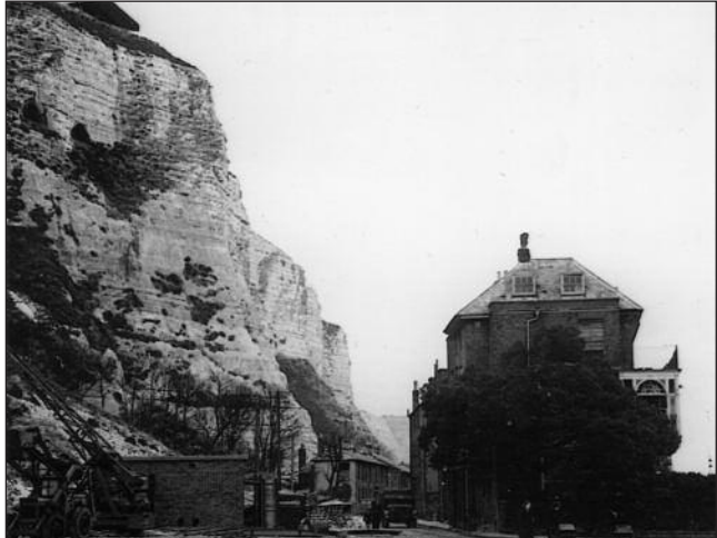
Left: The security of the new HQ was tested by commandos who easily gained access by climbing the spoil heap on the left
