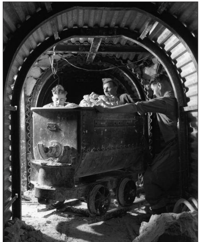
Left: Sappers removed only enough rock to enable each section of the steel shutter to be put in place. The lightweight Holman pick was ideal for cutting into the chalk. Above: The spoil was dumped through the cliff face. (IWM)
