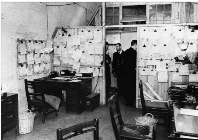
These two photographs are part of the same series so they may show the other end of the same room as the corridor — the vertical wood boarding on the right, is on the correct side.
