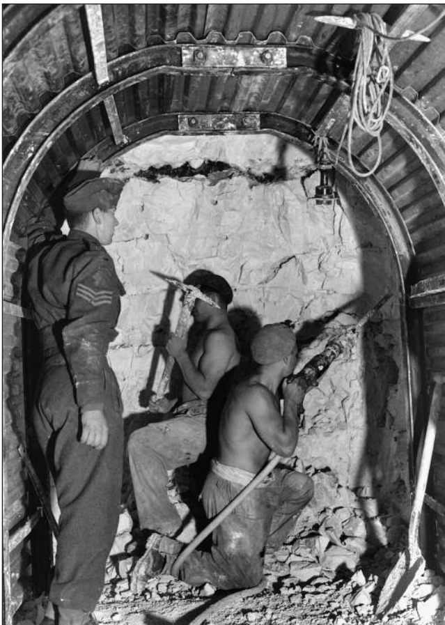
Left: Sappers removed only enough rock to enable each section of the steel shutter to be put in place. The lightweight Holman pick was ideal for cutting into the chalk. Above: The spoil was dumped through the cliff face. (IWM)
