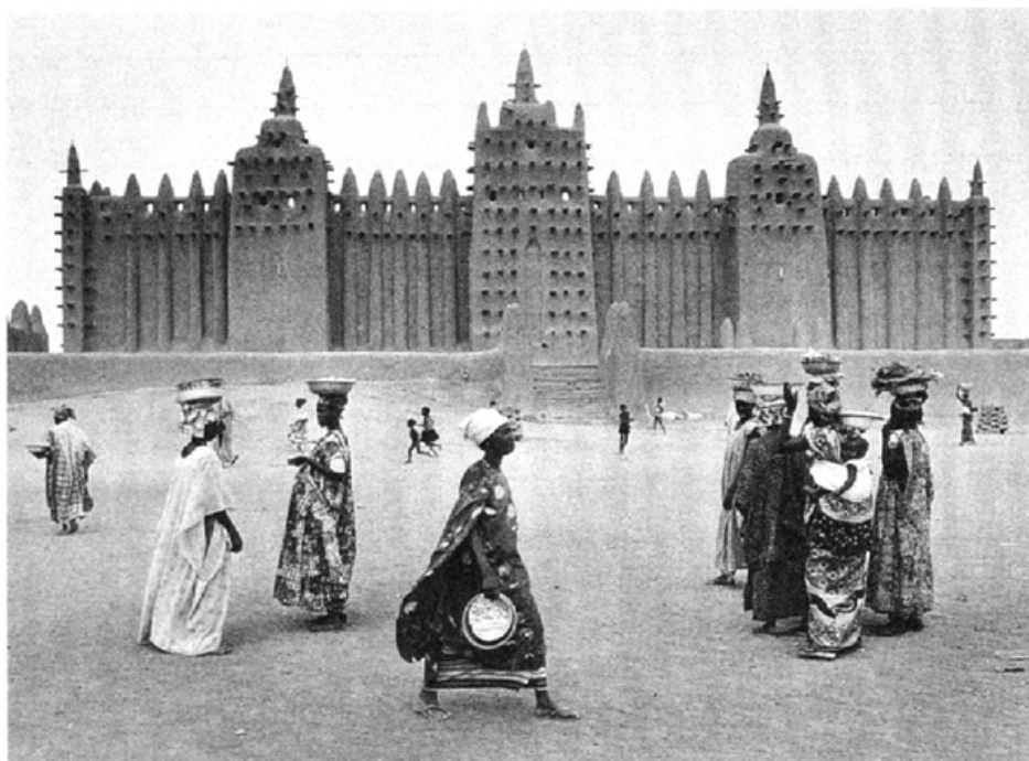
This mud-brick mosque in Jenne, Mali, was constructed in the fourteenth century and is the oldest in Africa. The mud, which washes away in the rain, needs continual renewal—hence the built-in “scaffolding” of the structure.
