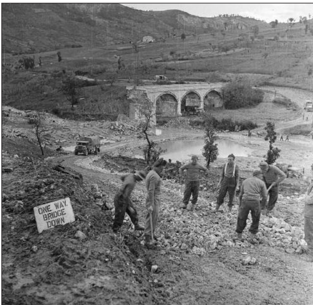
Left: The Germans left a trail of destruction as they retreated up the Italian peninsula, with several bridges on the New Zealanders' route blown. To get around this one, engineers of the 6th Field Company, INZE, built a road and a ford over the river next to the broken bridge. The picture was taken by George Kaye, the official New Zealand photographer, on November 19, 1943. Right: Although the official caption states that the bridge and ford were
