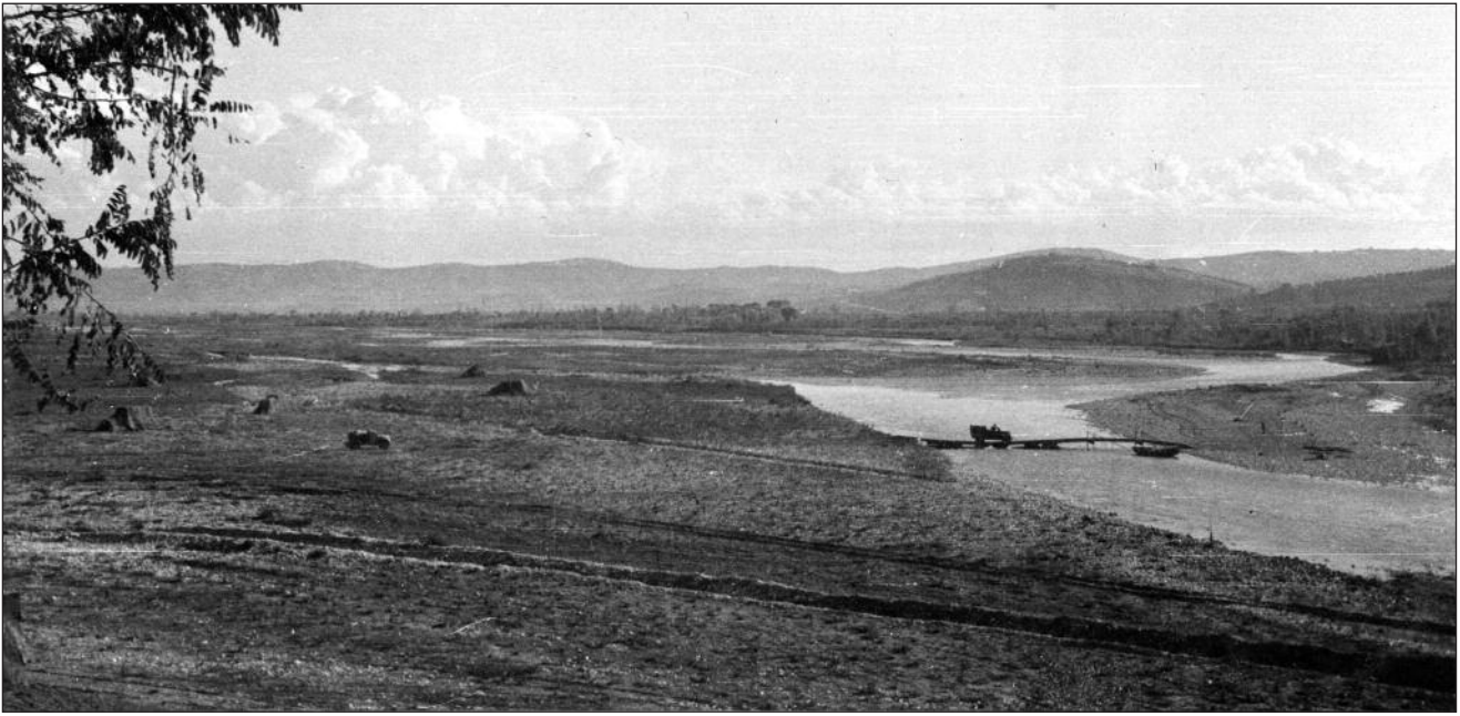
Lobe Bridge, an FBE folding-boat bridge built by the 6th NZ Field Company in the 6th Brigade sector, was located three kilometres south and upstream of Heartbeat. The first attempt to push it over the Sangro ended when it received a direct hit
