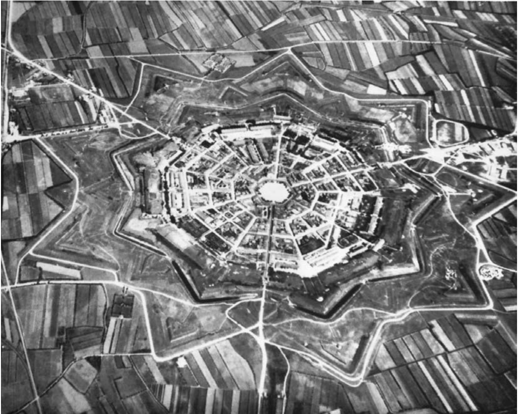
15.6. Vincenzo Scamozzi (attrib.), Palmanuova, Italy, begun 1593. Palmanuova was a new town, built according to the ideal circular model. Photo: Aerofilms, London.
