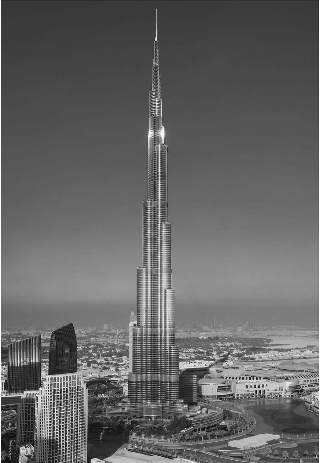
20.30. Skidmore, Owings & Merrill, Burj Khalifa, Dubai, United Arab Emirates, 2003–2010. For the moment the tallest building in the world, the tower has a series of setbacks at its base to provide a broader footprint. © Jose Fuste Raga/Corbis.
