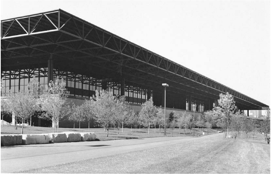
3.33. C. F. Murphy and Associates, McCormick Place, Chicago, Illinois, 1970–1971. Designed by Gene Summers, this space frame has spans of 150 feet (45.7 m) in both directions and covers a total area of 19 acres. Photo: Courtesy, Murphy-Jahn.
