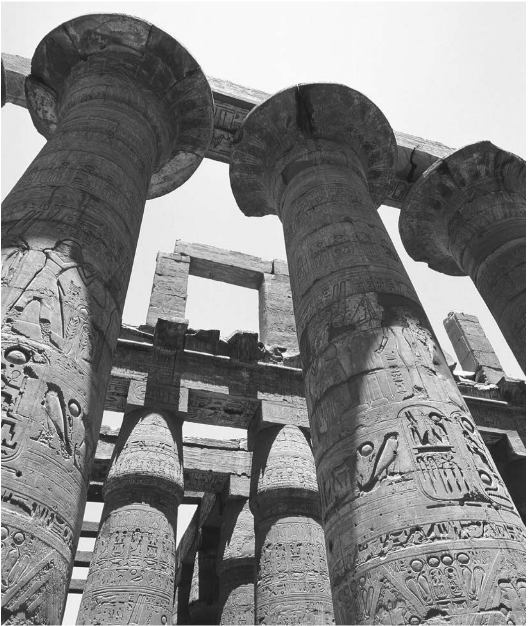
10.22. Hypostyle Hall, Temple of Amon, Karnak, Thebes, Egypt, c. 1315–1235 BCE. The huge columns along the central axis are 11.75 feet (3.6 m) in diameter and rise 69 feet (21 m); the axis they define is aligned to the rising sun at midwinter, pointing directly to the Valley of the Kings on the west side of the Nile. Photo: Gianni Dagli Orti/The Art Archive at Art Resource, NY.
