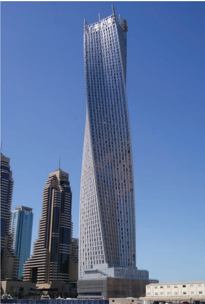
Plate 37. Santiago Calatrava, Infinity Tower, Dubai, United Arab Emirates, 2005–2012. By gently turning the square plan by increments, floor by floor, Calatrava creates a dynamic architectural form. Photo courtesy of Laticrete, www.laticrete.com .
