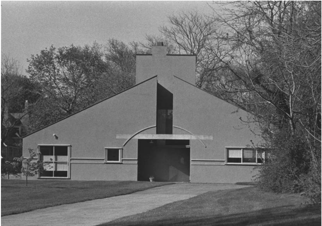
20.2. Venturi and Rauch with Cope and Lippincott, Vanna Venturi house, Chestnut Hill, Philadelphia, Pennsylvania, 1959–1964. In the early 1960s, when the minimalism of International Modernism was still dominant, Venturi composed a modest house for his mother that incorporated in abstracted form a classical pediment, articulated by decorative moldings. Photo: Courtesy of Venturi, Scott Brown, and Associates.
