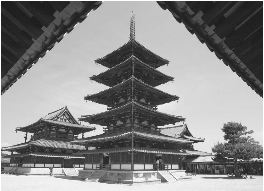
JP-1. Pagoda, Hōryū-ji Monastery, Hōryū-ji, Japan, c. 607. Inspired by Chinese pagodas, the Japanese pagoda tends to have far more extended, cantilevered roofs encircling the central shaft. This is the oldest wood pagoda in Japan. Photo: © Ivan Vdovin/Alamy.
