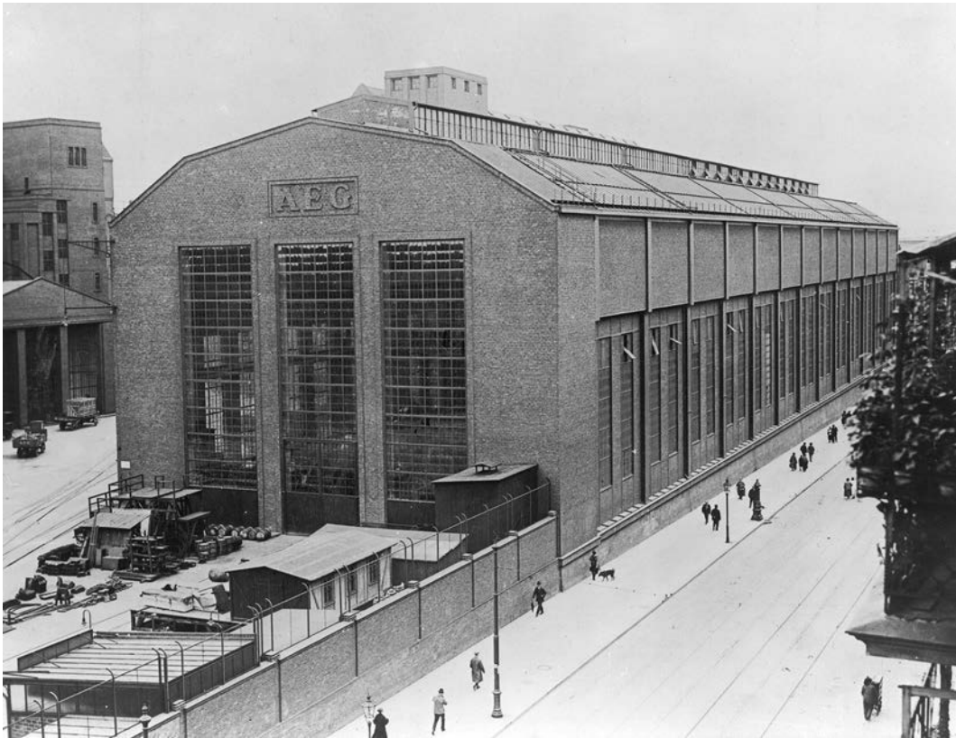
19.15. Peter Behrens, AEG Large Assembly Building, Berlin, Germany, 1911–1912. As in his Turbine Factory for the AEG [2.1], in this even larger assembly building Behrens offered another archetype of industrially based architecture elevated to the status of high-art architecture. Photo: bpk, Berlin/Art Resource, NY.
