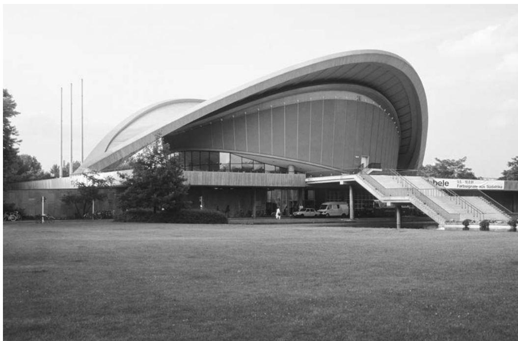
6.18. Hugh Stubbins, House of World Cultures (originally built as the West Berlin Congress Hall), Berlin, Germany, 1957; roof collapsed 1980; rebuilt. Constructed as a gift to Berlin from the US government. The roof collapsed in 1980 due to water infiltration, which caused corrosion of the steel cables supporting the concrete panels suspended between the arched edge beams. Photo: Vanni/Art Resource, NY.
