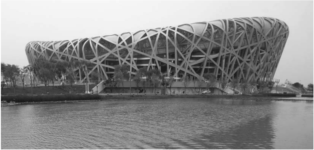
21.1. Herzog & de Meuron with artist/designer Ai Weiwei, Olympic National Stadium, Beijing, China, 2001–2008. Affectionately dubbed “The Bird’s Nest” because of its interwoven strands, this and other dramatic buildings were commissioned to make a dramatic public announcement of China’s arrival as a major player on the world’s architectural stage, signified also by China’s serving as host of the 2008 Olympic games. Photo: REUTERS/Alwin Chan.
