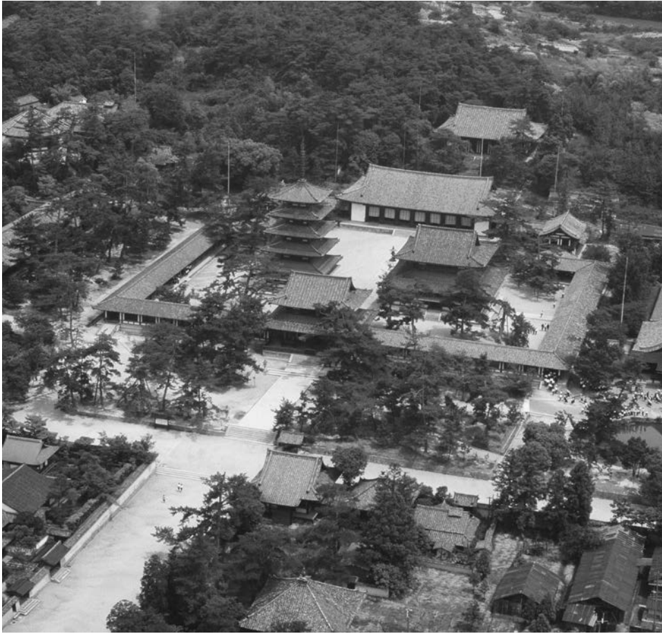
JP-3. Hōryū-ji temple complex, Hōryū-ji, Nara Prefecture, Japan, begun c. 607. This aerial view shows the contrast with Chinese Buddhist temple compounds, for the Japanese tend to avoid straight-line axial symmetry; here the axis runs between the five-story Gojū-no-Tō pagoda and the Kondō or Main Hall toward the Daikōdō or Great Lecture Hall on the north perimeter. Photo: © amana images inc./Alamy.
