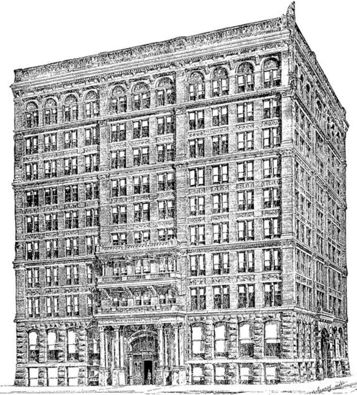
18.43. William Le Baron Jenney, Home Insurance Office Building, Chicago, Illinois, 1883–1886 (demolished 1931). When a bricklayers' strike interrupted progress in construction, Jenney substituted a full metal structural skeleton to allow work to continue; later, the outer masonry veneer was attached to the standing skeleton. This was the first constructed metal frame skyscraper. From A. T. Andreas, History of Chicago (Chicago, 1884–1886).
