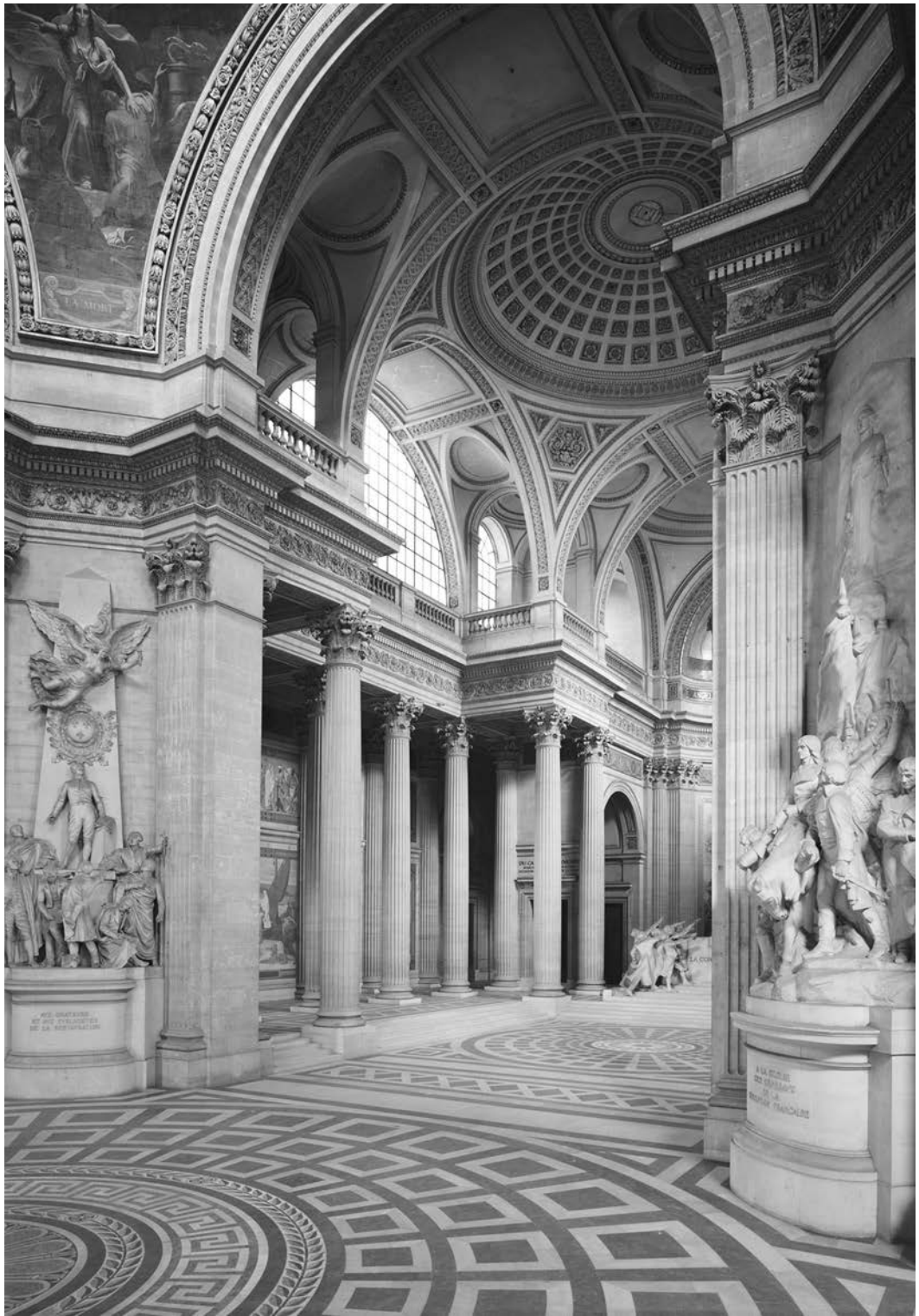
17.6. Jacques-Germain Soufflot, Church of Sainte-Geneviève ("Le Panthéon"), Paris, France, 1755–1790. Interior. The vaults are true structural shells of cut stone, not plaster illusions; their weight is poised directly over the structural Corinthian columns. Photo: Bridgeman-Giraudon/Art Resource, NY.
