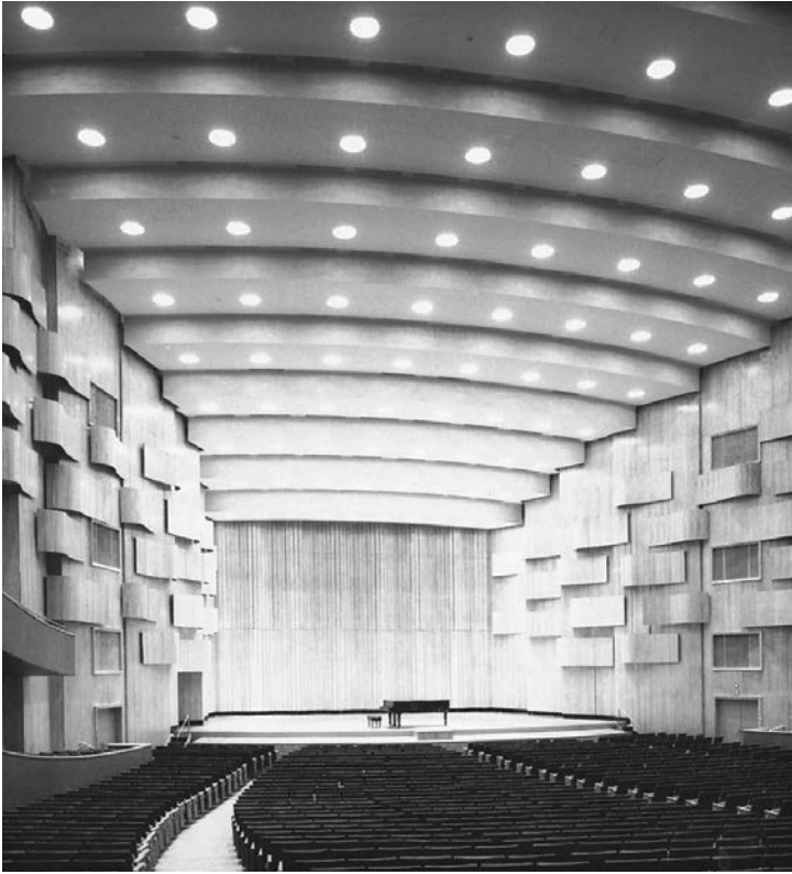
4.32. Harrison and Abramovitz, Philharmonic Hall, New York, NY, 1960–1962. The original interior shows the suspended “acoustical clouds” intended to disperse sound. Photo: ©1976 Lincoln Center for the Performing Arts, New York, by Norman McGrath.
