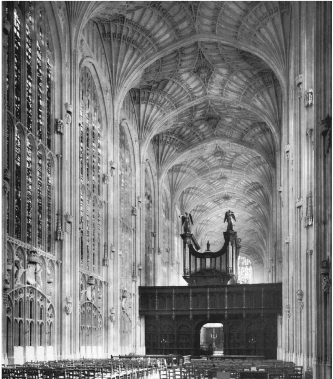
14.49. Reginald Ely and John Wastell, King's College Chapel, Cambridge University, Cambridge, England, 1446–1515. Interior. Unique to England was the fan vault, as found in King's College Chapel, suggesting a grove of trees. Photo: A. F. Kersting, London.
