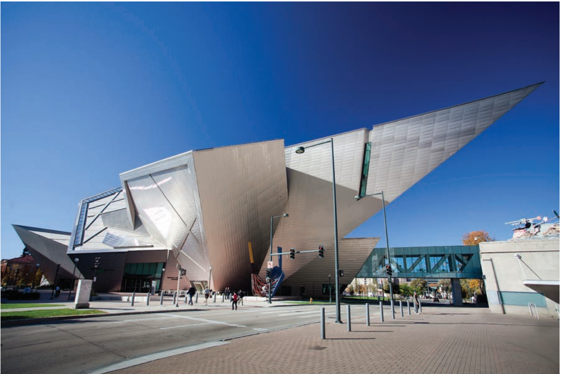
Plate 45. Daniel Libeskind, Hamilton Building addition, Denver Art Museum, Denver, CO, 2002–2006. Capitalizing on the sharply angular aggressiveness of Postmodernism, Libeskind has created a building that presents itself as a forceful work of art. Photo: © Prisma Bildagentur AG/Alamy.
