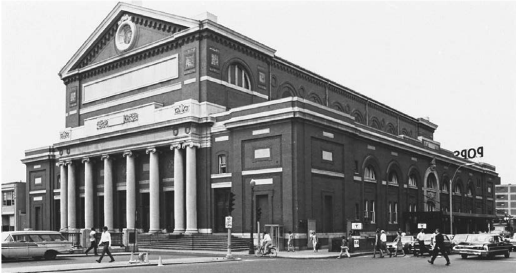
5.14. McKim, Mead & White, Boston Symphony Hall, Boston, Massachusetts, 1892–1900. Exterior. Although patterned after the Musikvereinsgebäude in Vienna and the Gewandhaus in Leipzig, this design was modified in accordance with acoustical calculations made by the engineer Wallace Sabine, making this the first building acoustically and scientifically planned to be a symphonic hall. Photo: L. M. Roth.
