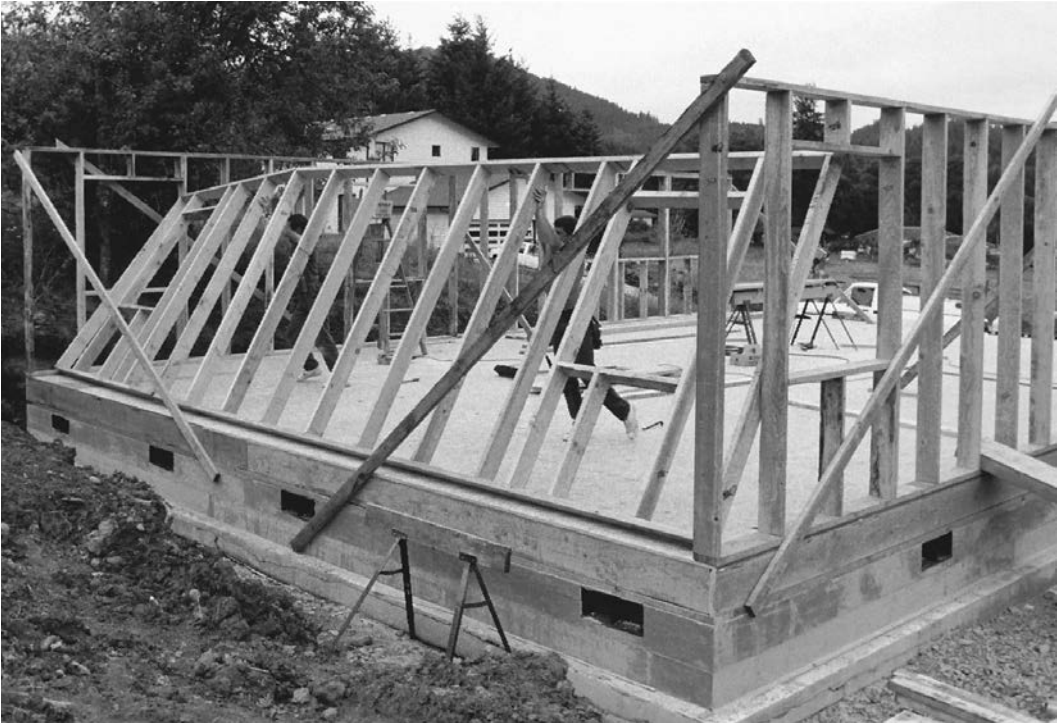
3.19. Balloon frame. Photo: L. M. Roth.
