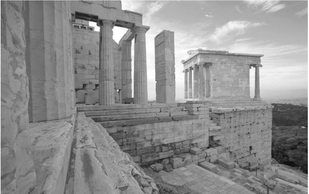
11.20. Temple of Athena Nike, Akropolis, Athens, Greece, c. 435–420 BCE. This tiny jewel was built to commemorate the Greek victory over the Persians in 449 BCE; it stands over an ancient Bronze Age defensive bastion protecting the gate to the Akropolis. It has Ionic columns only at the front and rear. Photo: NGS Image Collection/The Art Archive at Art Resource, NY.
