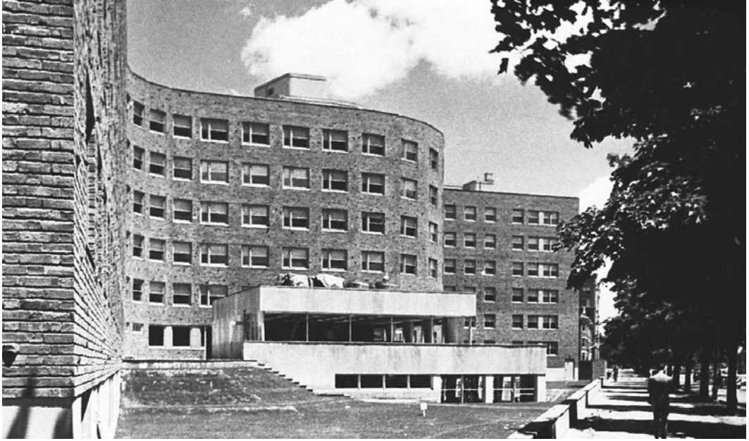
4.21. Alvar Aalto, Baker House, Massachusetts Institute of Technology, Cambridge, Massachusetts. Viewed at close range, the randomly placed and protruding rough bricks create a visual and tactile texture in the wall. Photo: C. Condit Collection, Department of Art History, Northwestern University.
