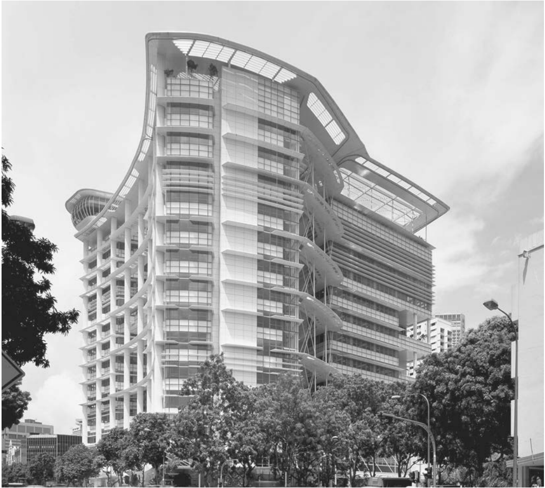
21.6. Ken Yeang, Singapore National Library, Singapore, 1998–2005. In a graceful form for this tropical high-rise, Yeang incorporates varied projecting floor ledges and fins, as well as open spaces, to reduce heat gain and allow wind to circulate through portions of the building. Photo: Courtesy of Ken Yeang.
