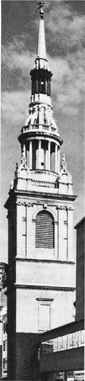
16.31. Sir Christopher Wren, Church of Saint Mary-le-Bow, London, England, 1670–1680. In re-creating the image of tall Gothic spires in the new City churches, Wren used stacked diminishing Classical elements. Photo: A. F. Kersting.
