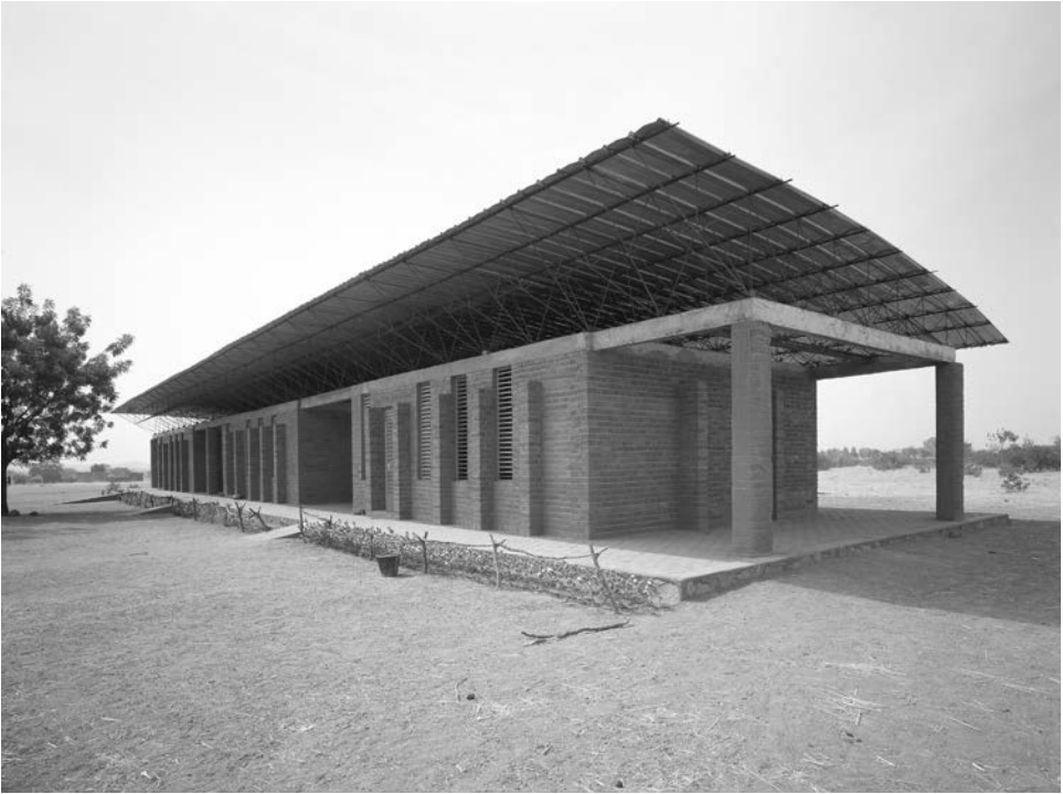
AF-5. Diébédo Francis Kéré, Primary School, Gando, Burkina Faso, Africa, 2004. Drawing on inexpensive modern materials (galvanized sheet metal) and traditionally based materials (hand-molded adobe brick), Kéré designed this school to be built largely using village workers. Photo: © Siméon Douchoud of the Aga Khan Award for Architecture.
