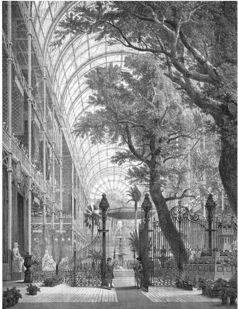
18.21. Crystal Palace. Interior view of the central transept, May Day 1851, showing how the building incorporated entire ancient trees already existing on the building site in Hyde Park. From: B. Dunlop and D. Hector, eds., Lost Masterpieces (London, 1999).
