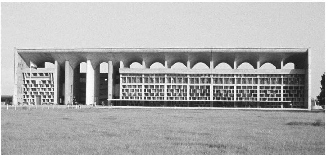
6.11. Le Corbusier, High Court Building, Chandigarh, Punjab, India, 1951–1956. In this semitropical climate, Le Corbusier used the traditional Indian parasol concept to keep the sun off the roof of the building. The double roof is raised so that breezes can carry away any heat buildup. Photo: John E. Tompkins, 1965, Visual Resources Collection, Architecture & Allied Arts Library, University of Oregon.
