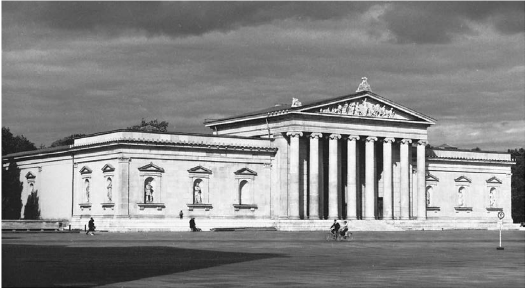
18.1. Leo von Klenze, Glyptothek (Sculpture Gallery) , Munich, Germany, 1816–1830. Designed as part of the campaign to embellish Munich as capital of Bavaria, this public museum was designed by von Klenze especially to house the Greek sculpture recently discovered at the Temple of Aphaia on the island of Aegina, Greece. Photo: © Wayne Andrews/Esto. All rights reserved.
