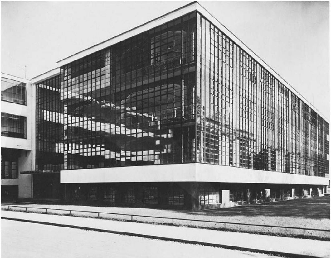
19.18. Workshop wing, Bauhaus, Dessau. In the workshop wing, particularly, Gropius succeeded in suggesting a weightless, transparent architecture; the wall, entirely of glass, is hung away from the supporting structure. Photo: Courtesy, Museum of Modern Art, New York.
