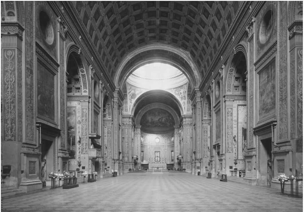
15.21. Sant' Andrea. Interior. The nave is covered by a massive brick barrel vault with deep coffers, recalling Roman baths. Photo: Scala/Art Resource, NY.
