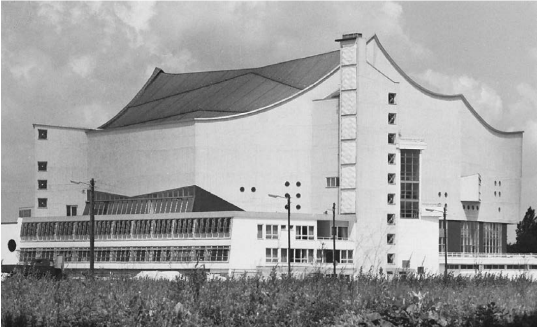
19.48. Hans Scharoun, Berlin Philharmonie, Berlin, Germany, 1957–1965. Exterior. The unusual plan and profile of this building were shaped by the desire to put music at the center of the audience. Photo: German Information Center, New York.
