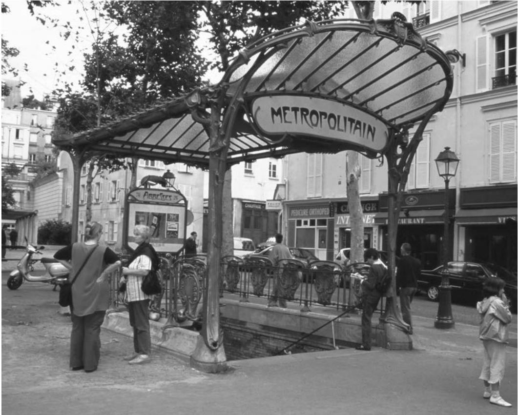
19.5. Hector Guimard, Metro Station (Les Abbesses stop) in Montmartre, Paris, France, 1900–1913. Using forms inspired by plants, Guimard devised a system of identical cast iron and ceramic parts to create entry gates for the new electrically powered underground mass-transit system. Photo: L. M. Roth, 2003.
