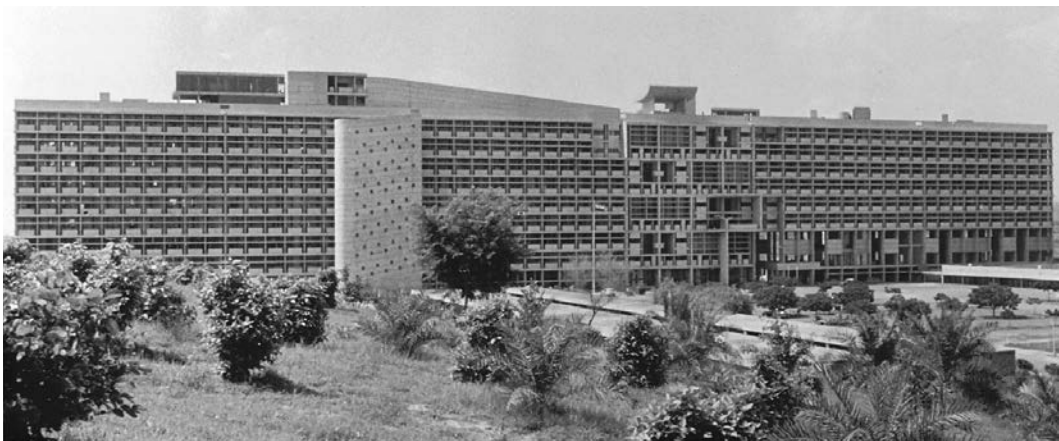
4.20. Le Corbusier, Secretariat Building, Chandigarh, India, 1951–1958. In this elongated building, Le Corbusier varied the rhythm of the shape and sizes of the sun screens, breaking up the long facade, and indicating office cells contrasted to committee rooms. Photo: John E. Tomkins, courtesy of the Visual Resource Collection, Architecture & Allied Arts Library, University of Oregon.
