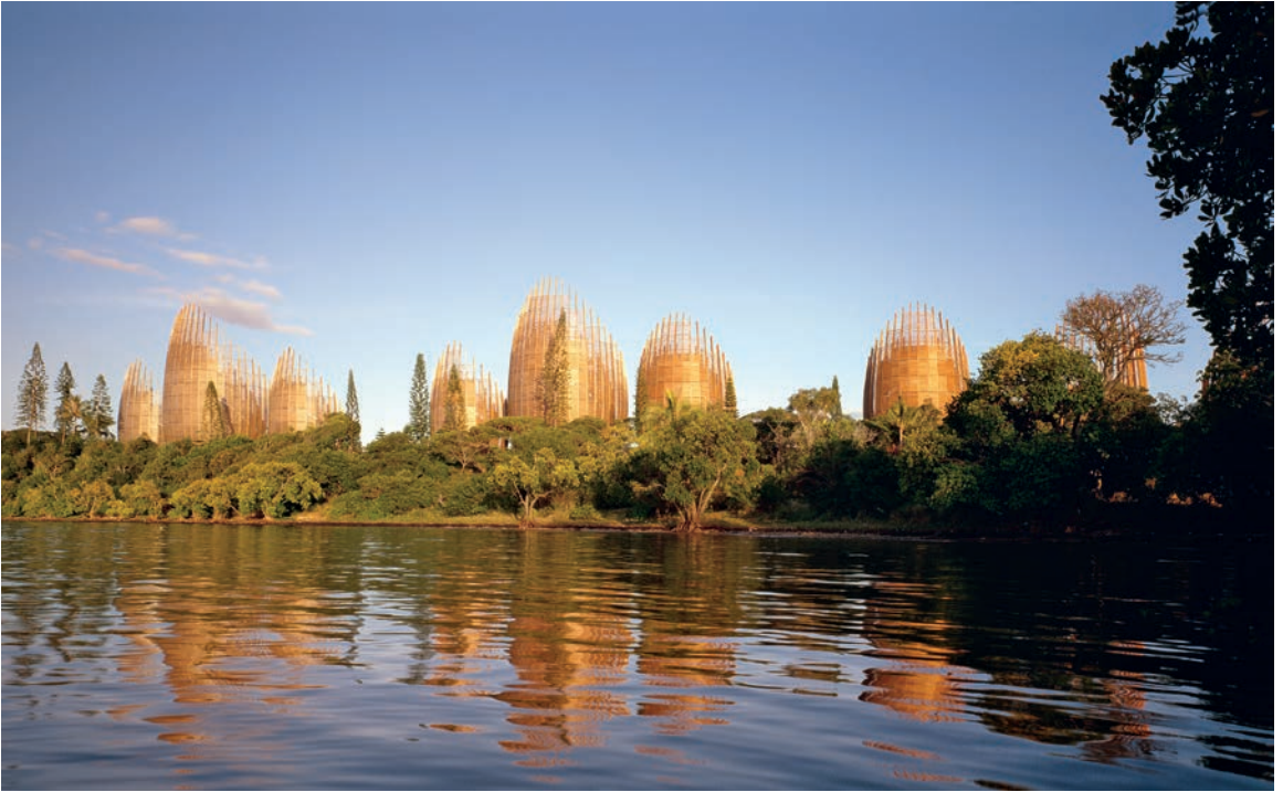
Plate 44. Renzo Piano, Tjibaou Cultural Center, New Caledonia, 1992–1998. Piano's complex of low exhibition rooms and towering "great houses" merges with a landscape carefully designed to highlight indigenous plants. Photo: © John Golling, courtesy of Renzo Piano Building Workshop.
