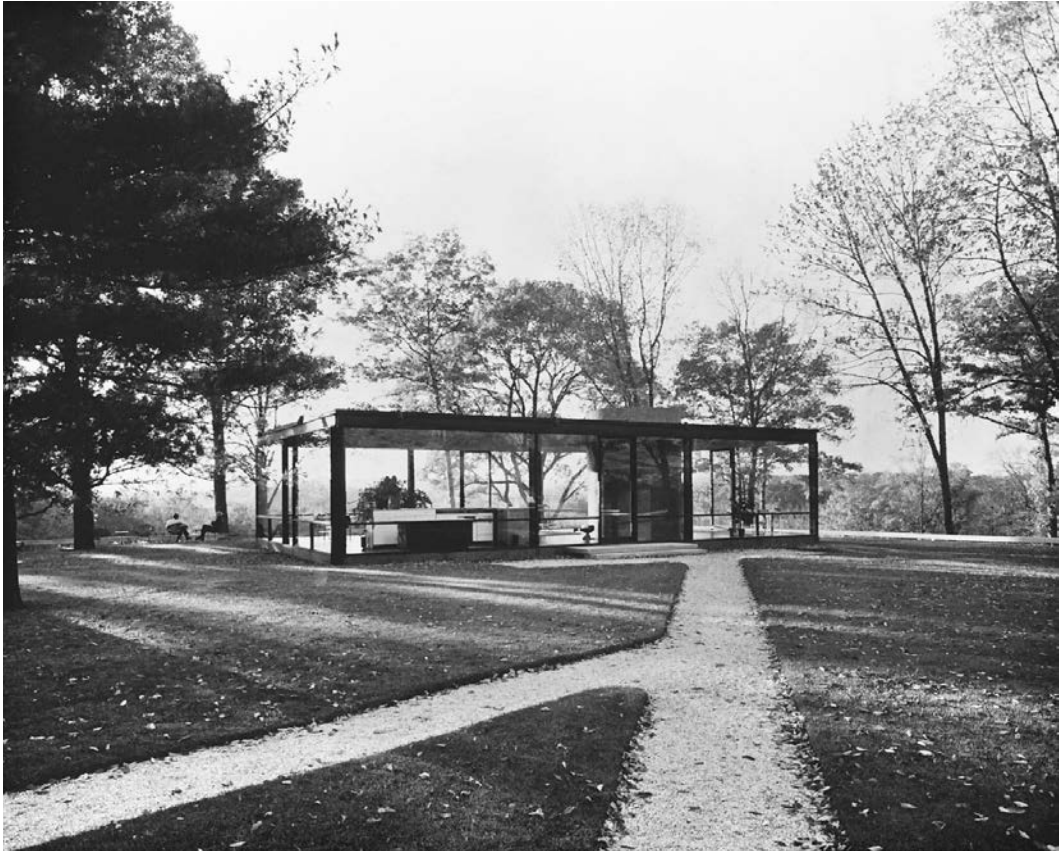
6.15. Philip Johnson, Johnson House, New Canaan, Connecticut, 1945–1949. Although the house that Philip Johnson built for himself has walls entirely of glass, it is shaded and cooled in the summer by trees to the west, but then warmed in the winter when sunlight filters through the bare branches. Photo: Alexandre Georges, courtesy of Philip Johnson.
