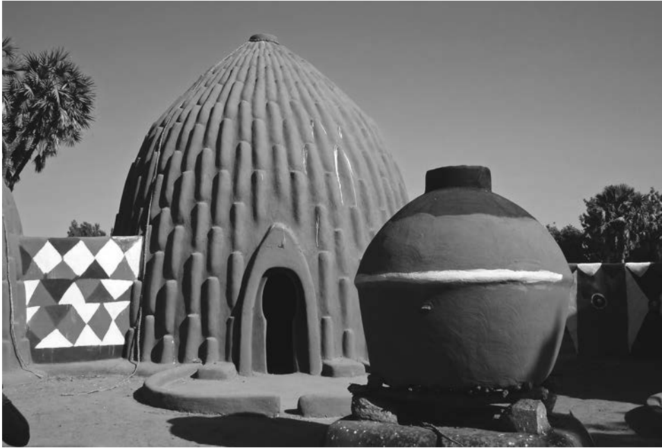
AF-2. Musgum house, in Cameroon, Africa, late twentieth century. Over a light sapling frame, layers of a clay-adobe are applied forming slightly projecting oval forms; once dried, these forms serve as foot rests for those applying the upper layers of the adobe shell until the top is reached. These houses can reach heights of over 35 feet (30.7 m). Photo: © Anthony Asael/Art in All of Us/Corbis.
