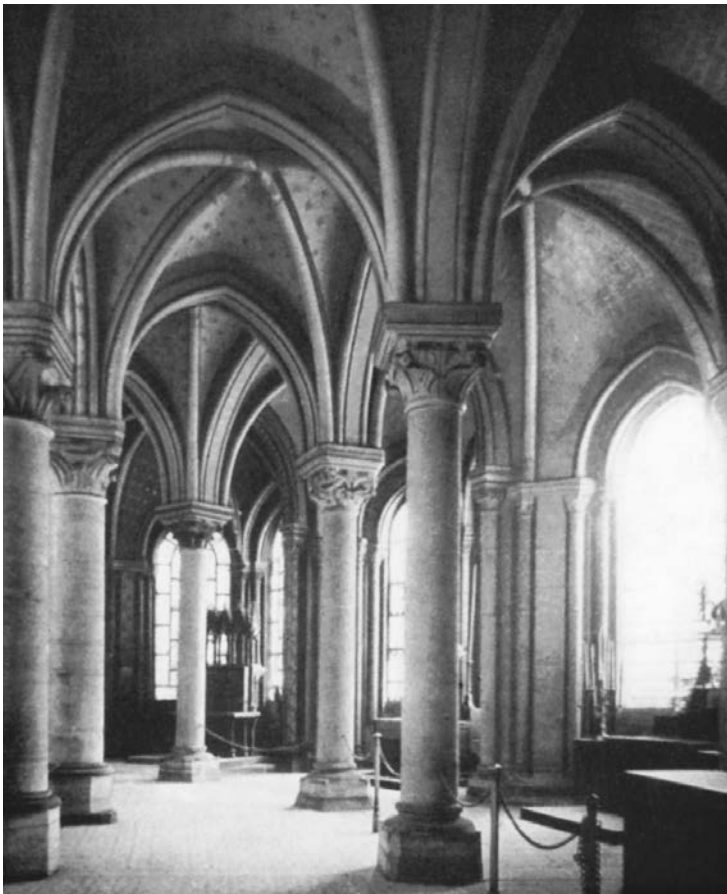
14.33. Saint-Denis. Interior of the choir ambulatory. By combining rib vaults and pointed arches with careful resolution of structural forces, Suger's architects were able to achieve unprecedented lightness of structure and to open the walls to large panes of stained glass. Photo: University of Munich, Kunstgeschichtliches Seminar.
