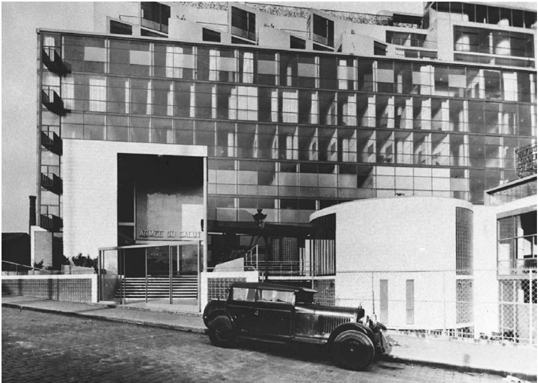
6.10. Le Corbusier, Cité de Refuge (Salvation Army Hostel), Paris, France, 1929–1933. Like the Robie House, Le Corbusier's Salvation Army Hostel was orientated east-west, its broad southern glass front exposed to the sun. The heat buildup was to be countered by double glazing and an air-conditioning system, but these were not installed, necessitating the later retro-installation projecting sun screens. Photo: C. Condit Collection, Department of Art History, Northwestern University.
