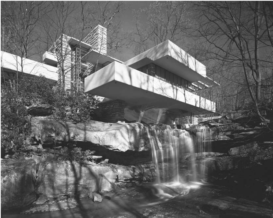
4.24. Frank Lloyd Wright, Edgar Kaufmann residence, Fallingwater, near Mill Run, Pennsylvania, 1936–1938. Wright created strong contrasts between the rough vertical masonry piers (with stone slabs laid to imitate natural rock strata) and the smooth horizontal concrete floor slab upstands. Photo by Hedrich Blessing. Chicago History Museum, negative HB-04414-5d.
