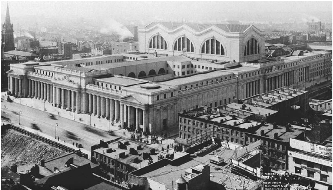
18.46. McKim, Mead & White, Pennsylvania Station, New York City, 1902–1910 (demolished 1963–1965). As had G. G. Scott in the St. Pancras Station in London, McKim, Mead & White wanted to celebrate the power of the railroad and create a magisterial gateway for the city. Photo: Dreyer photo, c. 1909; courtesy of Avery Library, Columbia University.
