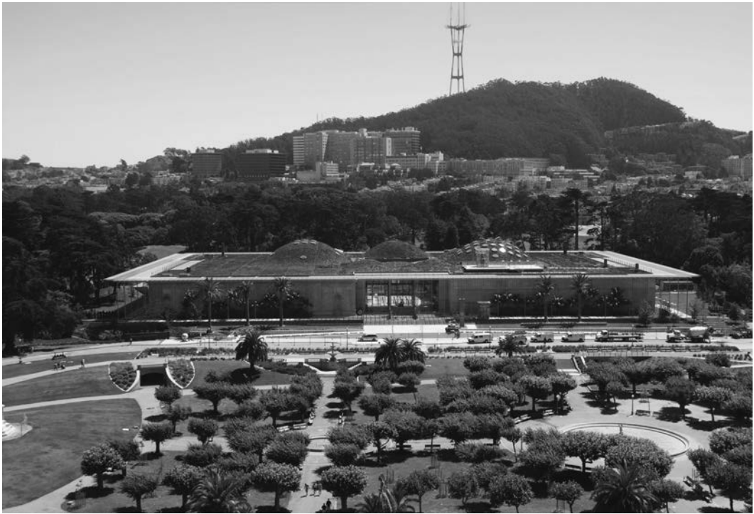
21.3. Renzo Piano, California Academy of Sciences , Golden Gate Park, San Francisco, California, 2005–2008. Covering the entire roof with gently undulating roof gardens, Piano and his associates created a landscape that mediates between the park and nearby hills. Photo: © Lee Foster/Alamy.
