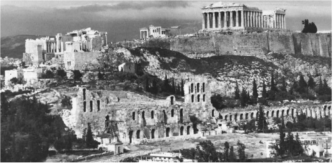
11.7. Akropolis, Athens, Greece, viewed from the west. Photo: Hirmer Fotoarchiv, Munich.
