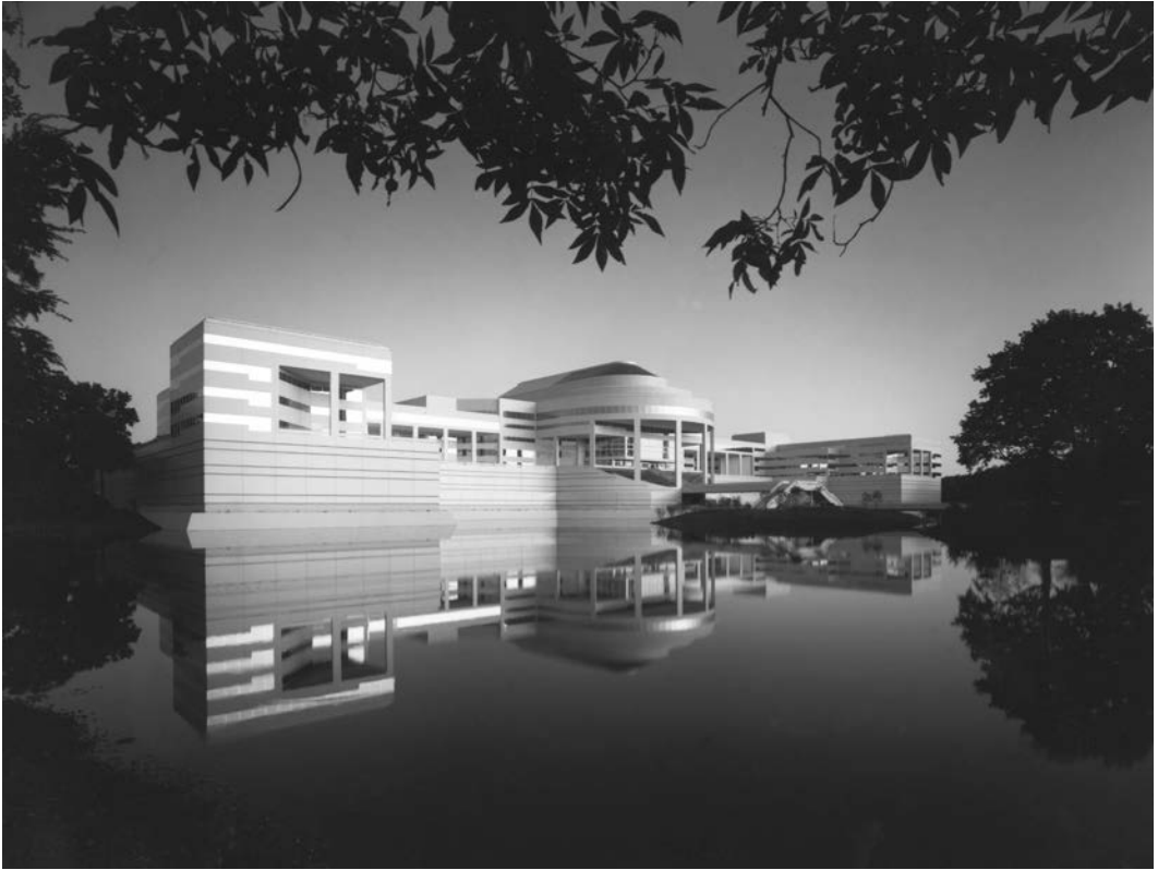
20.8. Kevin Roche, General Foods Headquarters , Rye, New York, 1977–1983. Latent Classicism incorporates a fundamental order, often based on bilateral symmetry, but couched in a language of modern building technology. Photo: Courtesy of Kevin Roche.
