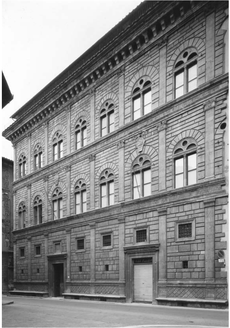
15.29. Leon Battista Alberti, Palazzo Rucellai , Florence, Italy, begun c. 1452. Alberti based his facade (actually a remodeling of existing houses) on Roman sources, using superimposed pilasters to create a varied rhythm and to visually support the crowning cornice. Photo: Scala/Art Resource, NY.
