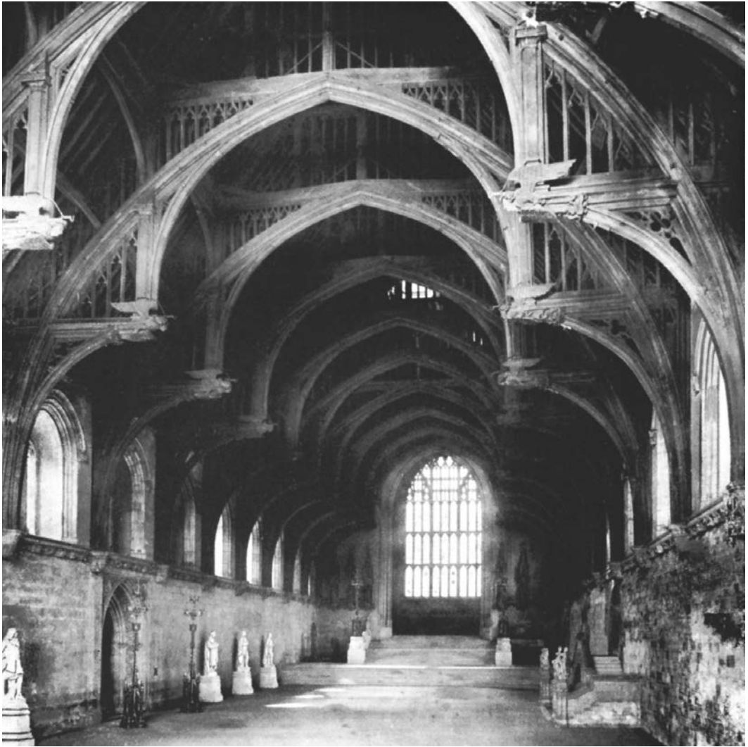
14.46. Henry Yevele and Hugh Herland, Westminster Hall, Palace of Westminster, London, England, 1394. Interior. Spanning 68 feet (20.7 m), this is one of the largest surviving medieval wooden roof trusses. Photo: Country Life, London.
