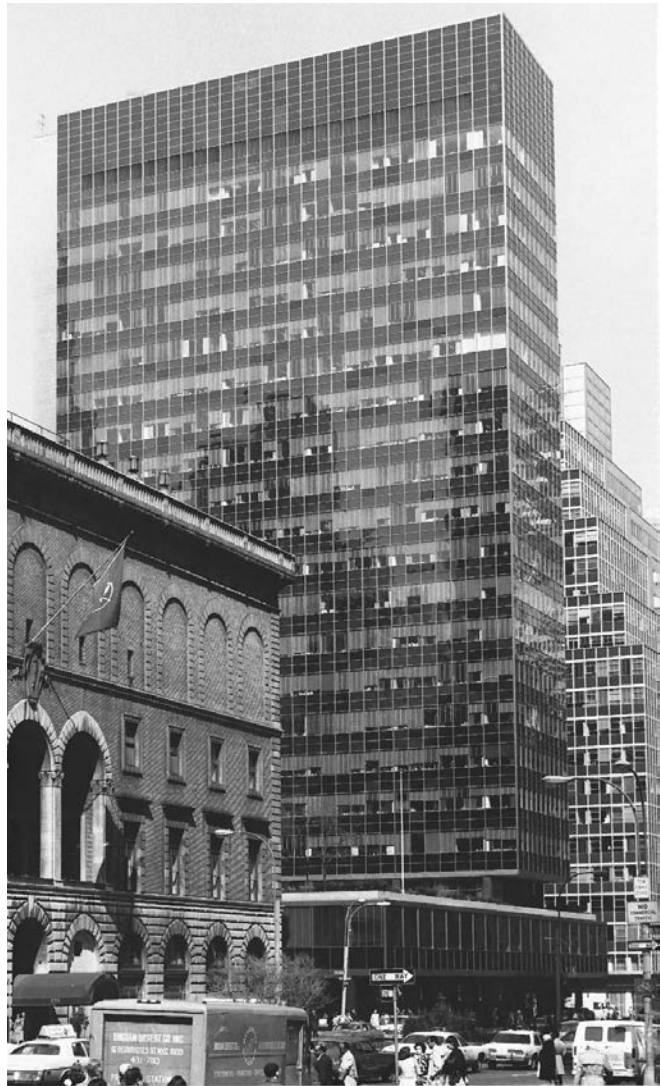
3.2. Skidmore, Owings & Merrill, Lever House, New York, 1951–1952. With its glass envelope suspended from the inner skeleton, Lever House visually hides its structure, whereas the adjacent New York Racquet and Tennis Club (by McKim, Mead & White, 1916–1919) has a boldly expressed wall structure. Photo: L. M. Roth.
