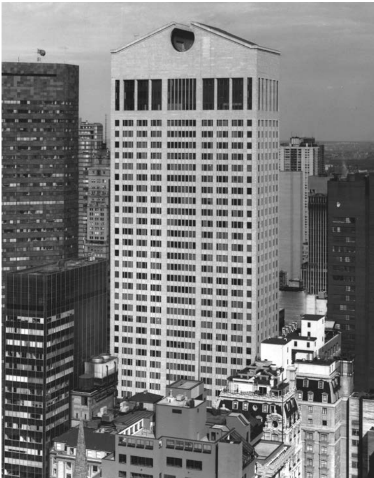
20.5. Philip Johnson, AT&T Building, New York, NY, 1978–1983. In this corporate headquarters building, Johnson used bold ornament and pattern, recalling similar New York skyscrapers of the 1920s. Photo: Richard Payne.
