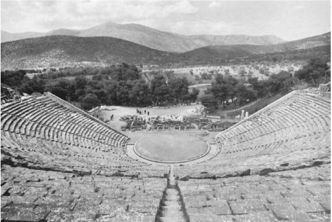
11.15. Polykleitos the Younger, Theater, Epidauros, Greece, c. 350 BCE. Elevated view. Typically, Greek theaters adjoined religious sites and were built into hillsides. The seats here extend around 200° and looked down onto low, temporary skēnē structures. Photo: Hirmer Fotoarchiv, Munich.
