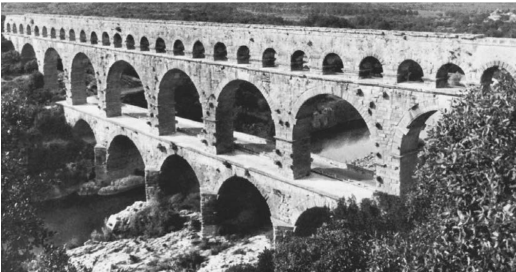
3.23. Pont du Gard Nîmes, France, 25 BCE. A combination bridge and aqueduct with superimposed arches. Photo: Touring Club de France, Paris.
