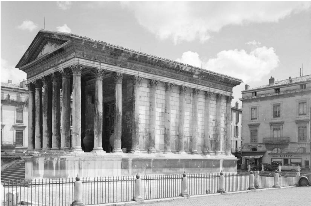
12.2. Maison Carrée , Nîmes, France (the Roman city of Nemausus, Gaul), begun c. 19 BCE. One of the best preserved of all Roman temples, this shows the high base, emphatic front, and engaged columns in the side walls typical of Roman temples. Photo: © Wayne Andrews/Esto. All rights reserved.
