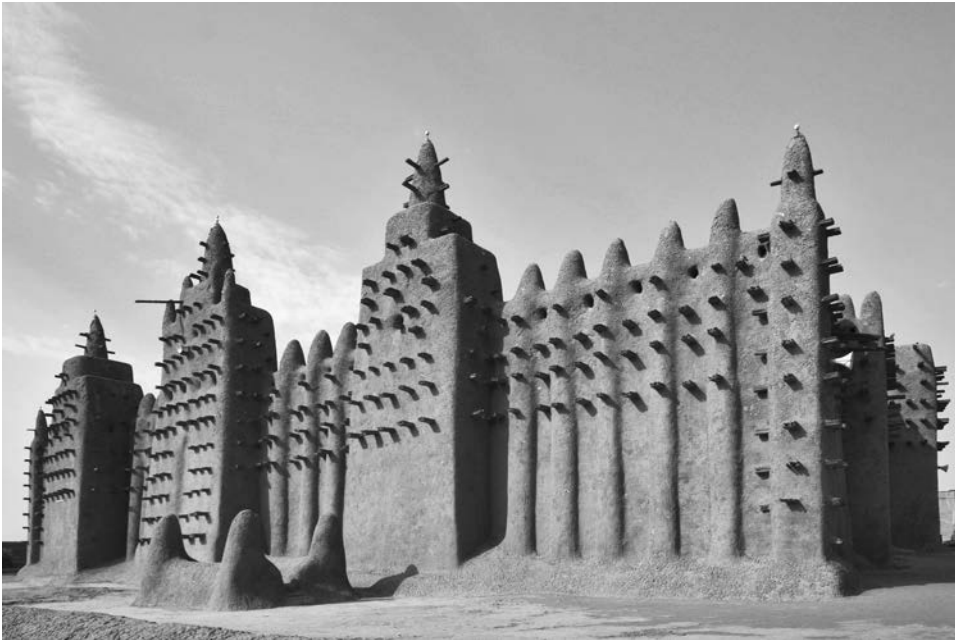
AF-4. Djenné Mosque, Djenné, Mali, Africa, 1906–1907. Though rebuilt after extended neglect, the form and building material continue a centuries-old local tradition; the protecting bundles of rodier palm are used for periodic adobe plaster maintenance. Photo: AFP/Getty Images.
