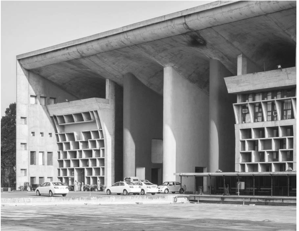
6.1. Le Corbusier, High Court Building, Chandigarh, Punjab, India, 1951–1956. Detail. Drawing from the idea of a parasol carried to protect dignitaries from the sun, Le Corbusier used an elevated roof over a roof to protect the rooms within from direct exposure to the sun, with broad openings for moving air to carry away built-up heat. Photo: Fernando Stankuns.
