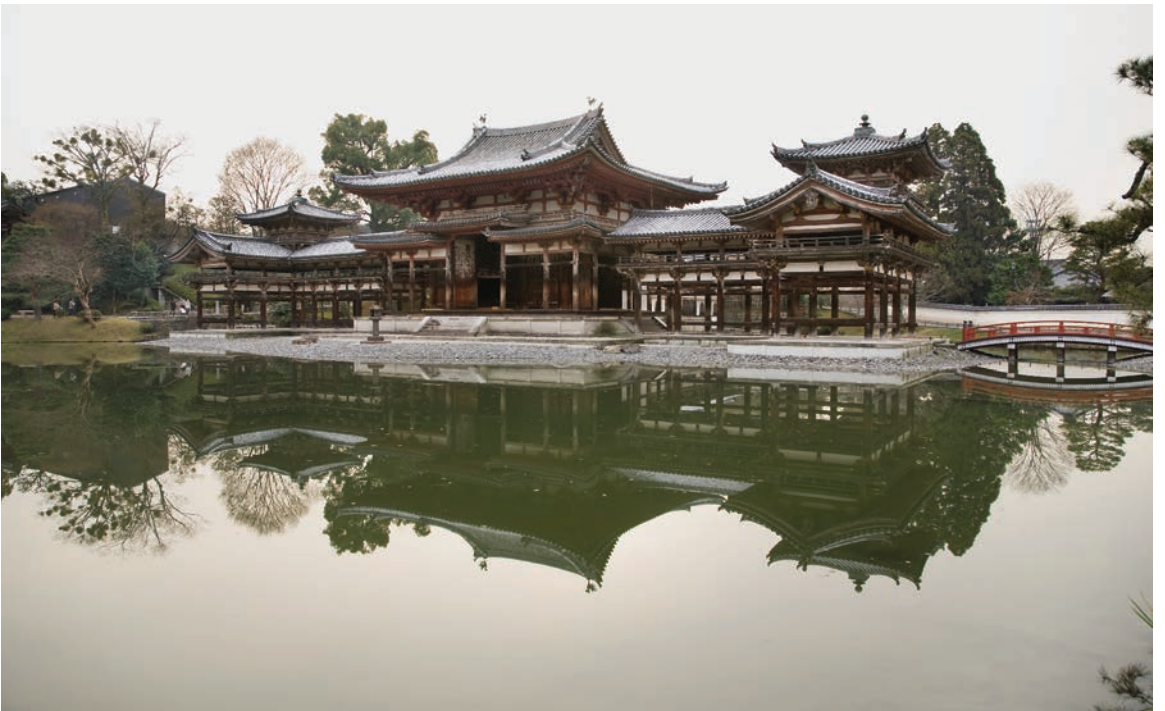
Plate 24. The Amida Hall (Hōōdō) or Phoenix Hall, Byōdōin, Uji, near Kyōto, Japan, 1053. The outstretched arms extending from the central hall are thought to symbolize the wings of the phoenix. Here the extended cantilevered beams, creating the lifting roofs, are evident. Photo: Vanni/Art Resource, NY.
