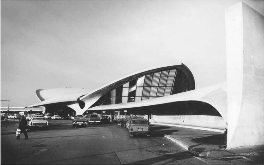
19.46. Eero Saarinen, Trans World Airlines Terminal, John F. Kennedy Airport, New York, NY, 1956–1962. With its soaring cantilevered concrete wings, Saarinen endeavored to shape in the TWA Terminal a symbolic representation of flight. Photo: L. M. Roth.
