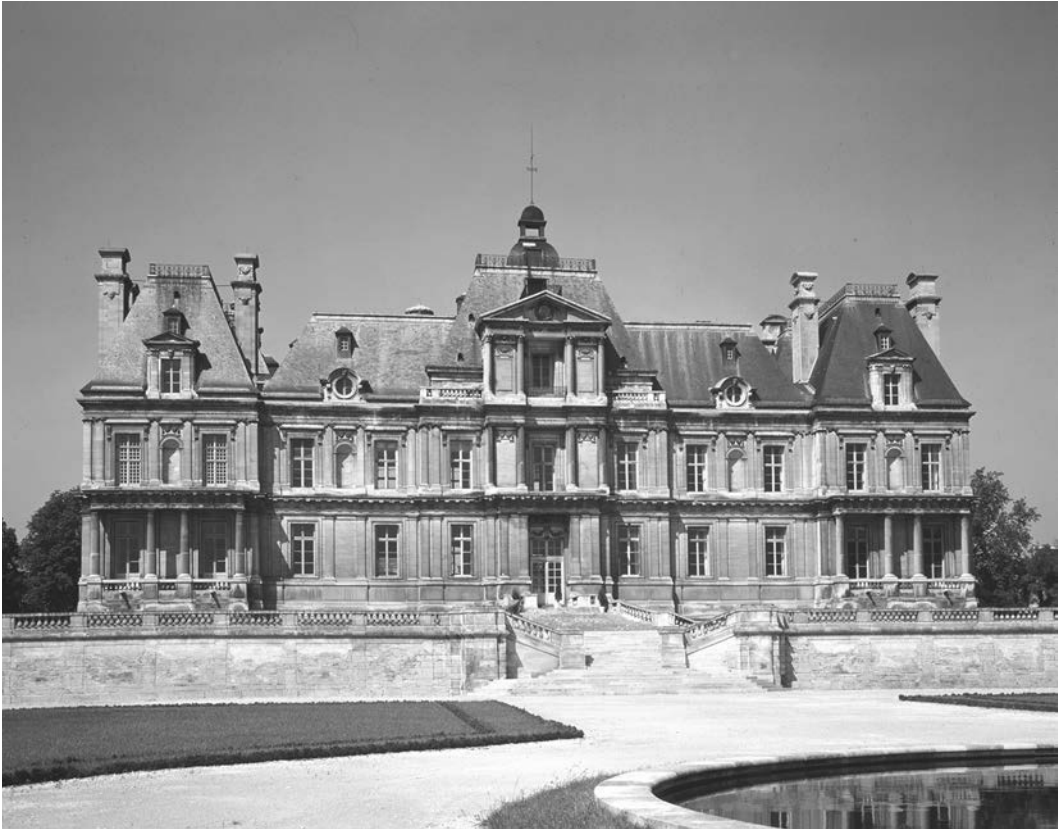
15.50. François Mansart, Château de Maisons , originally the village of Maisons, near Paris, France, 1642–1646. Although the forms have been clarified and the Classical details thoroughly mastered, the separation of pavilions and wall segments is continued, and the pavilions are capped by tall roofs that soon came to be called by the architect's name (spelled “mansard” in English). Photo: Bridgeman-Giraudon, Art Resource, New York.
