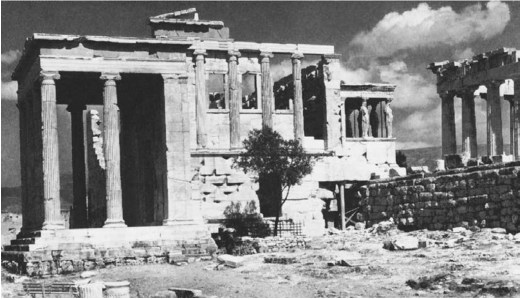
11.24. Erechtheion temple, Akropolis, Athens, Greece, 421–405 BCE. This complex building houses shrines to a variety of gods, including Athena Polias, protectress of the city. It sits astride a drop in the level of the rock, and hence has a split-level plan. It includes the Porch of the Maidens (Caryatids). Photo: A. Frantz.
