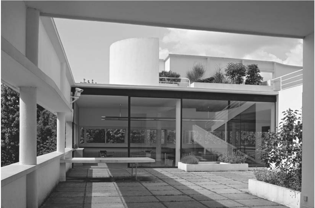
19.27. Villa Savoye. View of the outdoor living room, showing the ramp to the upper roof garden. Photo: © Jeff Goldberg/Esto.
