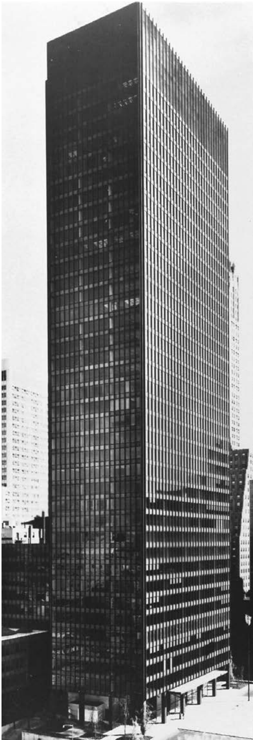
6.13. Ludwig Mies van der Rohe with Philip Johnson, Seagram Building, New York, NY, 1954–1958. This building is totally sealed, relying on an extensive heating and cooling system to regulate the temperature. Photo: Ezra Stoller © Esto.
