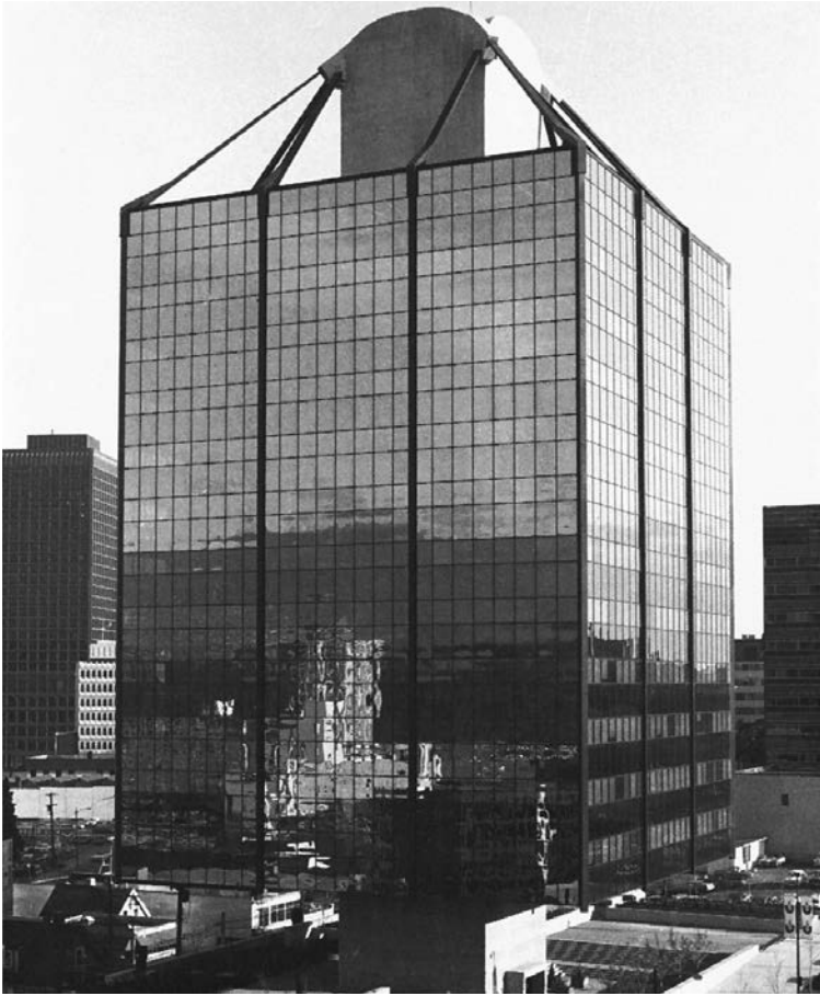
3.44. Rhone and Iredale, with Bogue and Babicki, engineers, Westcoast Transmission Building, Vancouver, British Columbia, Canada, 1968–1969. The floors are carried on beams and columns attached to exterior cables that angle back to the central structural mast. Photo: Jack Lindsay, Vancouver, Canada.
