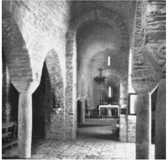
14.12. Saint-Martin-du-Canigou. Interior of upper church. Although perhaps conducive to meditation, the darkness of the interior shows the problem in creating openings in barrel vaults. Photo: Foto Mas.
