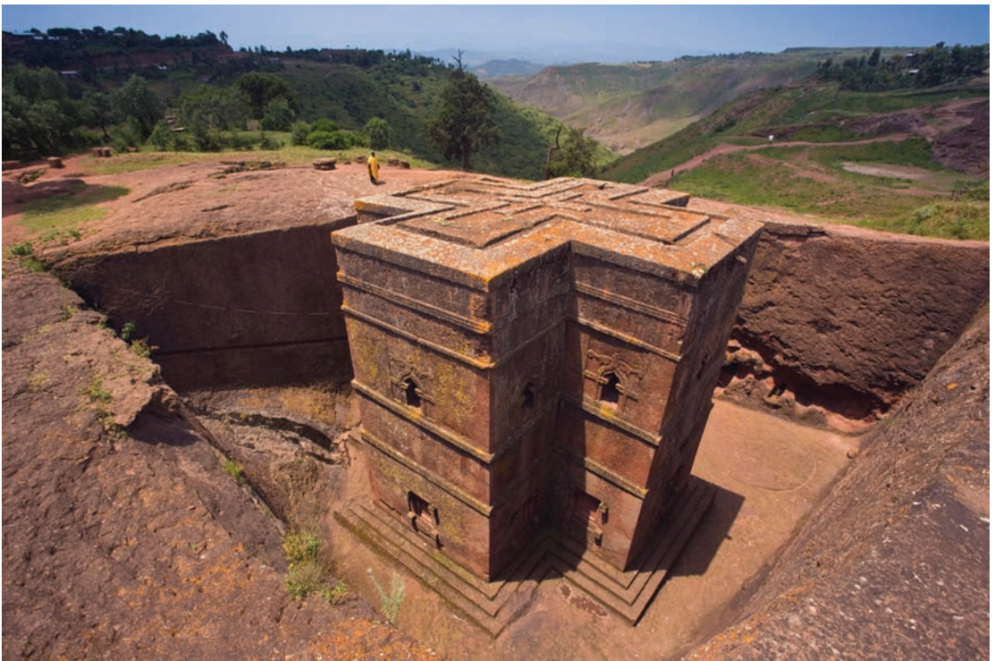
Plate 27. Church of St. George, Lalibela, Ethiopia, thirteenth century. One of the relatively rare examples of a building that was created by cutting away the surrounding rock, much as a sculptor cuts away a block of marble to reveal the figure residing “inside” the stone. Photo: © Robert Harding Picture Library Ltd/Alamy.
