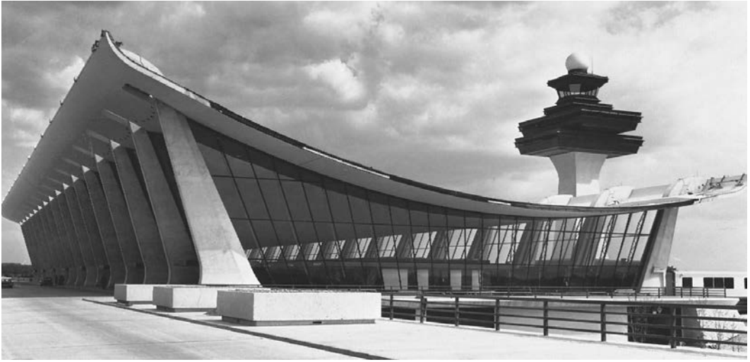
3.42. Eero Saarinen, Dulles International Airport Terminal, Washington, DC, 1958–1962. The roof is suspended on cables anchored in the beams running along each side of the building. Photo: © Wayne Andrews/Esto. All rights reserved.
