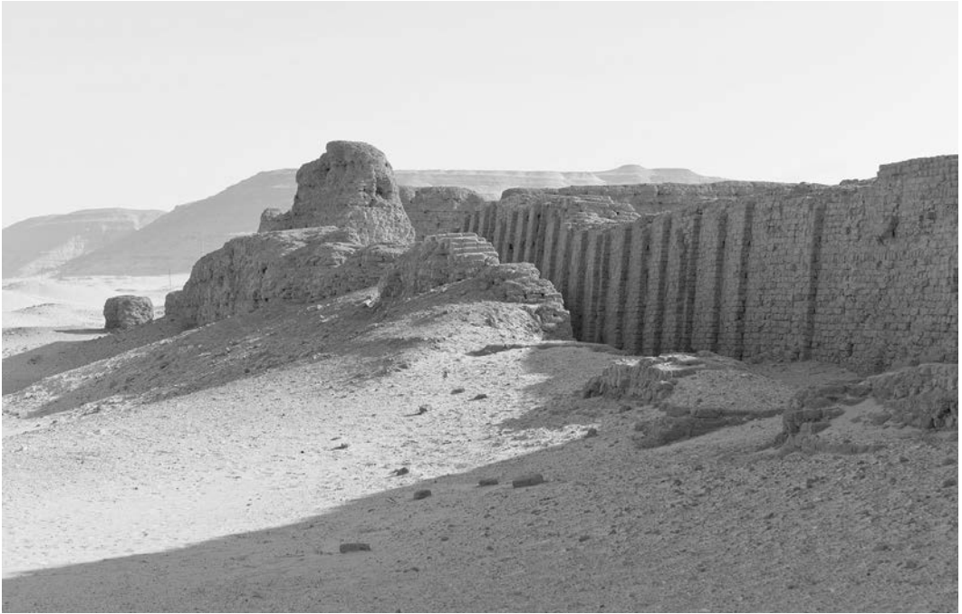
10.9. Palace of Khasekhemwy, Abydos, Egypt, c. 2780 BCE. This is one of the oldest ancient Egyptian buildings, now exposed with the sand removed; the ancient adobe brick walls are being given a new veneer of fresh adobe bricks as protection. Photo: © Mike P. Shepherd/Alamy.
