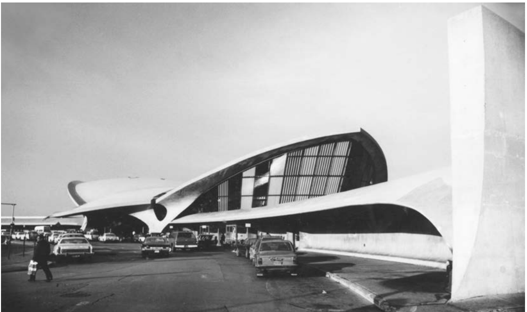
2.10. Eero Saarinen, Trans World Airlines Terminal, John F. Kennedy Airport, New York, NY, 1956–1962. With its soaring cantilevered concrete wings, Saarinen endeavored to shape in the TWA Terminal a symbolic representation of the magic of flight. Photo: L. M. Roth.
