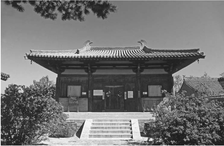
CH-3. Nanchan Buddhist Temple at Mt. Wutai, Shanxi Province, China, 782. The oldest wood temple in China, this shows the wood bracketing ( dougong ) construction that carried roofs cantilevered well beyond the walls. Photo: Christopher Liu, Chinastock.
