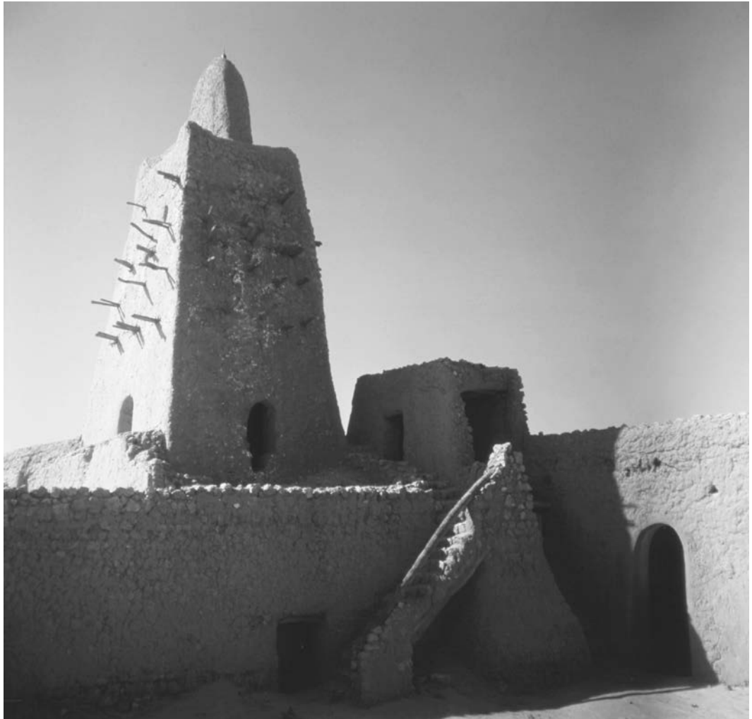
AF-1. Great Mosque at Timbuktu, Mali, Africa, fourteenth century. The oldest mosque south of the Sahara, built of rounded adobe bricks and stone rubble with a clay stucco finish. Photo: Werner Forman/Art Resource, NY.
