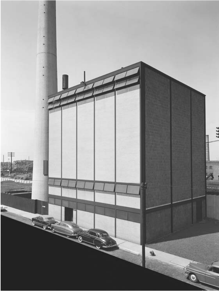
2.7. Mies van der Rohe, Boiler House, Illinois Institute of Technology, Chicago, Illinois, 1940. Heating plant building. With its tower-like chimney and high clerestory windows, this building has the physical attributes of early churches. Photo by Hedrich Blessing. Chicago History Museum, negative HB-12979B.
