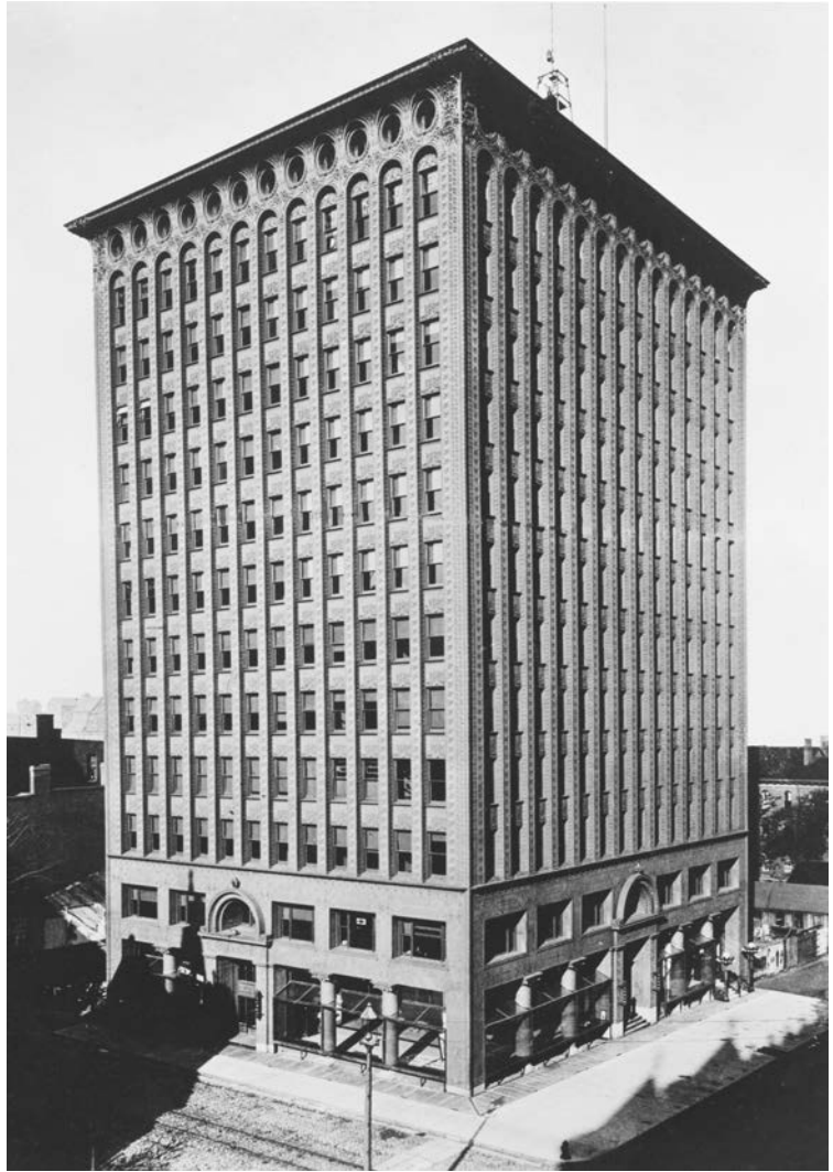
18.44. Adler & Sullivan, Guaranty Building, Buffalo, New York, 1895. Sullivan gave clear expression on the exterior of three major functional zones of the modern office skyscraper. Photo: Rosenthal Collection, Department of Art History, Northwestern University.
