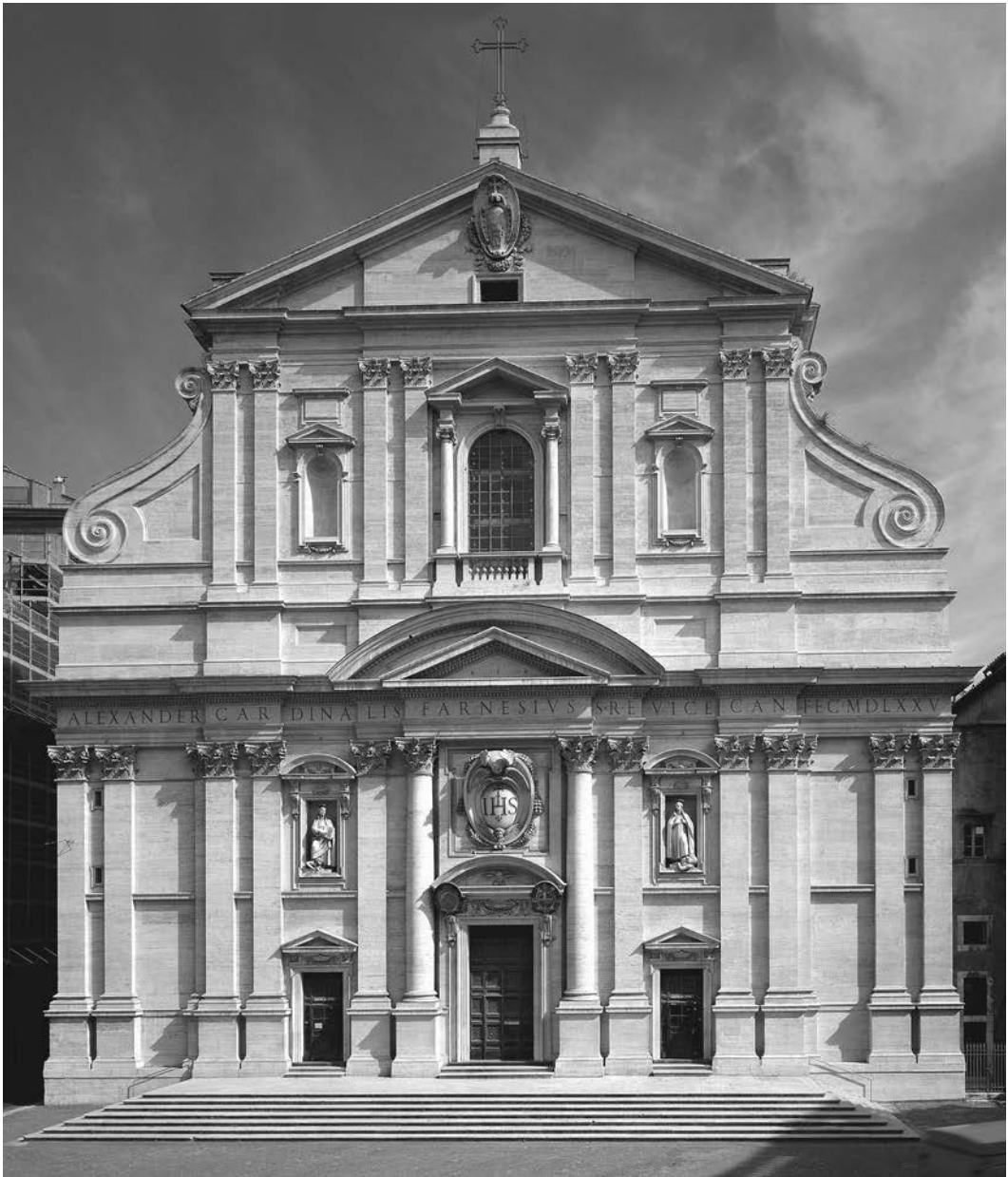
16.3. Giacomo della Porta, facade of the Gesù, Rome, Italy, 1573–1577. Giacomo della Porta, who completed the Gesù façade, was also inspired by Alberti, and used large curved volutes to make the transition from the high nave to the lower side chapels. Photo: Scala/Art Resource, NY.
