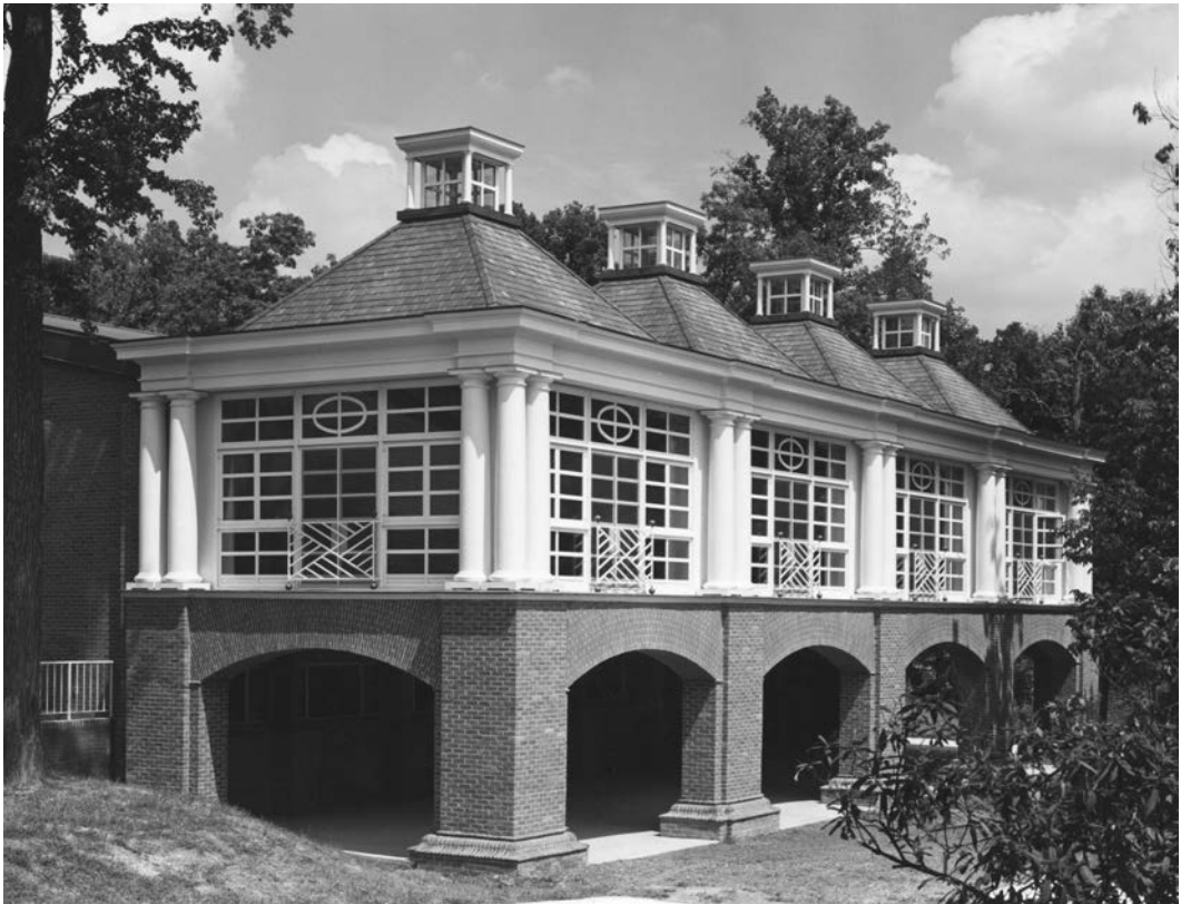
20.16. Robert A. M. Stern, Observatory Hill Dining Hall, University of Virginia, Charlottesville, Virginia, 1982–1984, demolished c. 2005. Elevating the dining rooms because of the sloping site, Stern uses brick arches and white Roman Tuscan Doric columns in an innovative way sympathetic to Jefferson's original campus buildings. Photo: Whitney Cox.
