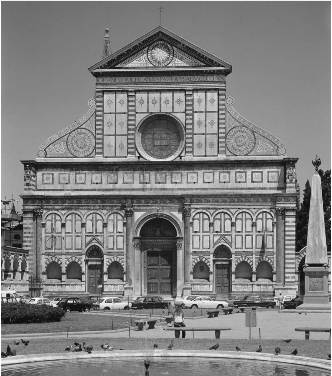
15.18. Leon Battista Alberti, facade of Santa Maria Novella, Florence, Italy, 1458–1471. In this facade design for an existing medieval church, Alberti pursued further his ideas of uniting the parts of the design by means of proportional systems as well as volutes to make the transition from tall nave to lower side aisles. Photo: Scala/Art Resource, NY.
