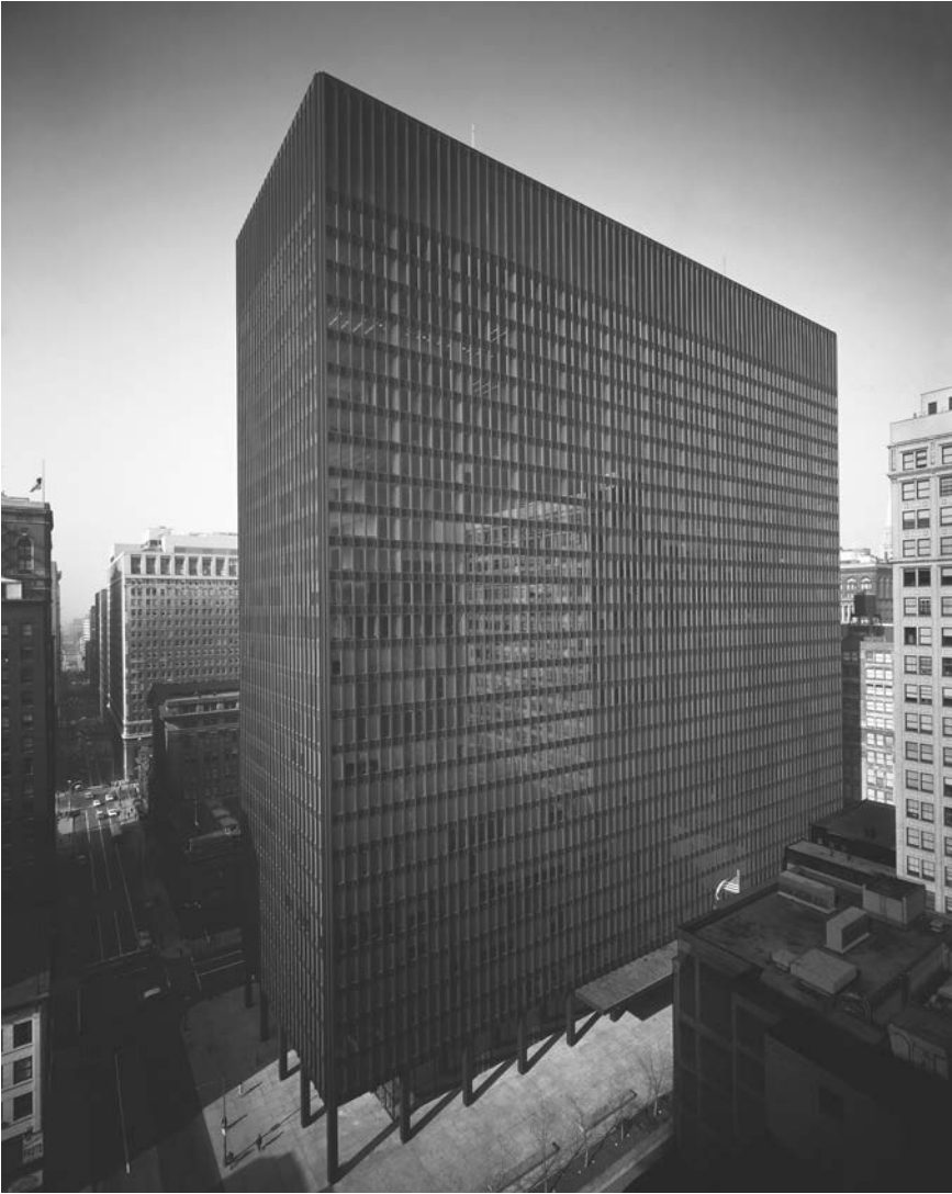
4.6. Mies van der Rohe, Federal Center Chicago, Illinois, 1959–1964 . In this design, Mies van der Rohe pulled the glass curtain wall outside the columns, resulting in absolutely uniform window bay units, and suggesting that activities within were all similar. Photo by Hedrich Blessing. Chicago History Museum, negative HB-27043d3.
