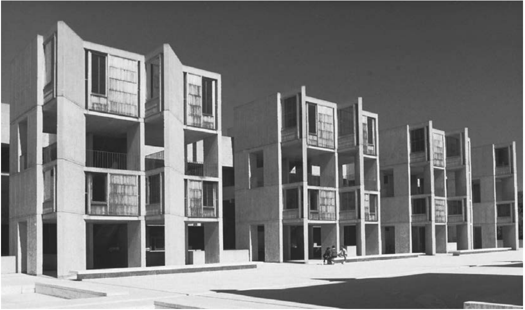
19.55. Salk Institute for Biological Studies. View of the interior court. The working areas are housed in large multifunctional spaces, whereas small, individual private studies are clustered in the central courtyard. Photo: L. M. Roth.
