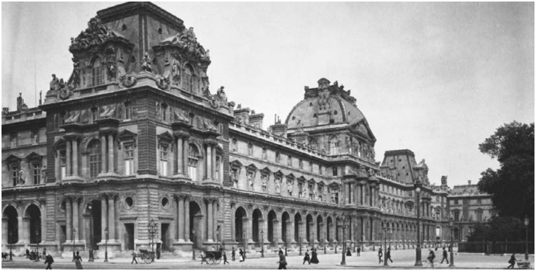
18.12. Louis Visconti and Hector-Martin Lefuel, the new Louvre, Paris, France, 1852–1857. The richly embellished French Neo-Baroque style was developed by Visconti and Lefuel to integrate the new additions to the building with the original portions of the Louvre, built in the sixteenth and seventeenth centuries. Photo: Giraudon/Art Resource, NY.
