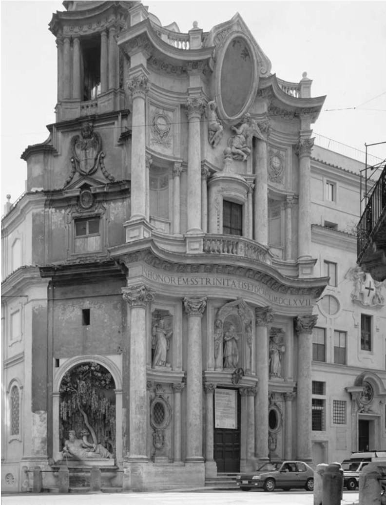
16.15. San Carlo alle Quattro Fontane, facade built 1662–1667. Exterior. Photo: Scala/Art Resource, NY.
