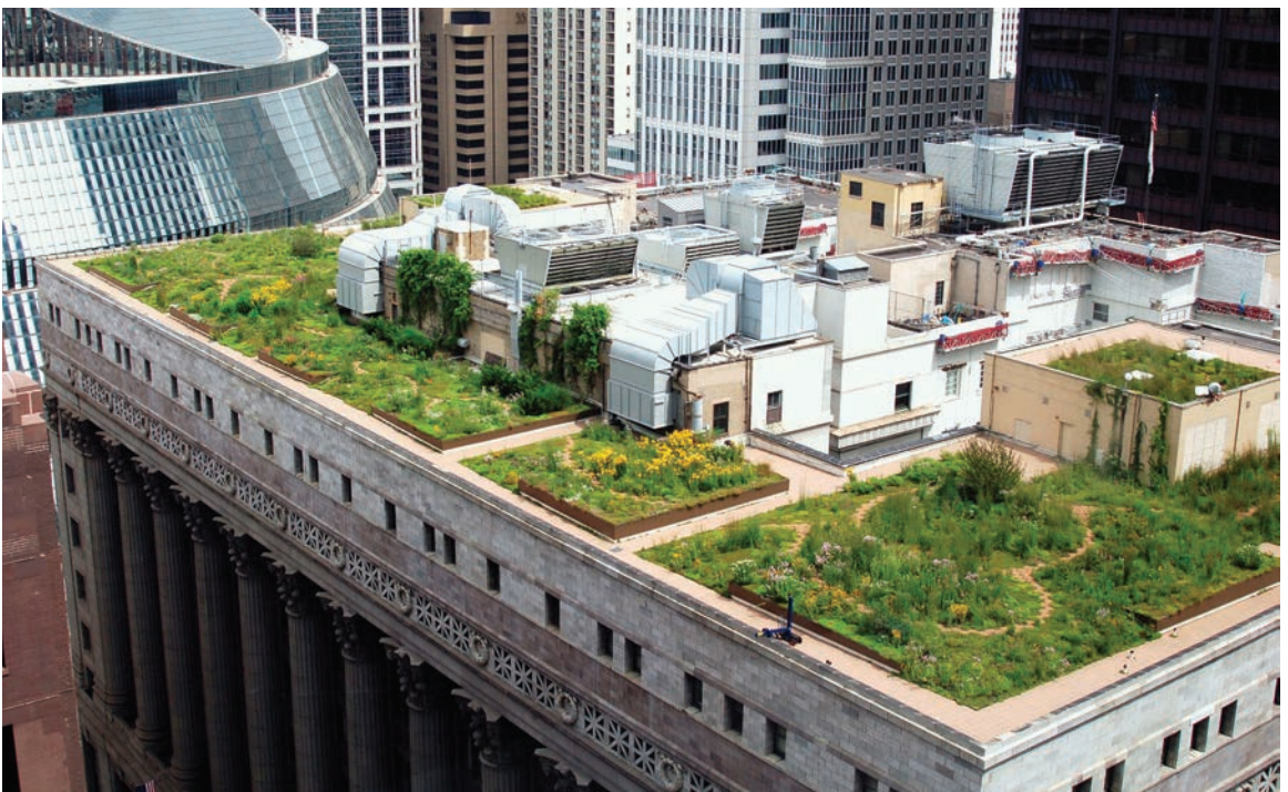
Plate 51. Conservation Design Forum, Inc., City Hall Building Roof Garden, Chicago, Illinois, 2001. Positioned in a very prominent political location is this dramatic demonstration of making a useful place while significantly reducing ongoing building energy demands. Photo: Chicago Department of Environment/Mark Farina/AP.
