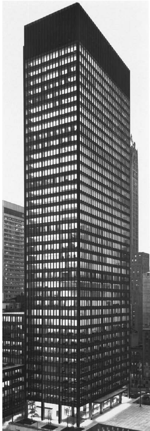
6.14. Seagram Building. This twilight view reveals how transparent the building is to radiant energy. Despite the darkly tinted glazing, during the day sunlight passes into the building, heating it up; but in the winter just as easily heat escapes at night. Photo: Ezra Stoller © Esto.
