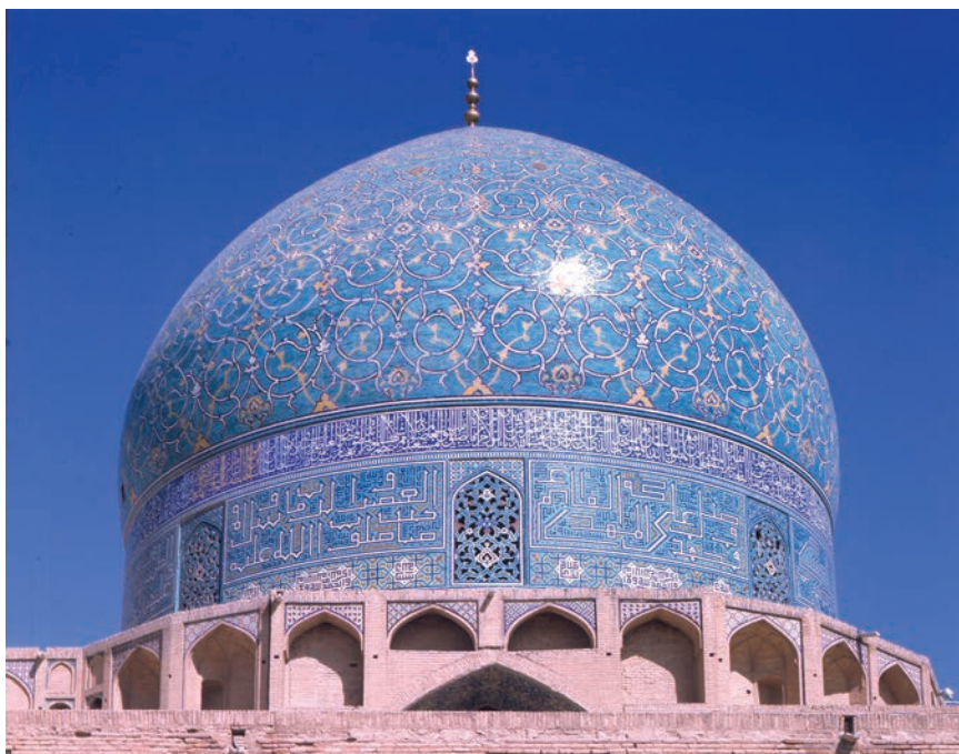
Plate 8. Masjed-i-Shah Mosque, Isfahan, Iran, 1611–1638. The glistening glazed tiles that cover the softer, structural material bring a note of vivid color to Islamic architecture. Photo: SEF/Art Resource, NY.
