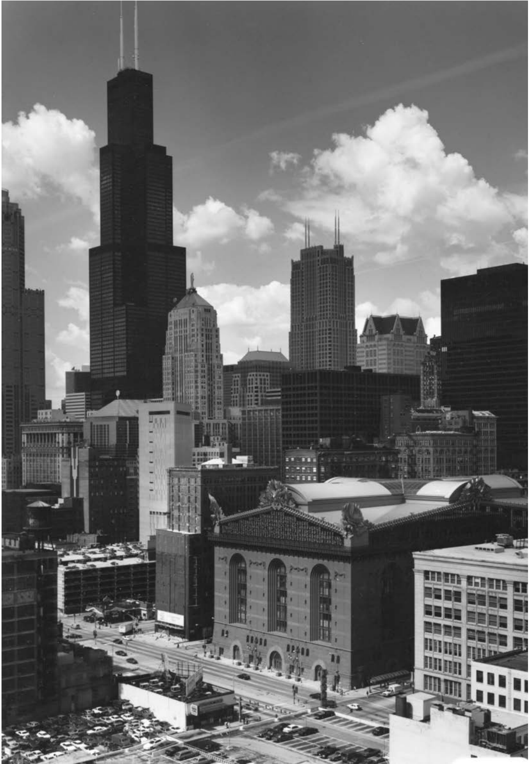
20.17. Hammond, Beeby, and Babka, Harold Washington Library Center , Chicago, Illinois, 1987–1991. Responding to the downtown Chicago location, the architects incorporated many generic references to numerous surrounding historic early skyscrapers. Photo: Courtesy of Hamman, Beeby and Babka.
