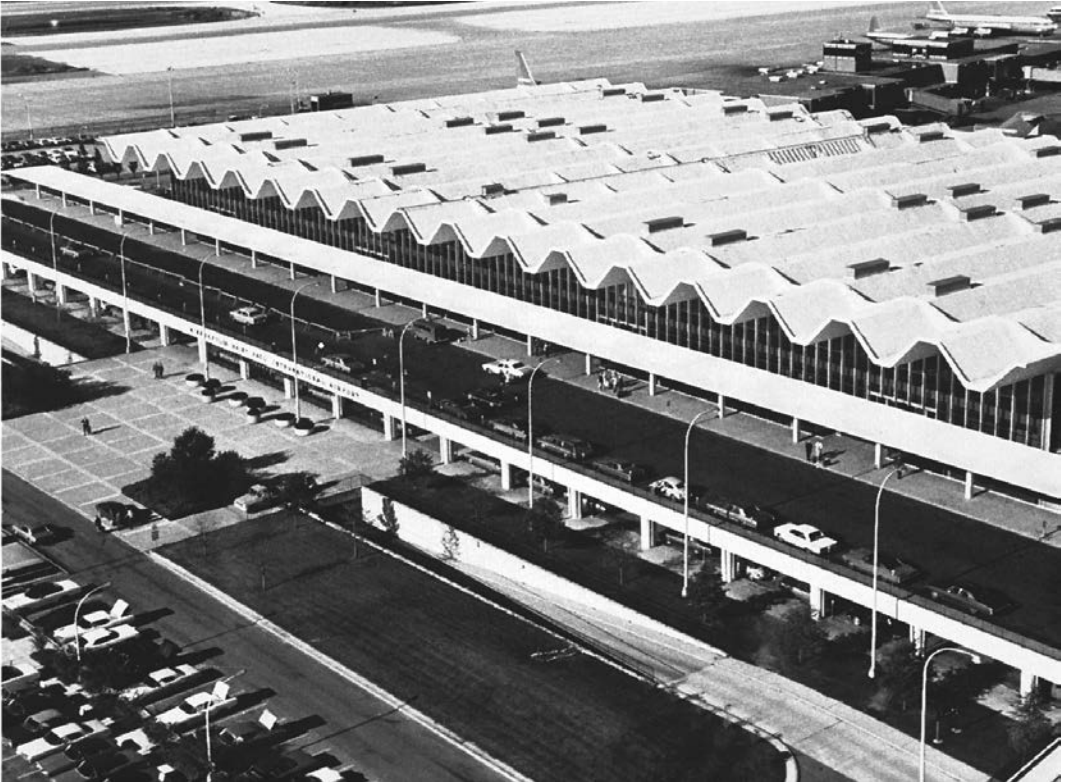
3.37. Cemy Associates, Minneapolis International Airport Terminal, Minneapolis, Minnesota, 1962–1963. The roof has the form of a folded plate similar to a simple accordion-fold fan. Photo: Ron Tadsen.
