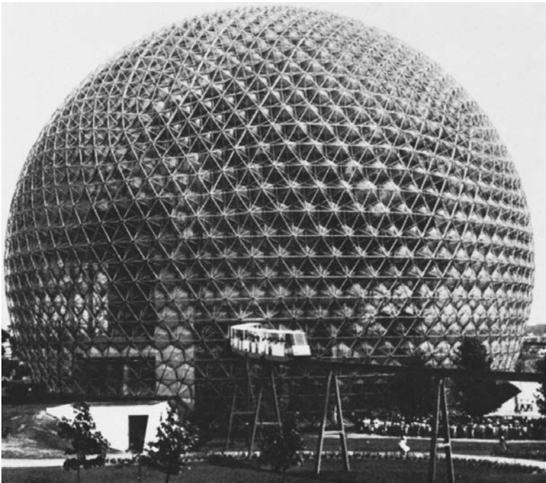
3.35. R. Buckminster Fuller. United States Pavilion, 1967 World's Fair, Montreal, Quebec, Canada, 1967 (destroyed by fire, 1976). In this structure a space frame is curved to enclose a sphere. Photo: Ilse Friesmen, courtesy of R. Buckminster Fuller.
