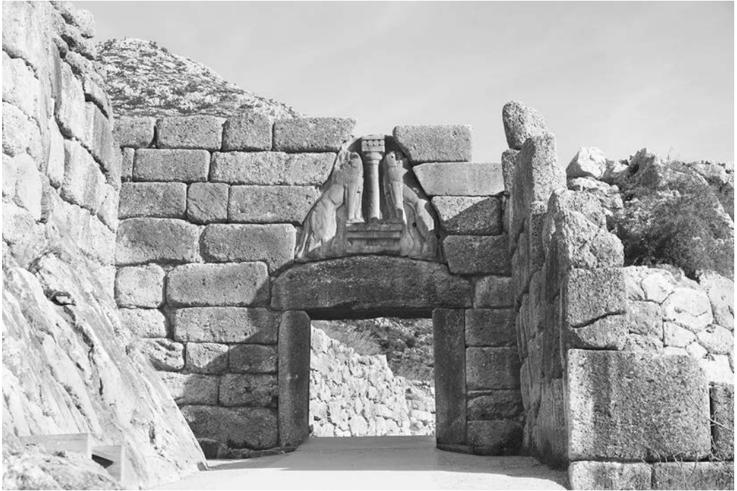
11.3. City walls and Lion Gate, Mycenae, Greece, c. 1300 BCE. The huge size, roughness, and irregularity of the stones in the wall greatly impressed the later Greeks of the Classical age. The Lion Gate still makes a strong impression on approaching visitors. Photo: Manuel Cohen/The Art Archive at Art Resource, NY.
