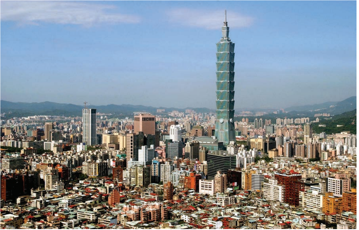
Plate 39. C. Y. Lee, Taipei 101, Taipei, Taiwan, 1997–2003. Taiwanese architect Lee achieved a form suggestive of a gigantic pagoda, with its upper portion divided in eight sections of eight floors each, a most auspicious number in Chinese culture. Photo: AP Images/Wally Santana.
