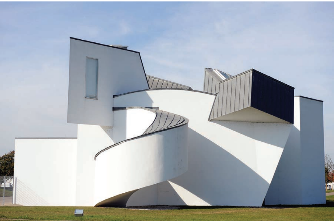
Plate 40. Frank Gehry, Vitra Design Museum, Weil am Rhein, Germany, 1987–1989. Beginning to create elaborately sculpted building forms in the 1980s revealed to Gehry the complicated issues involved in producing working drawings for such complex nonlinear forms. Photo: © Caro/Alamy.
