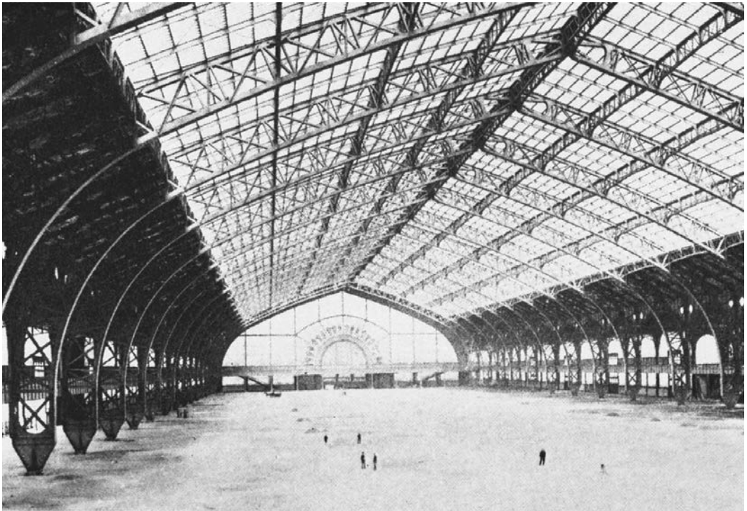
18.23. Charles-Louis-Ferdinand Dutert, with Contamin, Pierron, and Charton, Palais des Machines, Paris, France, 1886–1889. Designed to house all the major machinery exhibits of the Paris World's Fair of 1889 and marking the centennial of the French Revolution, this vast shed had a span of 377.3 feet (115 m). It is shown here just after construction ended and before the exhibits were installed. From N. Ponente, The Structures of the Modern World, 1850–1900 (New York, 1965).
