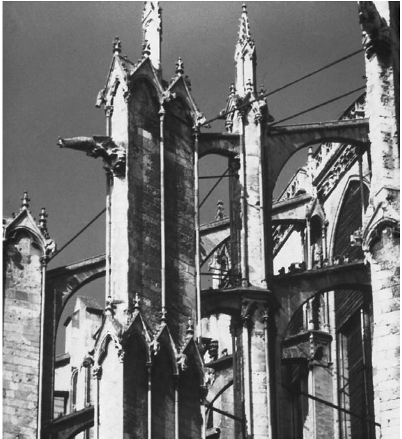
4.31. Notre-Dame de Amiens, Amiens, France, 1221–1269. The gargoyles on the buttresses of the choir serve the very practical purpose of throwing rainwater away from the building. Photo: Sandak, University of Georgia.
