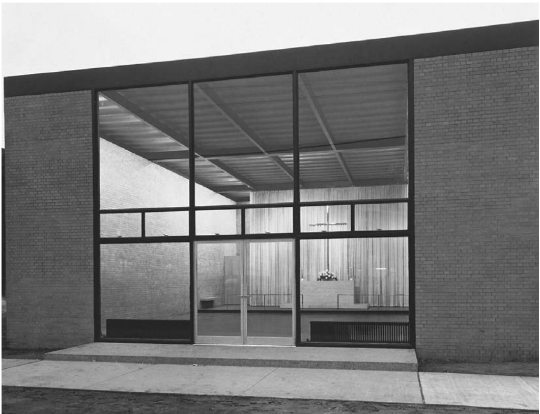
19.39. Mies van der Rohe, Chapel, Illinois Institute of Technology, Chicago, Illinois, 1949–1952. Although a chapel, it has none of the conventional clues as to its function. Photo: Hedrich-Blessing, Chicago. Photo by Hedrich Blessing, Chicago History Museum, negative HB-15691-D.
