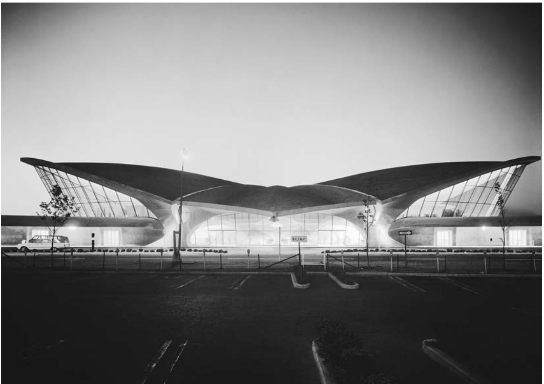
19.47. Trans World Airlines Terminal, John F. Kennedy Airport. This night view, taken from the parking area, shows well the enormous reach of the 80-foot cantilevered roof shells. Photo: Ezra Stoller © Esto. All rights reserved.
