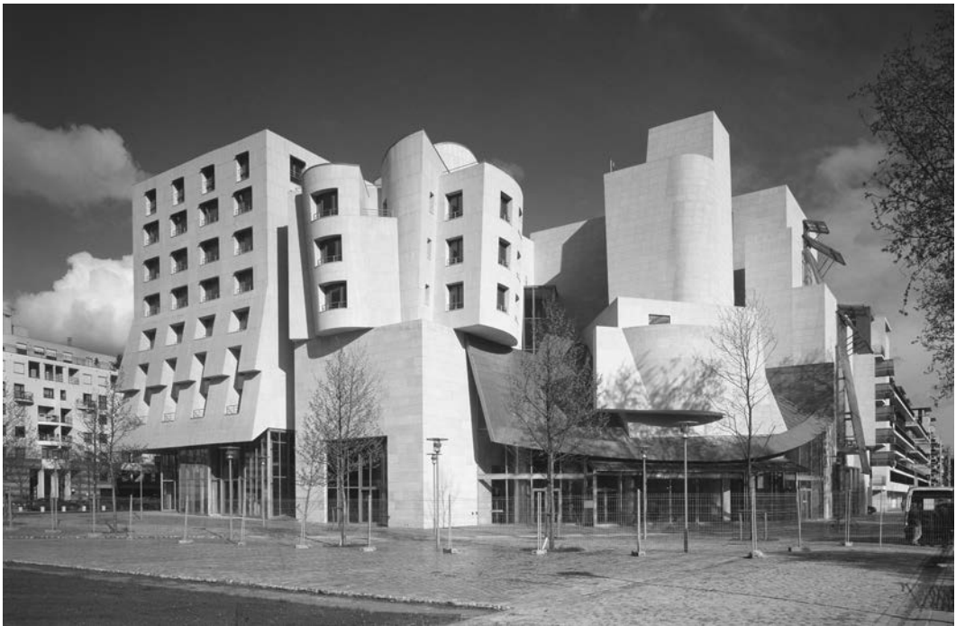
20.33. Frank Gehry, American Center, Paris, France, 1988–1994 . Moving away from the angular straight-line forms of his work in the previous decade, Gehry confronted the difficulty in hand-drawing construction drawings for free-form buildings, prompting his firm's interest in using the French aviation design software, CATIA. Photo: View Pictures Ltd/SuperStock.
