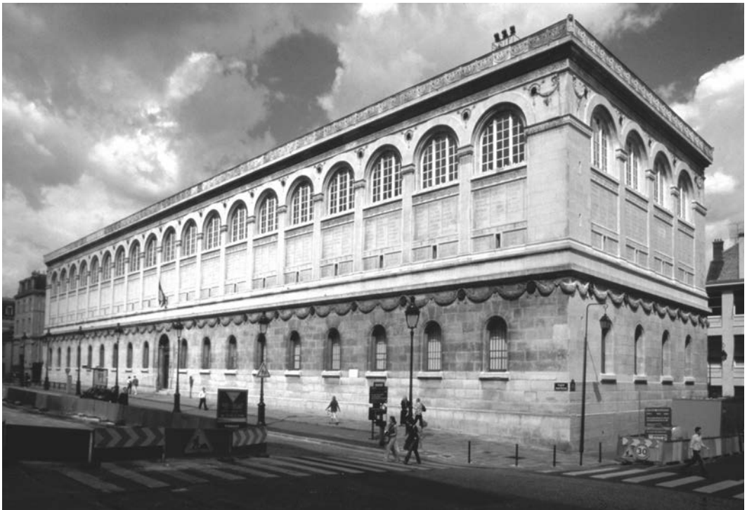
18.37. Henri Labrouste, Bibliothèque Sainte-Geneviève , Paris, France, 1838–1850. In this public reference library, framed in iron, Labrouste took care to define urban space and to let the external form and details of the building speak of its internal function by means of the glazed arcade and the inscribed authors' names. Photo: L. M. Roth, 2003.
