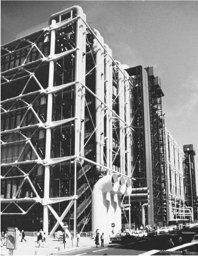
20.26. Renzo Piano and Richard Rogers, Centre Georges Pompidou, Paris, France, 1971–1977. This museum has been turned inside out, so to speak, with the structure and building utilities externalized so that the internal spaces can be opened up. Photo: Michel Proulx, Architectural Record .
