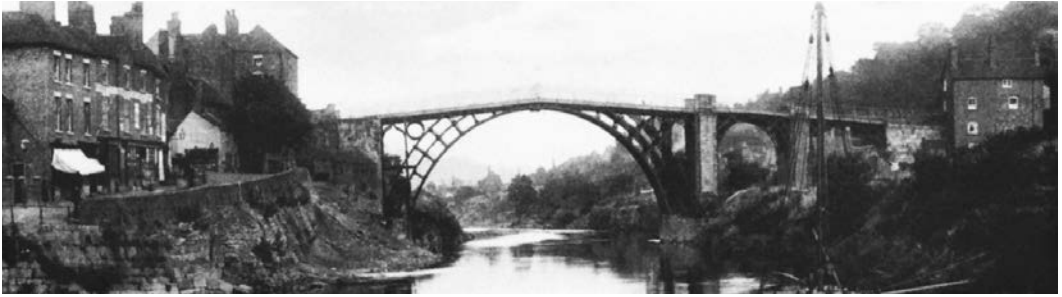
17.31. John Wilkinson, Thomas F. Pritchard, and Abraham Darby III, Coalbrookdale Bridge, Coalbrookdale (Ironbridge), England, 1777–1779. One of the first demonstrations of the dramatic potential of cast iron as a structural material, this bridge was cast in 50-foot-long half sections. Photo: British Museum, London; Courtesy, the Trustees.
