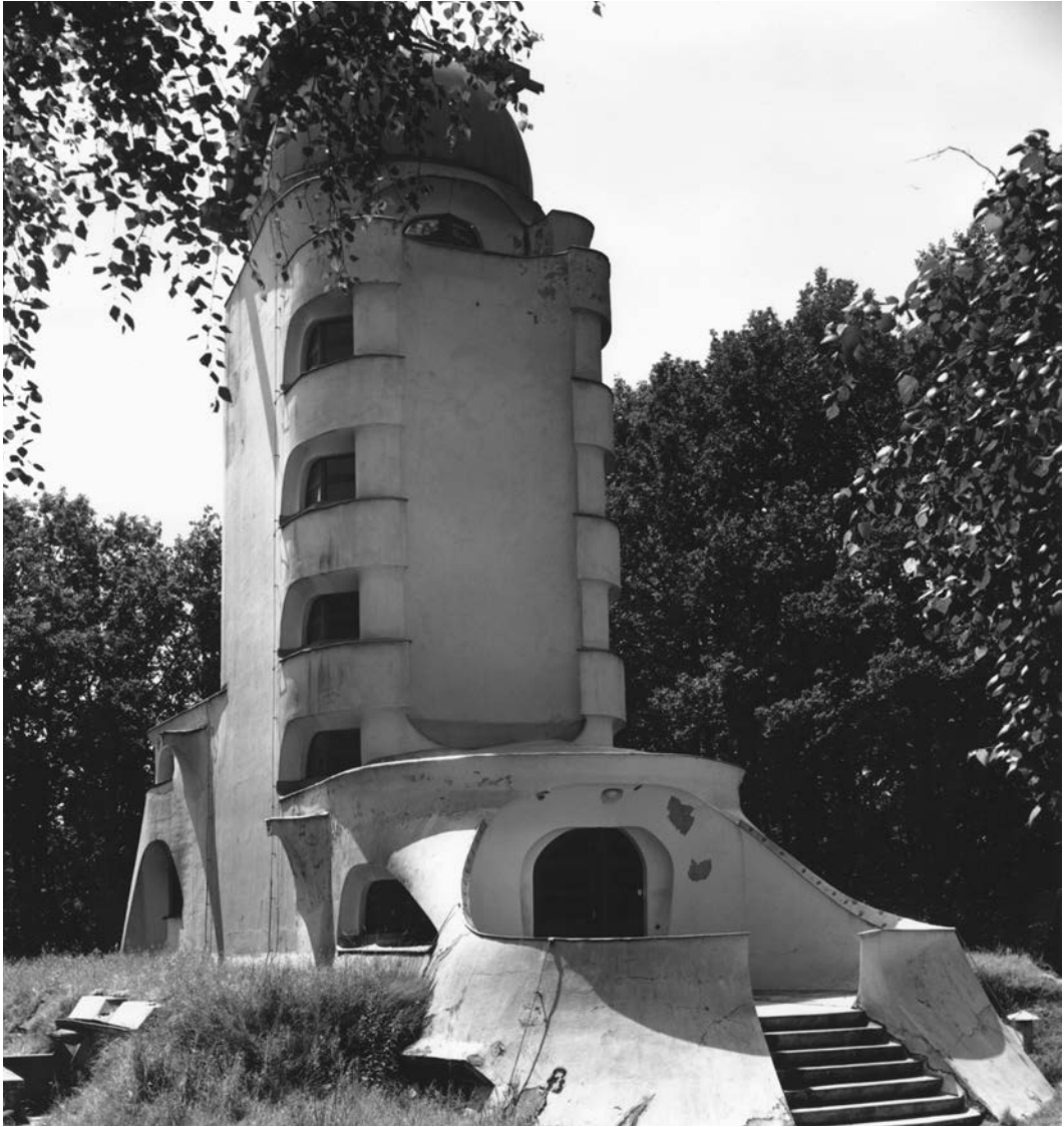
19.13. Erich Mendelsohn, Einstein Tower , Potsdam, near Berlin, 1917–1921. Designed especially to house equipment to test Einstein's theory of relativity, this also was meant to suggest an image of modern Promethean power. Photo: © Wayne Andrews/Esto. All rights reserved.
