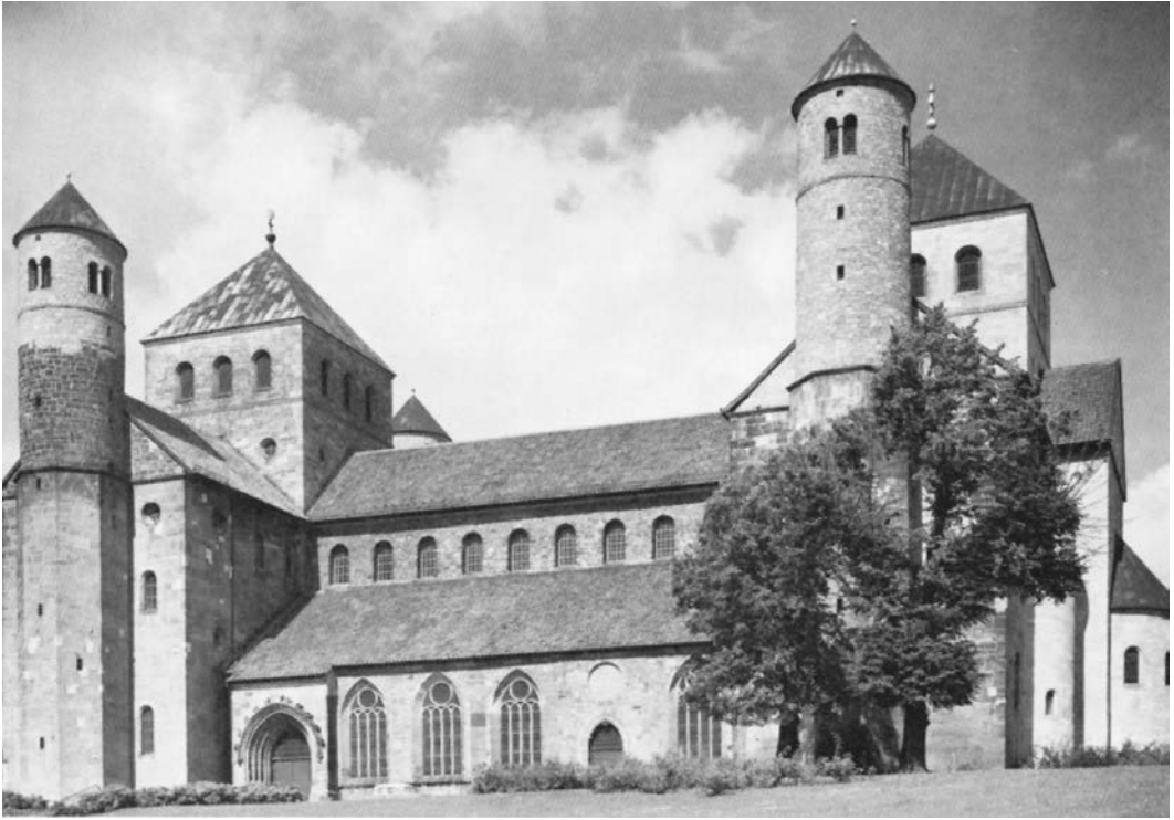
14.16. Monastery Church of Saint Michael, Hildesheim, Germany, 993–1022. View. Because this was built outside and north of the walls of the city, the church has massive stone walls to withstand attack. Yet the towers point heavenward, so that the church is both a stronghold and a gate to heaven. Photo: A. F. Kersting, London.
