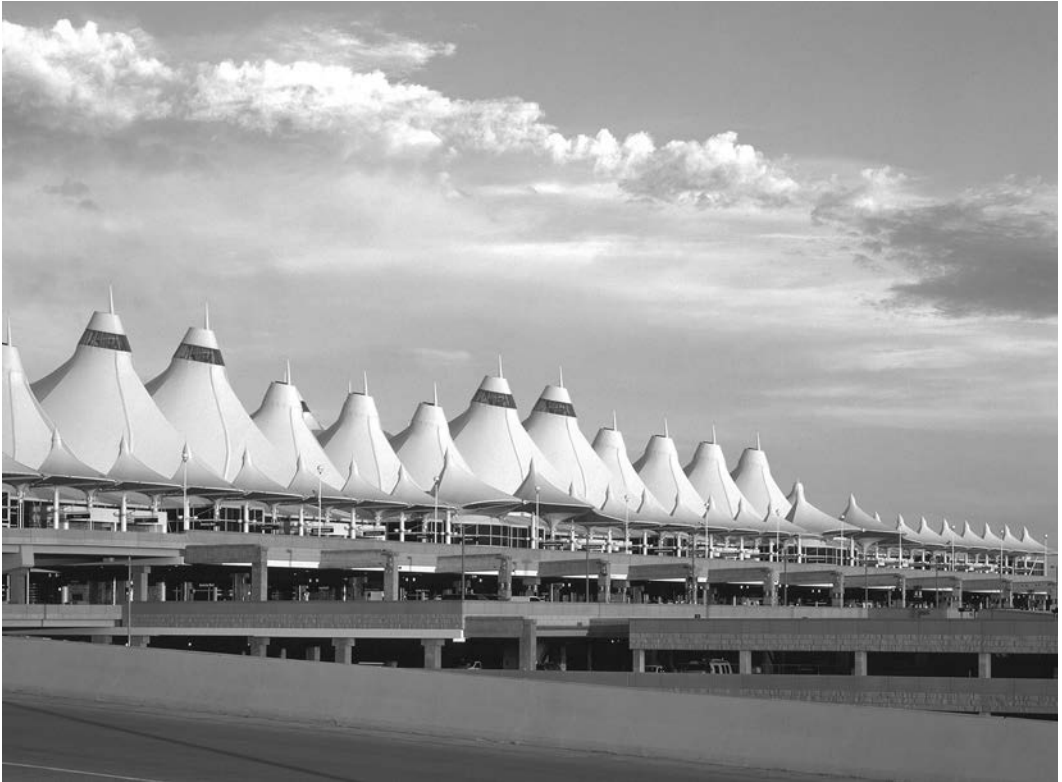
3.47. Fentress Bradburn Architects, Denver International Airport arrival terminal, Denver, Colorado, 1991–1995. Fiberglass-reinforced fabric is stretched from several masts to create this multi-peaked tent-like pavilion. Photo courtesy of Fentress Bradburn Architects.
