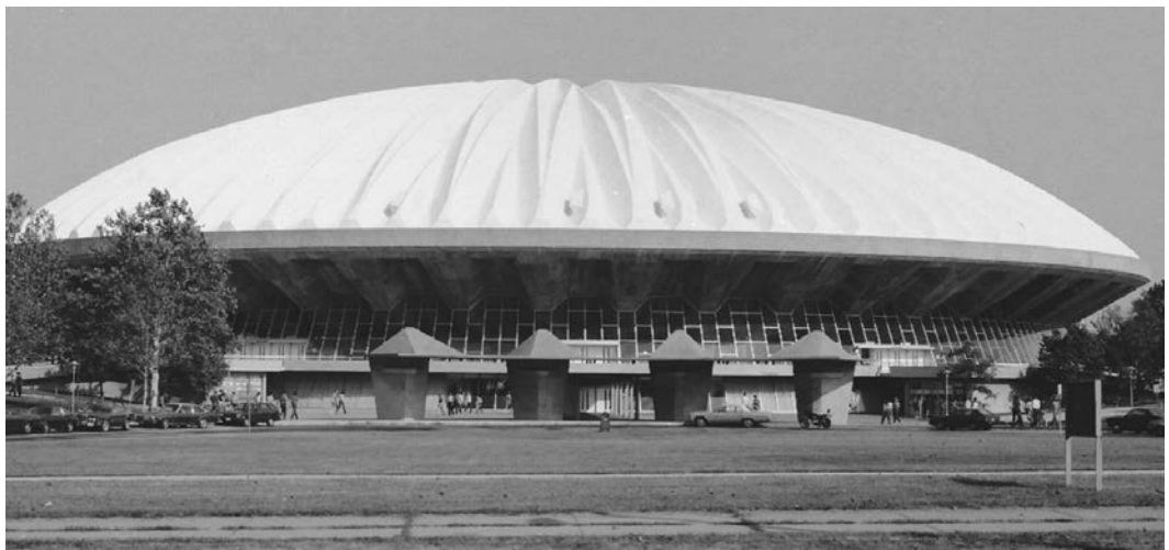
3.38. Harrison and Abramovitz with Ammann and Whitney, engineers, University of Illinois Assembly Hall, Champaign, Illinois, 1961–1962. This folded plate shell dome has folded corrugations radiating from the center. Photo: Courtesy, University of Illinois.
