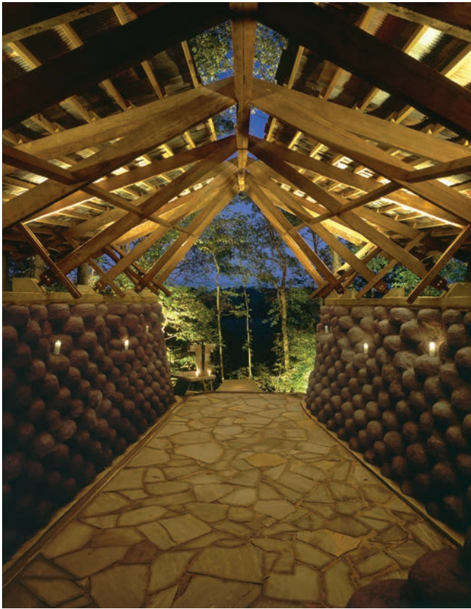
Plate 50. Samuel Mockbee with the Rural Studio, Yancey Chapel, Sawyerville, Hale County, Alabama, 1995. Using found materials such as discarded tires and salvaged wood, Mockbee and his architecture students provided needed buildings for rural people with extremely limited means. Photo: Timothy Hursley.
