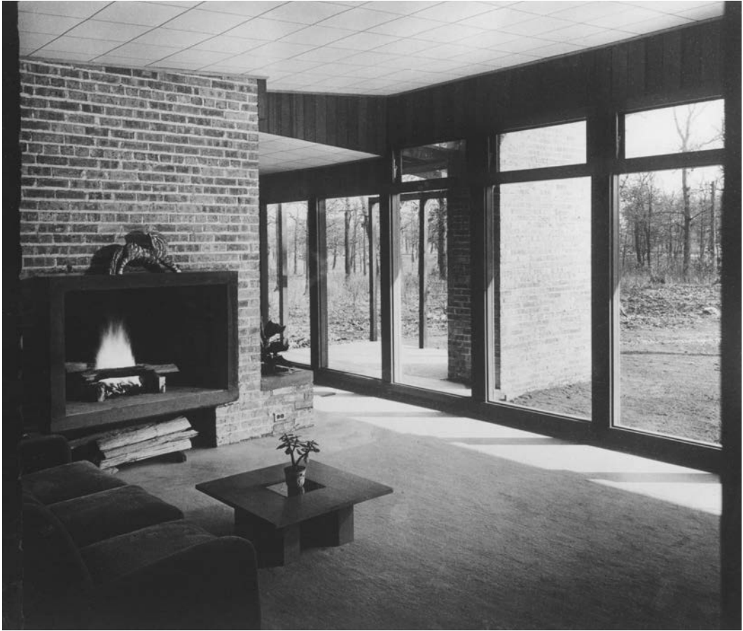
6.9. George Fred Keck and William Keck, Hugh D. Duncan house, Flossmoor, Illinois, 1941. In the mid-afternoon, since the house faces south, the roof overhang prevents the sun from penetrating very far into the room to keep the heat load down. Photo: C. Condit Collection, Department of Art History, Northwestern University.
