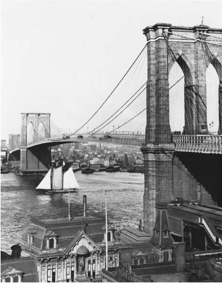
3.41. John Augustus Roebling, Brooklyn Bridge, New York, NY, 1867–1883. This bridge established the structural basis for all modern suspension bridges; its wrapped steel wire cables were among the first instances of steel being used in an American structure. Photo: Courtesy, The Long Island Historical Society.
