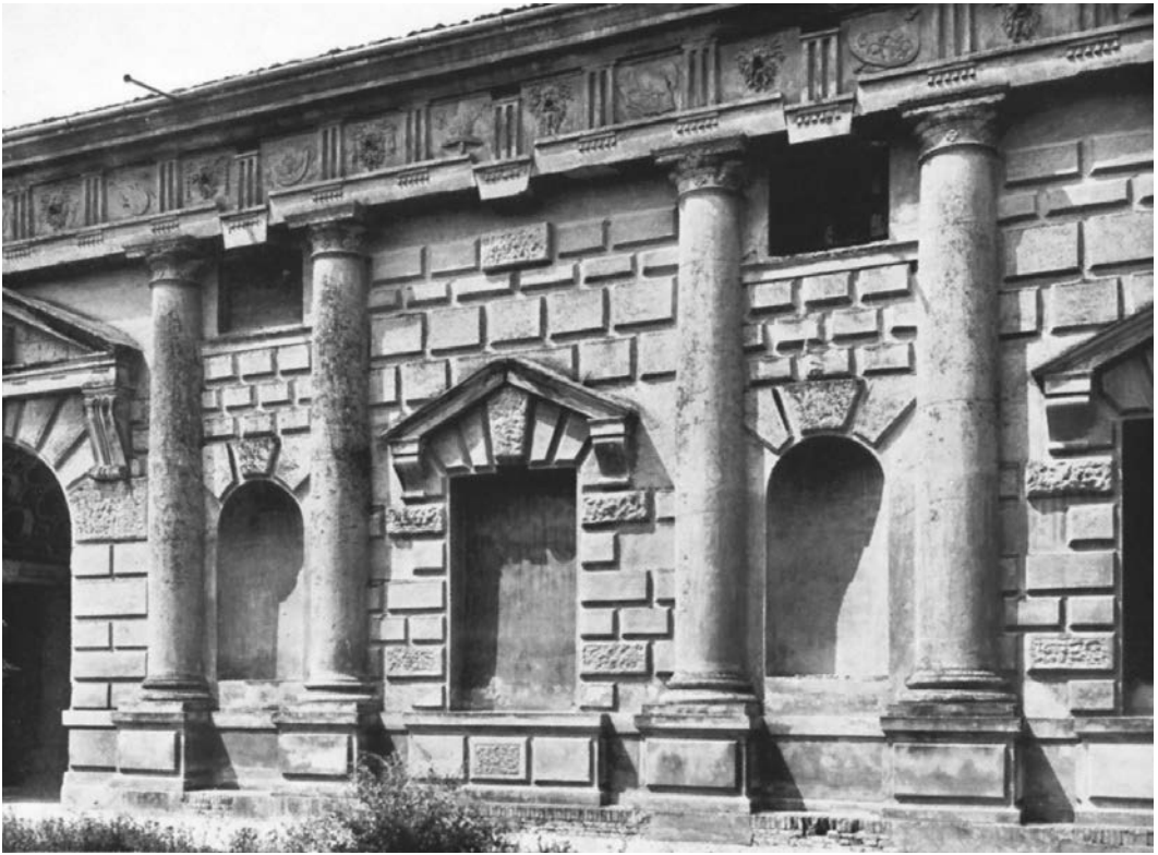
15.39. Giulio Romano, Palazzo del Te , Mantua, Italy, 1527–1534. View of the inner court. In the inner court, architectural elements are exaggerated, some are missing altogether, and what should be a straight architrave beam has keystones slipping out of place. Photo: Gabinetto Fotografico Nazionale, Rome.
