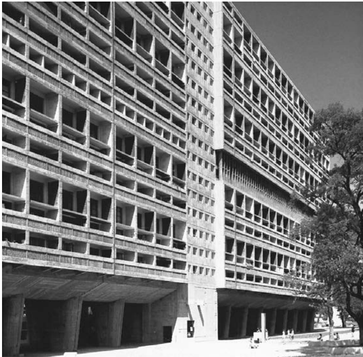
4.15. Le Corbusier, Unité d'Habitation, Marseilles, France, 1946–1952. The entire building, in all its parts, was proportioned using the Modulor and its numerical relationships based on the Fibonacci series (1:2:3:5:8, etc.). Photo: © Wayne Andrews/Esto. All rights reserved.
