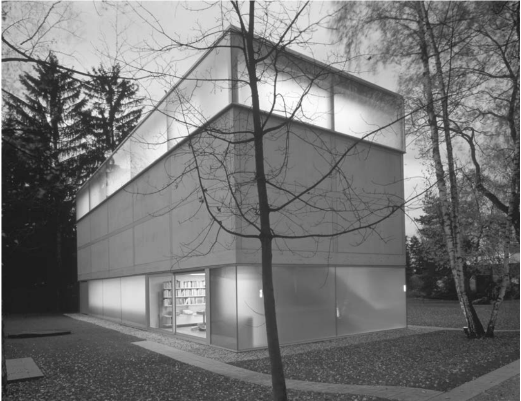
20.11. Herzog & de Meuron, Goetz Art Gallery, Munich, Germany, 1989–1992. The austere and pristine glass box of the Goetz Art Gallery is an excellent example of the minimalist architecture of the 1990s. Photo: Margherita Spiluttini, Schonlaterngasse 8, A-1010 Vienna, Austria.
