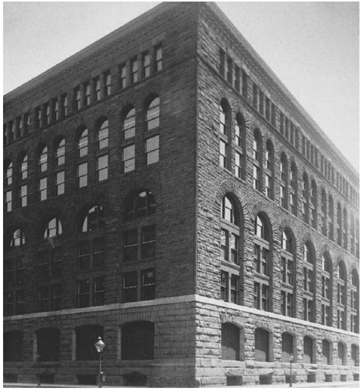
18.42. Henry Hobson Richardson, Marshall Field Wholesale Store, Chicago, Illinois, 1885–1887 (demolished 1930). For this utilitarian building, Richardson simplified his masonry, unifying this massive commercial block by the repetition of window arcades. Photo: Charles Allgeier, Chicago, c. 1887; author's collection.
