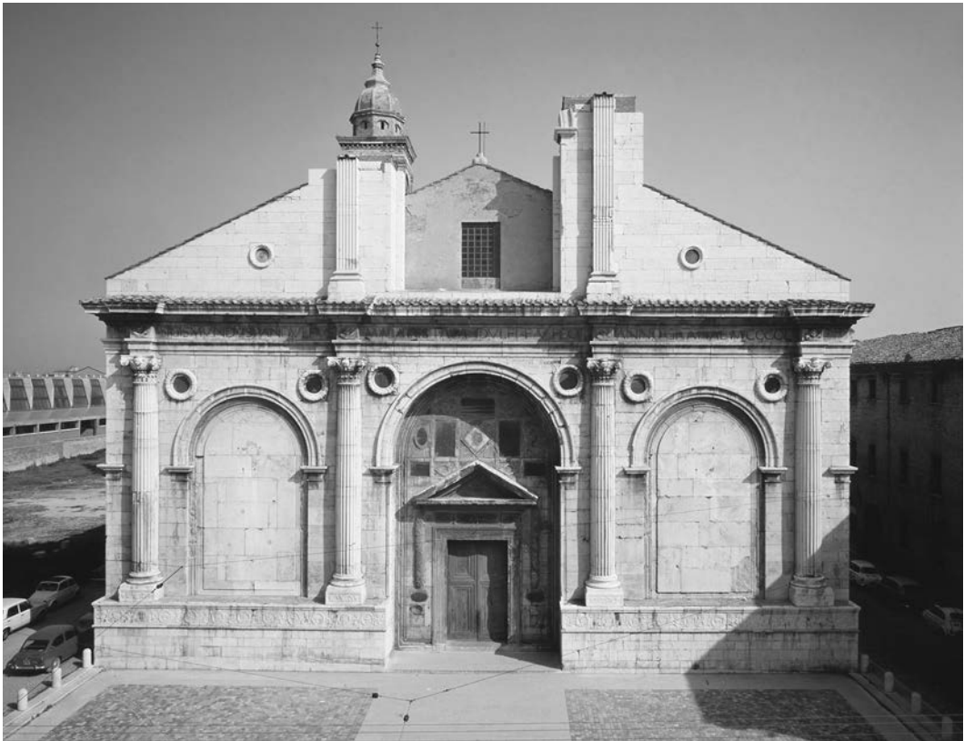
15.16. Leon Battista Alberti, Church of San Francesco (the Tempio Malatestiano), Rimini, Italy, 1450–1461. This new shell, wrapped around an existing medieval church, is based on Roman triumphal arch forms. Photo: Scala/Art Resource, NY.
