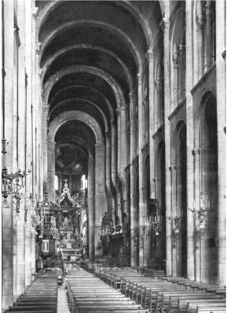
14.25. Saint-Sernin, Toulouse. In this interior, as at Saint-Martin-du-Canigou, the difficulty of admitting light in a barrel-vaulted nave is clear; much of the light comes through the later Gothic rose window at the west end. Photo: Jean Roubier, Paris.
