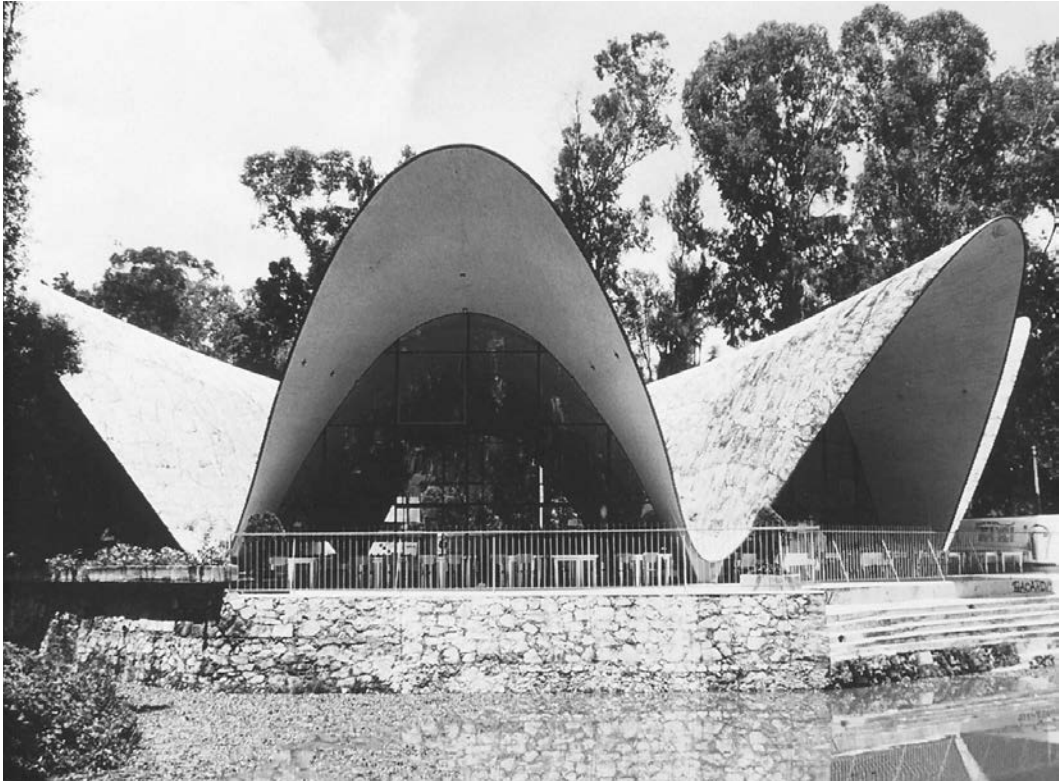
3.36. Félix Candela, restaurant, Xochimilco, Mexico, 1958. The building shell is built of concrete applied over a mesh of steel wire, with a total thickness of about 4 inches. Photo: George Andrews, courtesy of the Visual Resources Collection, Architecture & Allied Arts Library, University of Oregon.
