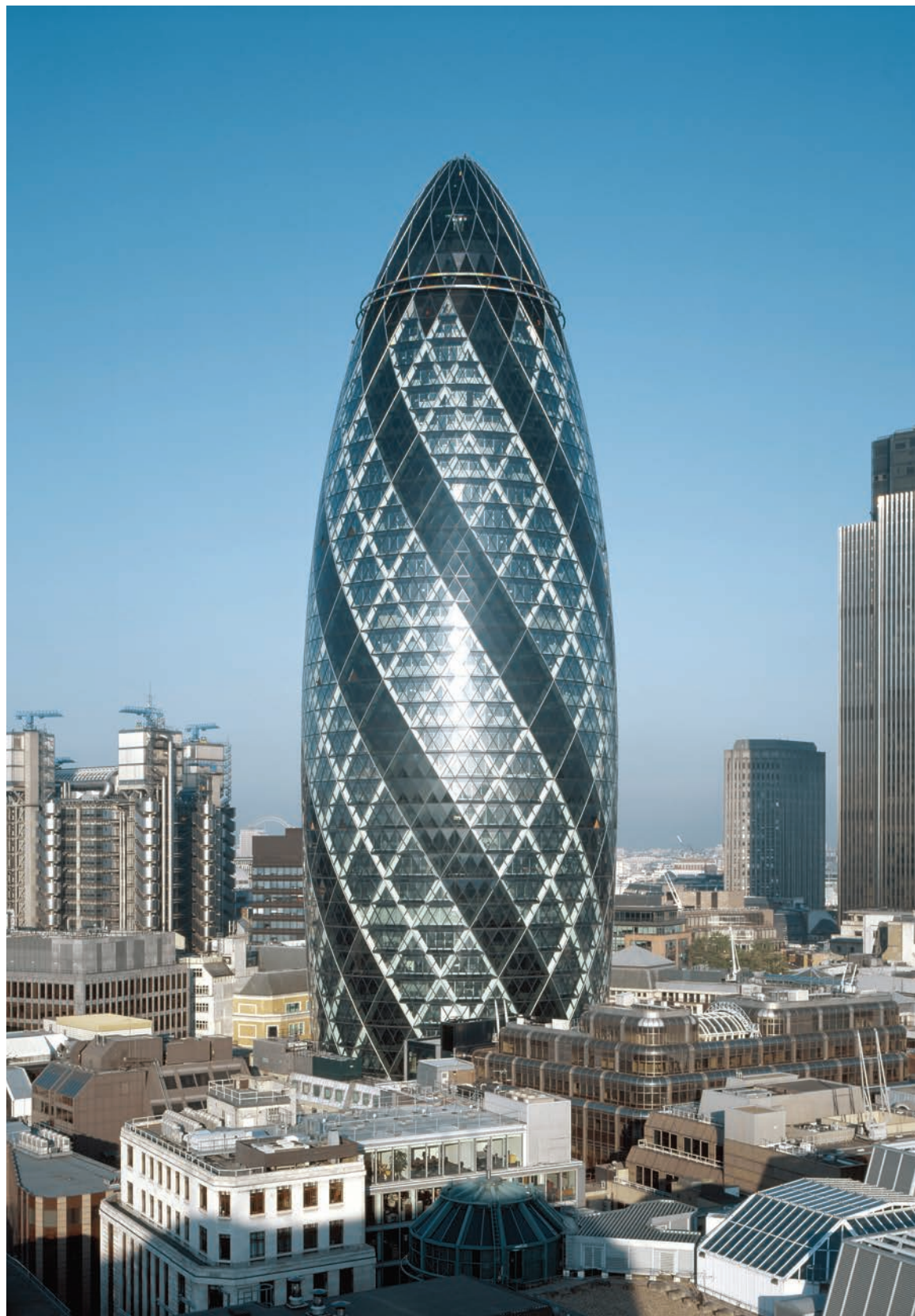
Plate 38. Norman Foster, 30 St. Mary Axe (“The Gherkin”), London, England, 1996–2004. Employing whimsy in both form and color, Foster created a distinctive building incorporating positive energy-saving attributes. Photo: UIG/Getty Images.
