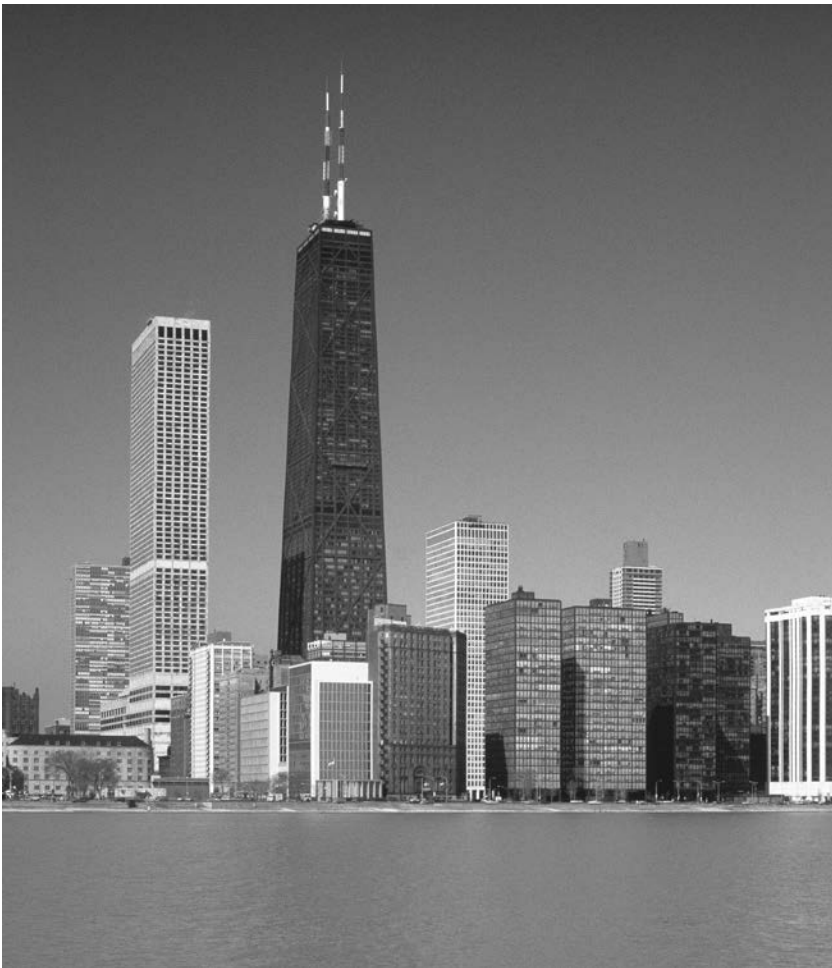
6.16. Skidmore, Owings & Merrill, John Hancock Center, Chicago, Illinois, 1965–1970. In buildings of great height, the lateral pressure of the wind becomes a more significant structural design factor than vertical gravity-generated forces; hence, as in the Hancock Center, large-scale externalized diagonal bracing stiffens each of the vertical columns. The shorter twin buildings just to the right, below the Hancock Center, and closer to the lake, are the Lake Shore Drive apartment buildings by Ludwig Mies van der Rohe, 1948–1951. Photo: L. M. Roth.
