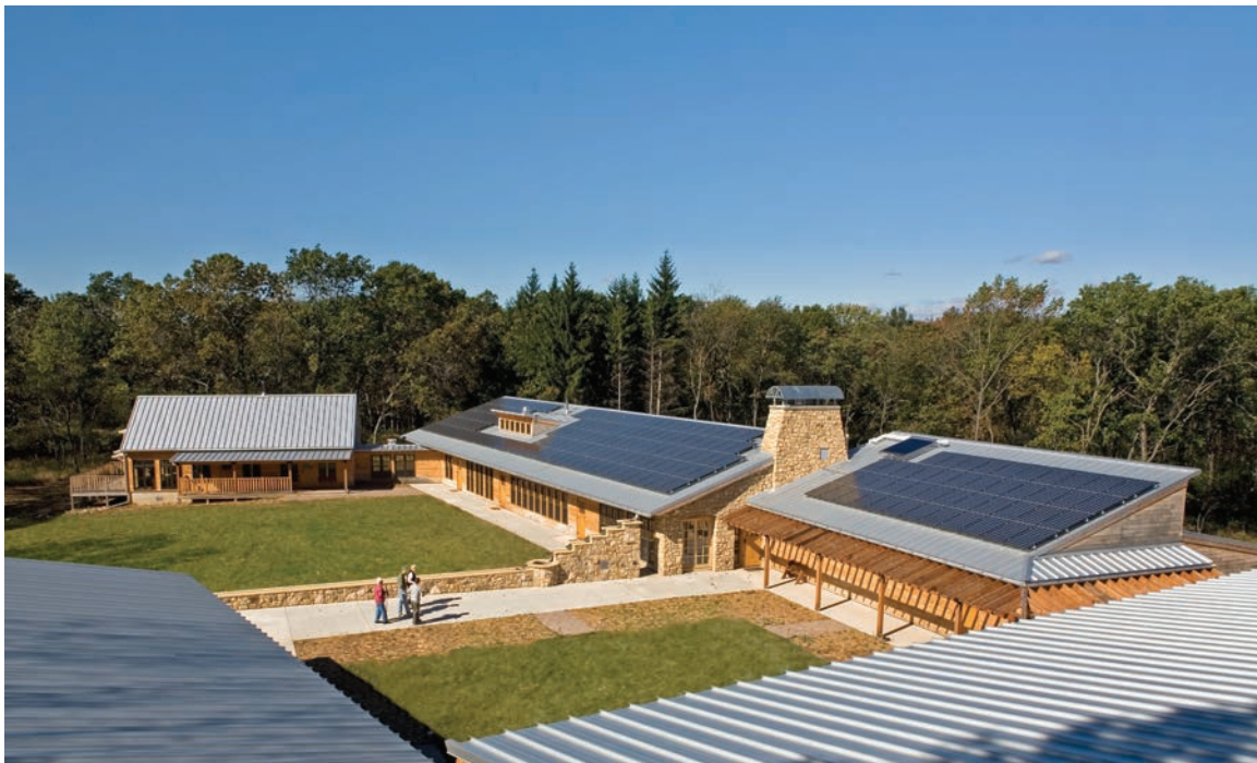
Plate 48. The Kubala Washatko Architects (TKWA), Aldo Leopold Legacy Center, Baraboo, Wisconsin, 2006–2007. The connection to the earth is maintained through exposed wood structure and rough stone, while the roof is almost entirely covered with photo-voltaic panels providing all needed energy. Photo: © The Kubala Washatko Architects, Inc./Mark F. Heffron.
