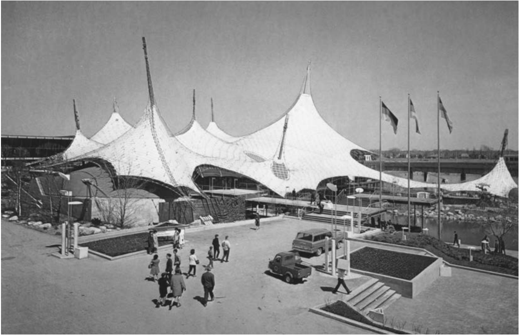
3.46. Frei Otto, German Pavilion , 1967 World's Fair Montreal, Quebec, Canada, 1967. In this building the protective enclosure is provided by a membrane held taut by cables stretched from masts to the ground. Photo: From W. Hoffmann and U. Kultermann, Modern Architecture in Color (New York, 1970).
