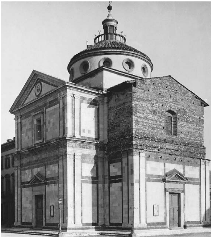
15.12. Giuliano da Sangallo, Santa Maria delle Carceri , Prato, Italy, 1485–1491. Sangallo used the proportional ideal to construct a centralized church generated by a square and cube at its center. Photo: Alinari/Art Resource, NY.
