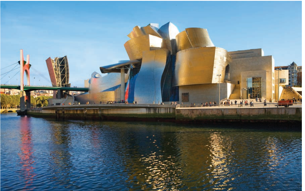
Plate 41. Frank Gehry, Guggenheim Museum, Bilbao, Spain, 1987–1997. The shimmer of the thin titanium sheets almost instantly established a new worldwide standard of prestige in turn-of-the-twentieth-century public architecture. Photo: © Art Kowalsky/Alamy.
