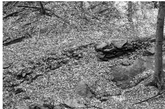
Old path supported by a dry wall in a side ravine below a rocky outcrop. A side path branches off from this road, climbing in serpentine to a rocky outcrop and higher.
