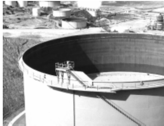
Figure E-6a—Open Top (External) Floating Roof Tank
