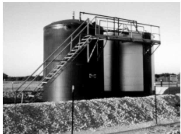
Figure E-2—Low-Pressure Tanks without Weak Seam
