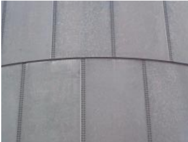
Figure E-4—Close-up View of Bolted Tank Seams
