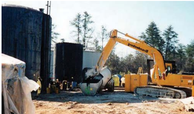
Figure 8.24 Purging tanks during decommissioning
