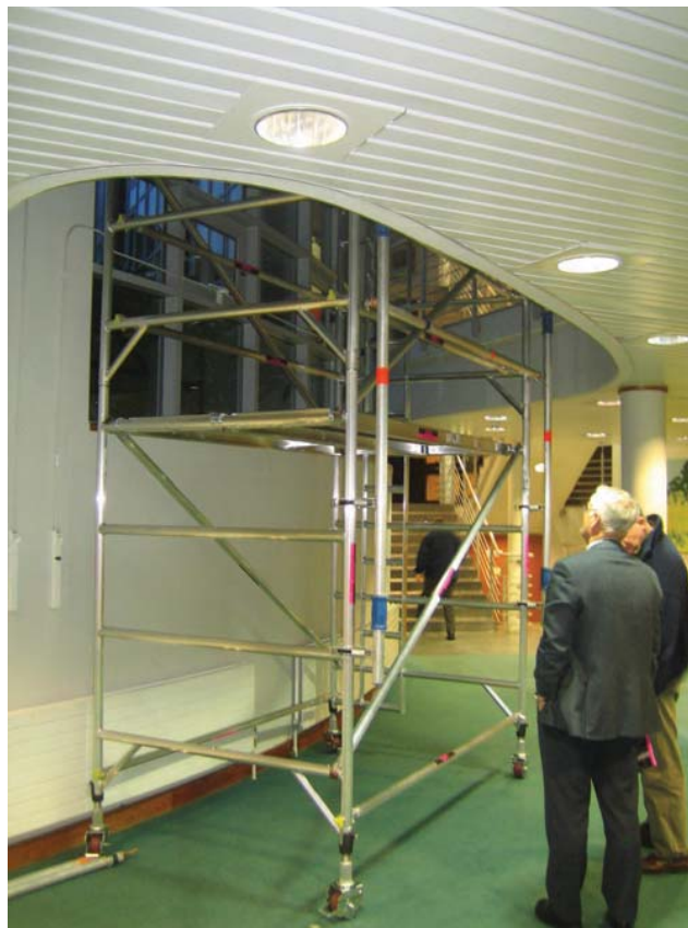
Figure 5.2 Inspecting contractors arrangements for working at height
