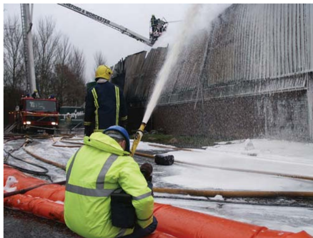
Figure 13.6 Boom used to catch overflow from bunded area
