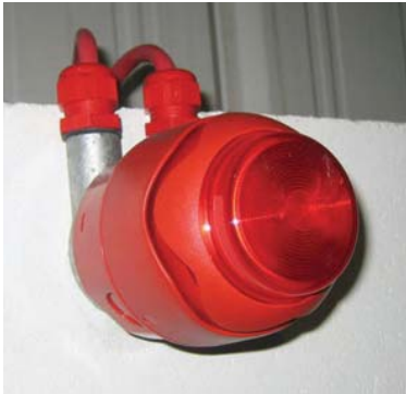
Figure 10.18 Visual alarm combined with an audible sounder
