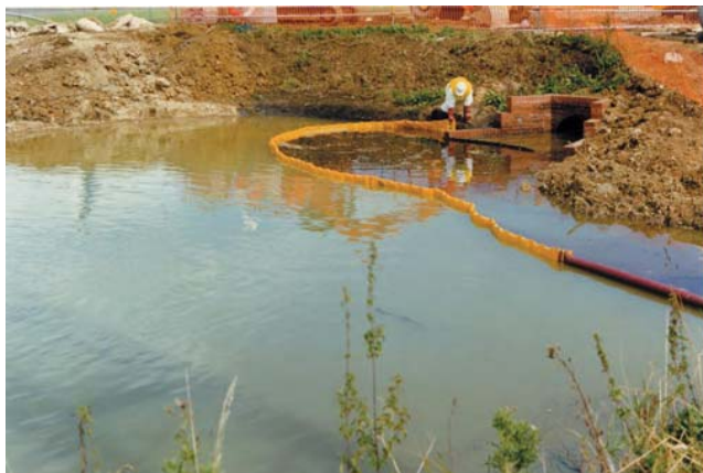
Figure 13.9 A boom designed to limit contamination
