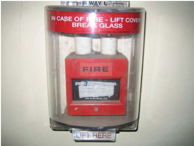
Figure 9.74 Proprietary device for protecting a manual fire alarm call point from accidental operation
