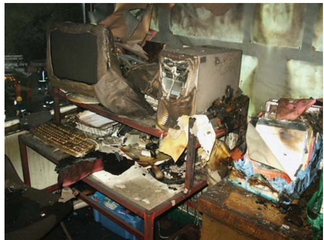
Figure 8.2 Electrical equipment involved in a school fire
