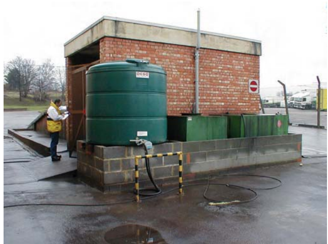
Figure 11.3 Fire safety hazards require active monitoring
