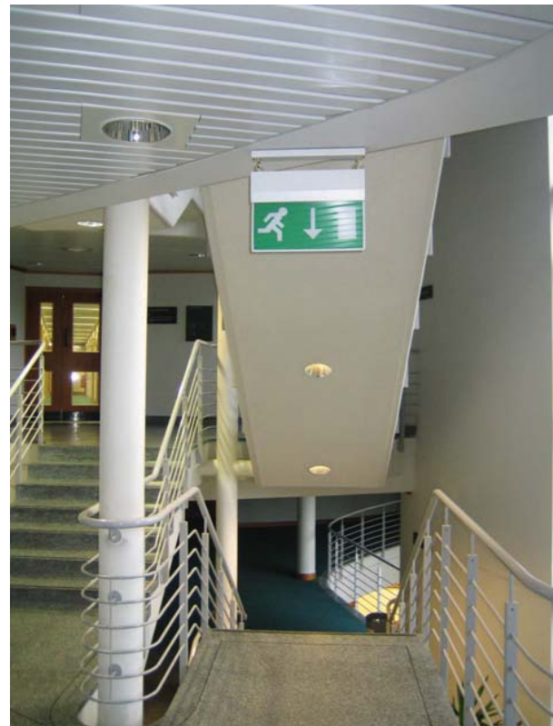
Figure 9.43 Typical modern escape stairway
