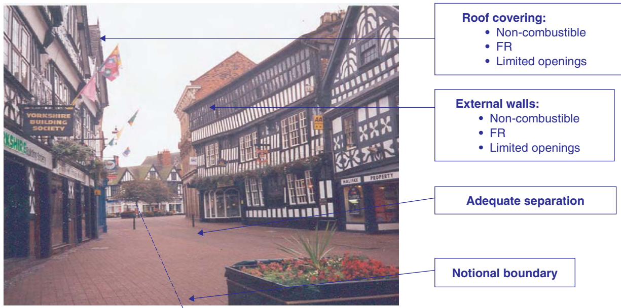
Figure 9.20 Preventing external fire spread
