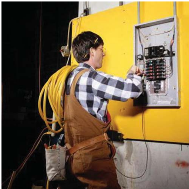
Figure 8.12 Electrical supply testing
