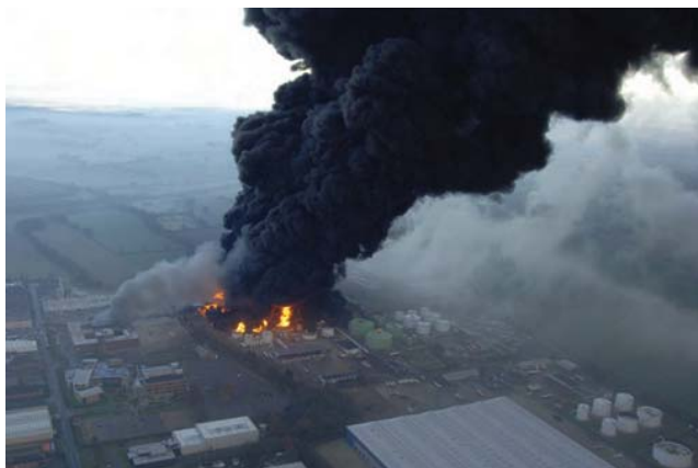
Figure 13.1 The environmental impact of fire
