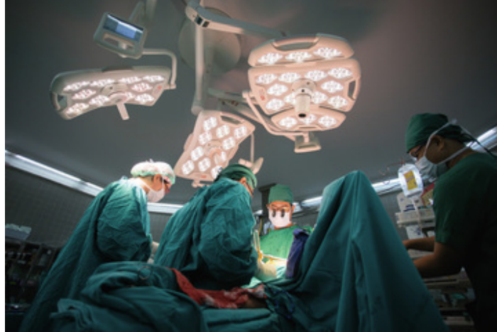
FIGURE 21-2 The lighting system in an operating room must provide a range of lighting intensity for a clear view of the surgical site. Source: surassawadee/ Shutterstock.com .
