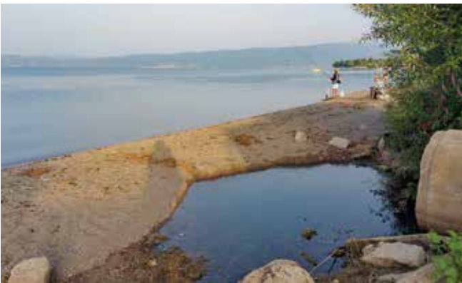
Fig. 11: The site of sewage overflows to Lake Ohrid at Voska in August 2022.
