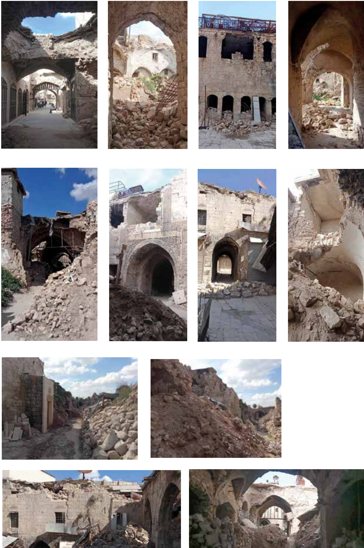
Fig. 40–51: Great destruction and collapse in the area of the old markets and caravanserais.
