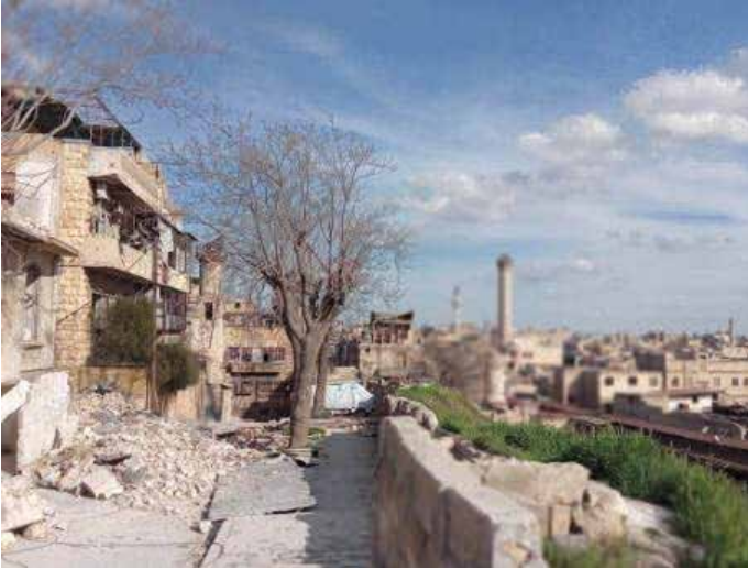
Fig. 10: A general view showing the demolition of the upper parts of many minarets.
