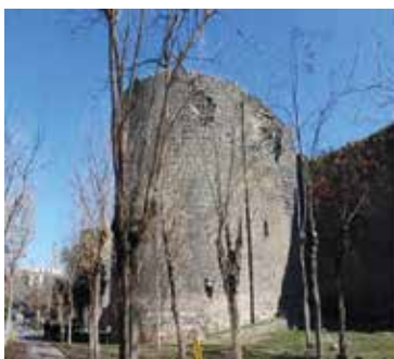
Fig. 42–44: 16th tower: On the surface, there are new collapses and swells. It bears risks in previously destroyed areas on the northern façade.
