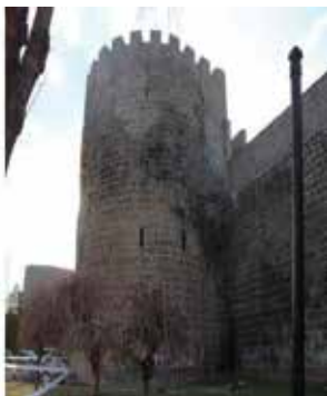
Fig. 47–50: 9th Tower: A large portion of the western façade collapsed. The destroyed area and its surroundings bear risks. There is also swelling on the northern façade and a high level of humidity.
