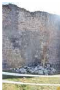
Fig. 30–34: 18th Tower: New stone falls have caused damage to the upper portion of the tower's south façade. Again, as a result of new stone falls caused by the earthquake, the damage in the previously ruined area in the upper part of the western façade grew. A small mass in the upper north façade above the previously devastated surface poses a danger.
