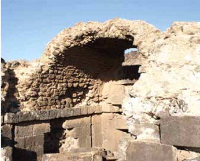
Fig. 6: Vault in Roman concrete and basaltic slag. Photo: T. F. Ifpo-MAFSS 2010
