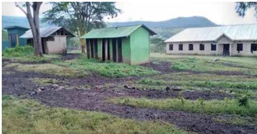
Fig. 4: The school compound in Endulen is deserted, and construction of the dormitory (on the right) has been stopped.
