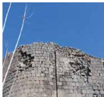
Fig. 45–46: 15th Tower: New stone collapses have occurred in previously fallen surfaces. The swellings on the tower's surface are at risk of demolishing it. The northern façade is saturated with humidity.
