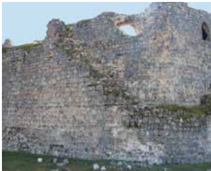
Fig. 5: Interior of the Wall between 49th and 48th Towers The surface stones of the fortification wall have fallen. There are partly swellings due to the earthquake on the wall as well as collapsed sections belonging to the pre-earthquake era. The wall between the 2nd buttress and the 47th tower has completely swelled, and the surface stones were poured in the upper part. The small openings at the bottom were closed during the restoration process. This wall needs an integrated, conservation-oriented conservation and restoration application.
