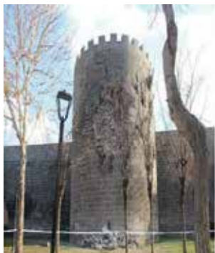
Fig. 47–50: 9th Tower: A large portion of the western façade collapsed. The destroyed area and its surroundings bear risks. There is also swelling on the northern façade and a high level of humidity.
