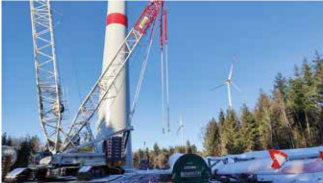
Fig. 1: Construction of wind turbines in Boppard-Weiler. Photo: Klaus Thomas
