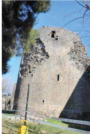
Fig. 45–46: 15th Tower: New stone collapses have occurred in previously fallen surfaces. The swellings on the tower's surface are at risk of demolishing it. The northern façade is saturated with humidity.
