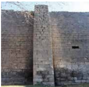
Fig. 13, 14: The Wall between 29th and 28th Towers: It was observed that there were new stone spills in the previously destroyed areas with the earthquake.
