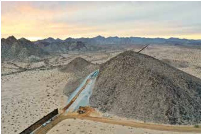
Fig. 1: New border wall built in El Pinacate. Photo: Russ McSpadden / Center for Biological Diversity
