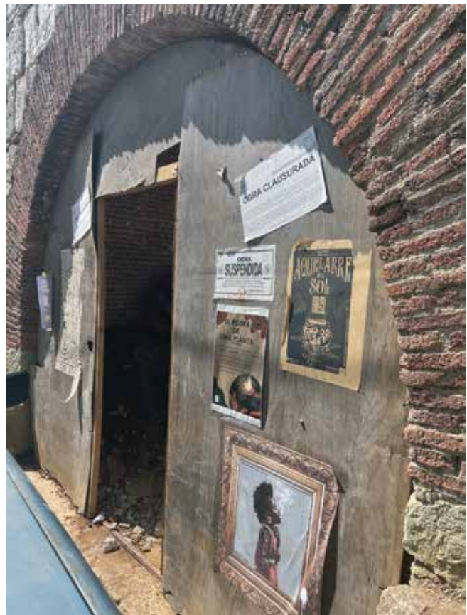
Fig. 3: Works continue despite foreclosure seals.
