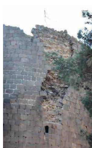
Fig. 38–41: 17th Tower: The shedding of surface stones on the southwest and northwest façades of the tower has resulted in demolition and weathering. It's perilous.
