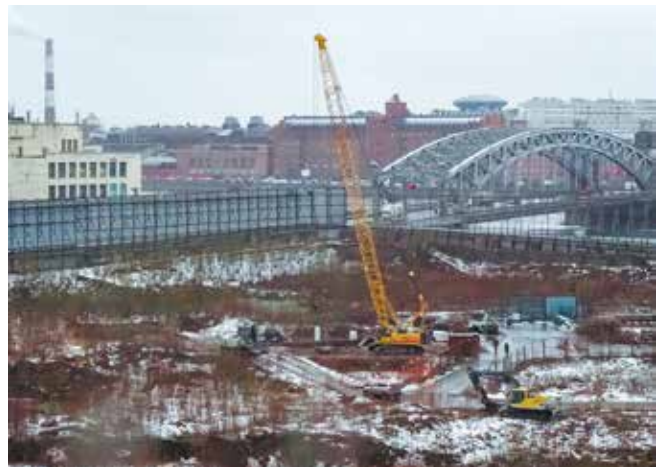
Fig. 5: Ongoing construction with heavy equipment on Okhta Cape, January 2023.
