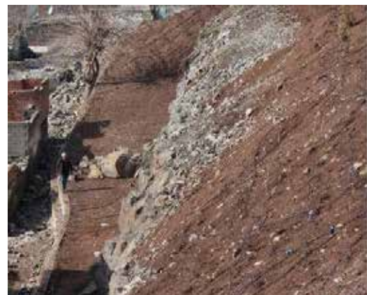
Fig. 9, 10: Rocky Area below Tower 36 and 35: It was observed that large pieces of rock fell from the rock layer at the base of towers 36-35.
