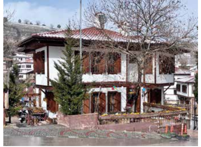
Fig. 4: Reinforced concrete replica hotel in Çukur, Safranbolu. Carelessness reveals itself by the fact that the protruding buttresses are too thin to be a carrier. Photo: İbrahim Canbulat
