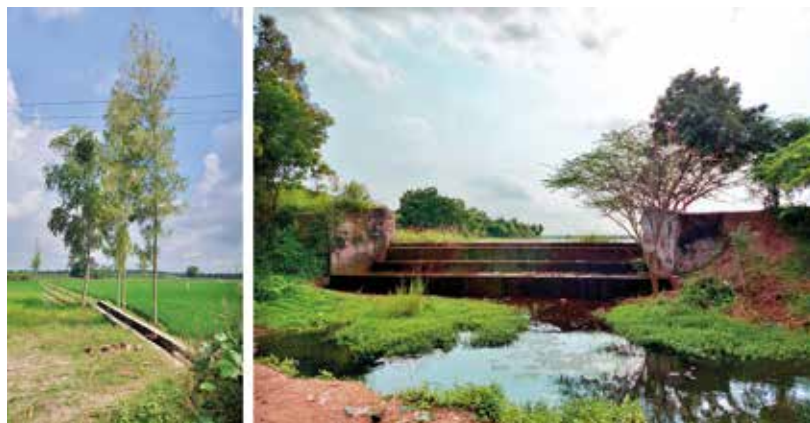
Fig. 6: (Left) Irrigation channel that supplies water to the agricultural fields; (Right) Surplus weir that allows excess water from an eri to reach the next one in a series. Photos: Aghash Natarajan
