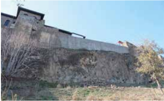
Fig. 55, 56: Rock Layer under the Eastern Walls of the inner citadel: The earthquake destroyed the rock layer beneath the Museum Excavation Exhibition Building. The same rocky surface has numerous cracks.
