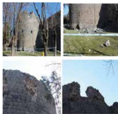
Fig. 30–34: 18th Tower: New stone falls have caused damage to the upper portion of the tower's south façade. Again, as a result of new stone falls caused by the earthquake, the damage in the previously ruined area in the upper part of the western façade grew. A small mass in the upper north façade above the previously devastated surface poses a danger.
