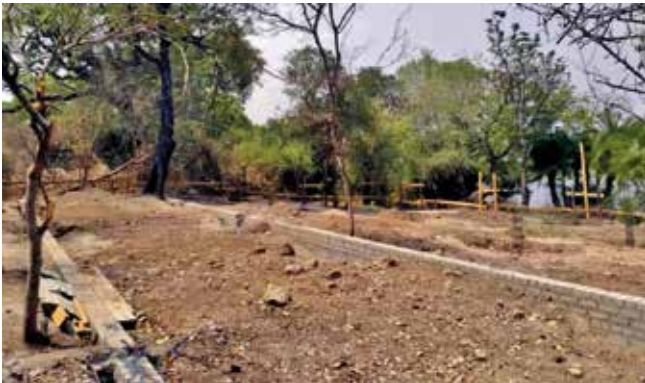
Fig. 1: Riverside Restaurant construction
