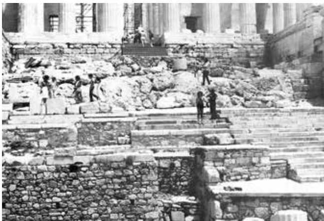
Fig. 7: View of the west access of the Acropolis from the west, about 1980. The restored steps from the 1850s are missing, because they were considered too intrusive. They have been replaced by a zig-zag ramp in a lower level, following the plan restored by Gorham P. Stevens (see below, fig. 8), which most probably was in use for centuries, after the erection of the Propylaia. Photo: Tasos Tanoulas
