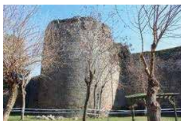
Fig. 38–41: 17th Tower: The shedding of surface stones on the southwest and northwest façades of the tower has resulted in demolition and weathering. It's perilous.
