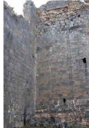
Fig. 45–46: 15th Tower: New stone collapses have occurred in previously fallen surfaces. The swellings on the tower's surface are at risk of demolishing it. The northern façade is saturated with humidity.
