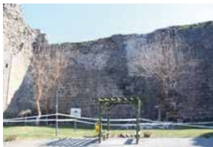
Fig. 30–34: 18th Tower: New stone falls have caused damage to the upper portion of the tower's south façade. Again, as a result of new stone falls caused by the earthquake, the damage in the previously ruined area in the upper part of the western façade grew. A small mass in the upper north façade above the previously devastated surface poses a danger.
