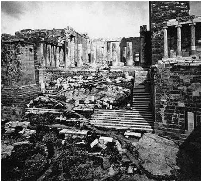
Fig. 6: View of the west access of the Acropolis from the west, after clearing of medieval and Turkish structures. Few of the Roman steps survive in situ. Next to the left wall of the Athena Nike bastion, a narrow flight of steps was reconstructed in the 1850s, after the model of the Roman steps, for providing visitors' access to the Propylaia. Photo: Stillman, 1869
