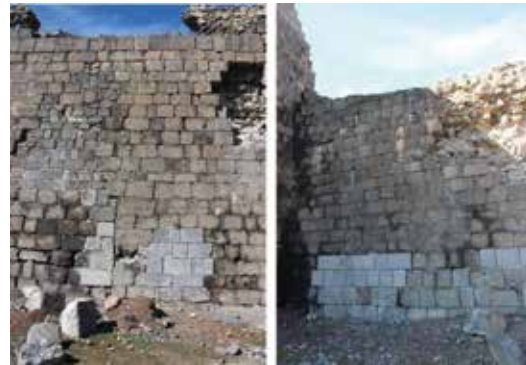
Fig. 5: Interior of the Wall between 49th and 48th Towers The surface stones of the fortification wall have fallen. There are partly swellings due to the earthquake on the wall as well as collapsed sections belonging to the pre-earthquake era. The wall between the 2nd buttress and the 47th tower has completely swelled, and the surface stones were poured in the upper part. The small openings at the bottom were closed during the restoration process. This wall needs an integrated, conservation-oriented conservation and restoration application.
