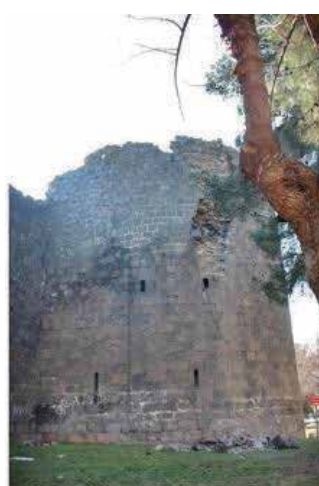
Fig. 38–41: 17th Tower: The shedding of surface stones on the southwest and northwest façades of the tower has resulted in demolition and weathering. It's perilous.
