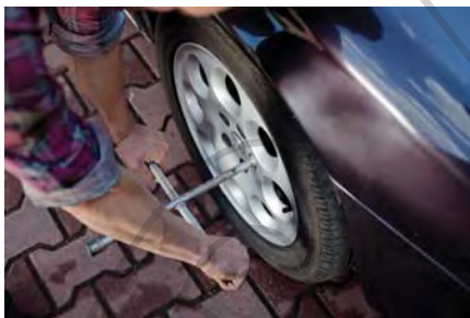
▲ Figure 5.23 A long spanner is used to undo the nuts on the wheel of a car.
