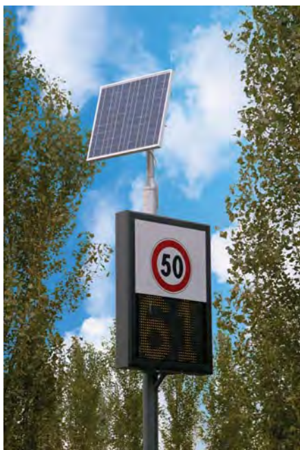
▲ Figure 1.33 This traffic slowing sign is powered by solar cells.
