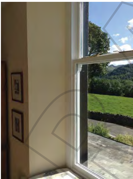
▲ Figure 1.17 This house was built in 1820. The walls are 70 cm thick. This keeps the house warm.
