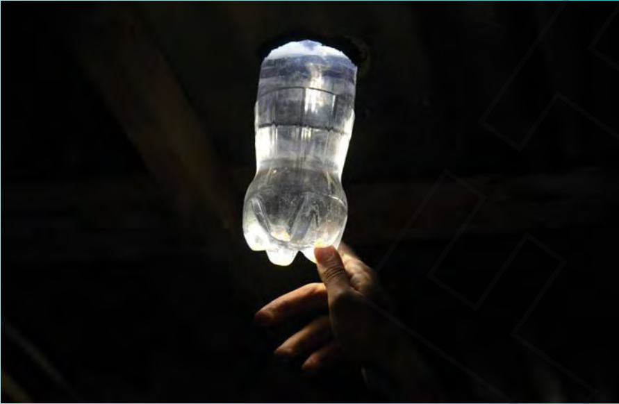
▲ Figure 7.63 A plastic bottle filled with water provides about the same amount of light as a 50W bulb.
