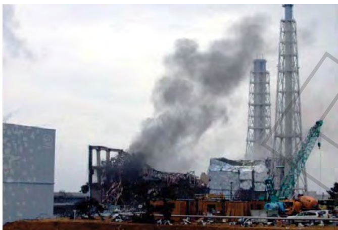
▲ Figure 4.19 The Fukushima Daiichi power plant in Japan
