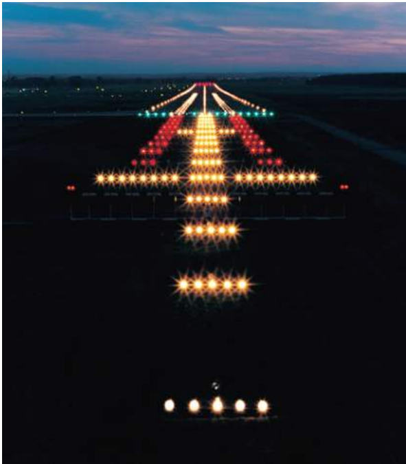
ALSF-2 Airport Rechnology.com/ Binrock.net / USAF/FAA photo
