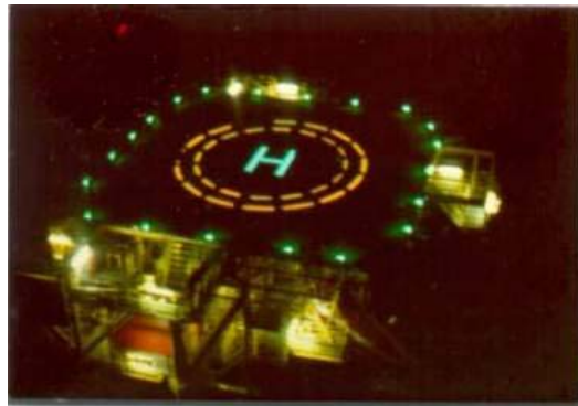
Lighting - Preferred Trial Equipment Configuration
