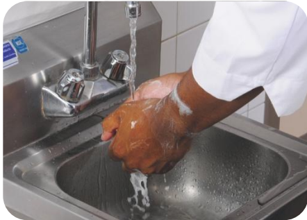
Hot and cold running water
