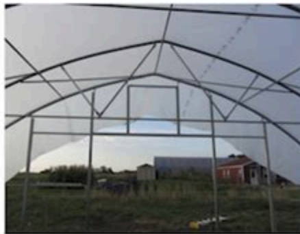
End Wall Framing
