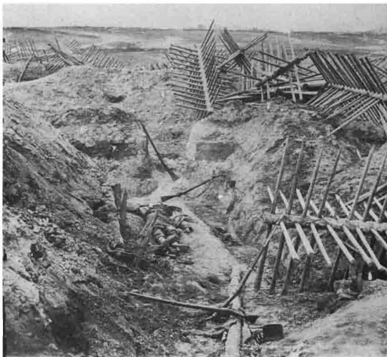
Confederate trenches at Petersburg, with chevaux-de-frise (pointed stakes) and dead soldier, after the successful Union assault on April 2, 1865
